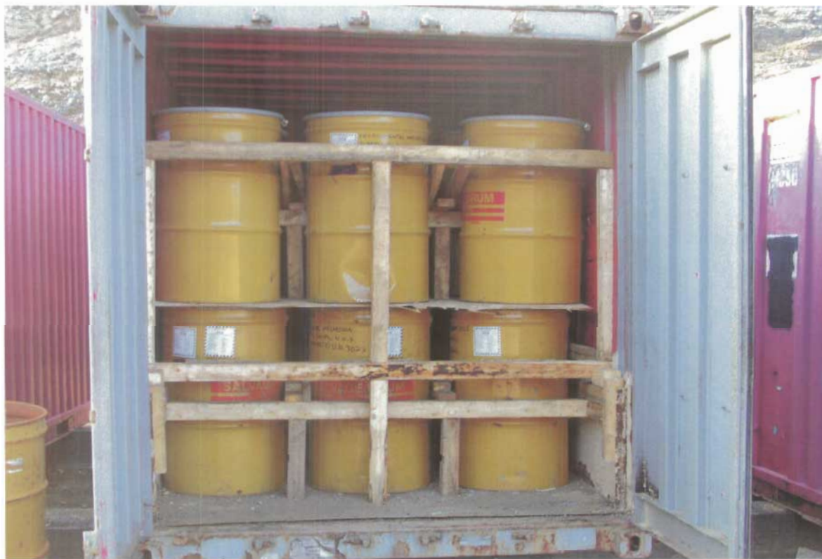
Photograph IV-2: Yellow Overpack Drums Containing Blue Plastic Barrels of PCB Contaminated Concrete Placed Inside a SeaCan Ready for Off-Site Disposal
