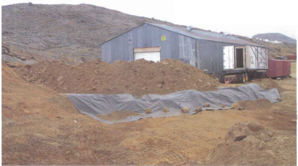
Photograph IV-3: The CEPA Soil Stockpile From the Excavation at the S1/S4 Beach Area The Soil Was Subsequently Screened and Transferred to Conical Steel Containers
