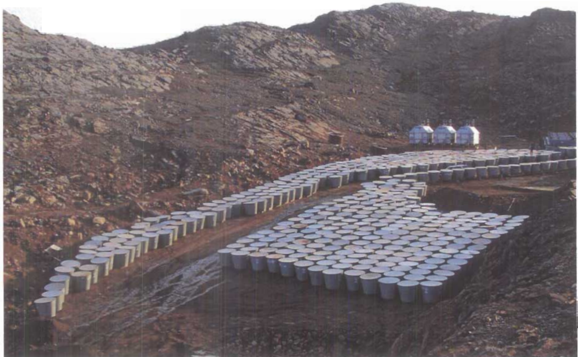
Photograph IV-4: Some of the 516 Conical Steel Containers Filled With CEPA Soil Awaiting the Ship to Transport Them to Quebec For PCB Destruction
