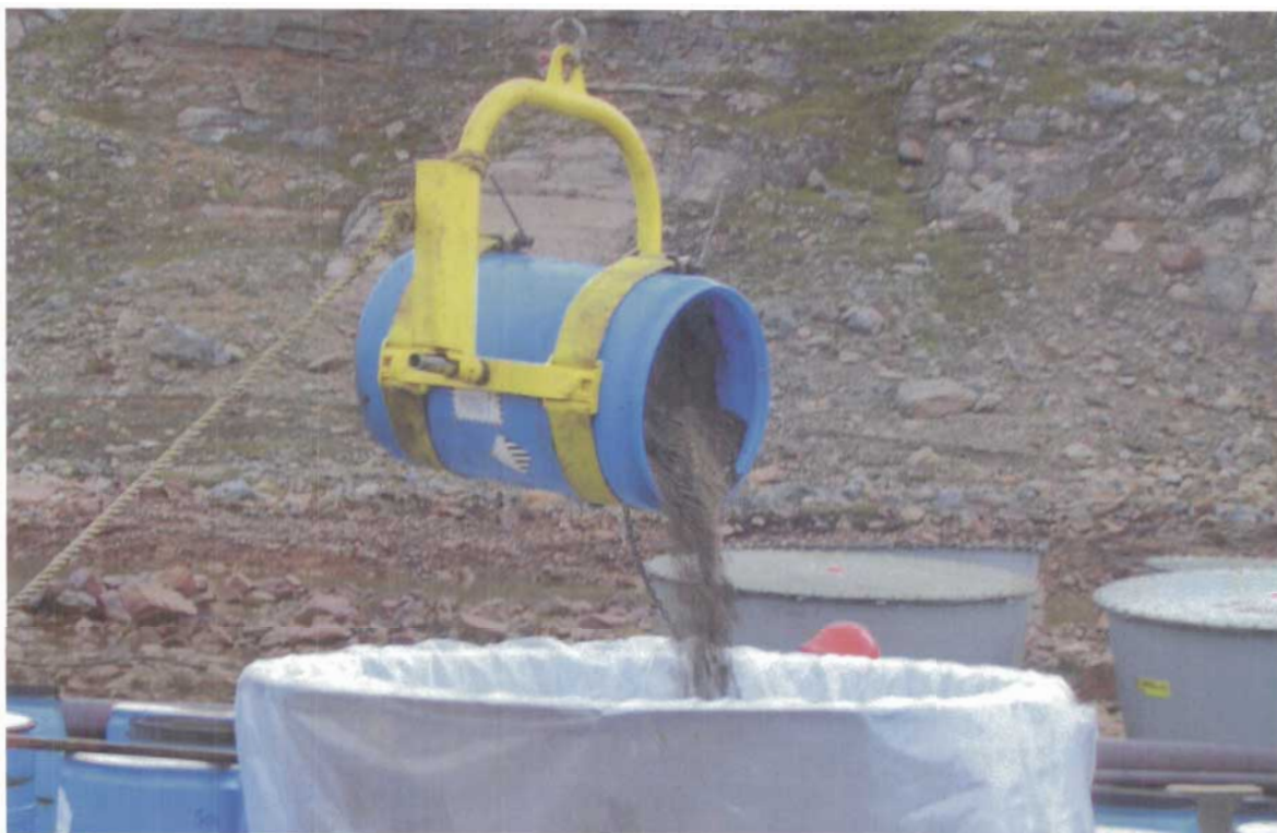
Photograph IV-1: Transferring CEPA Soil From a 205 Liter Plastic Barrel to a 3.1 Cubic Meter Conical Steel Container for Off-site Shipment
