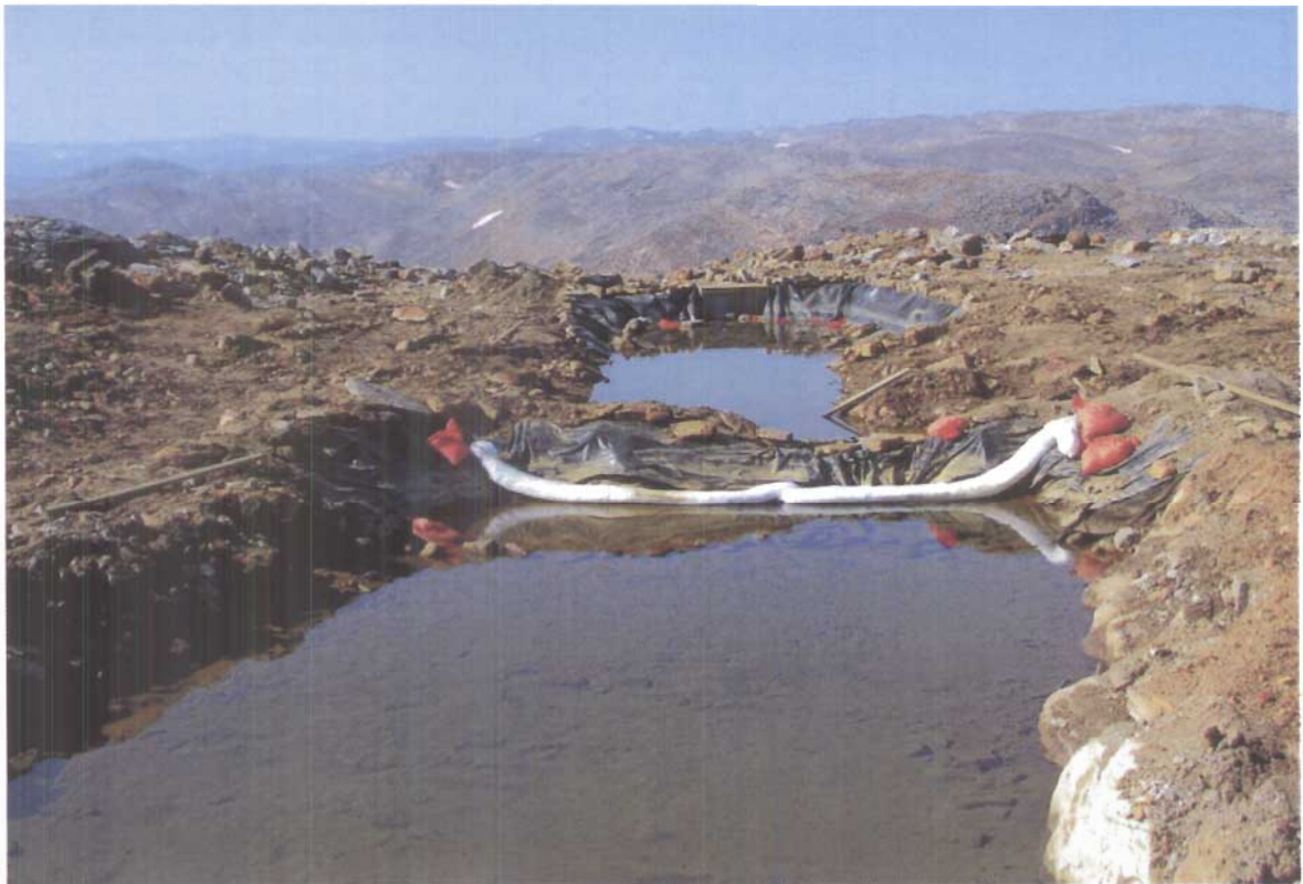
Photograph V-8: The Completed Trial Remediation System Showing the Pond With Boom in the Foreground and Barrier Filter Box Beyond and Down Stream
