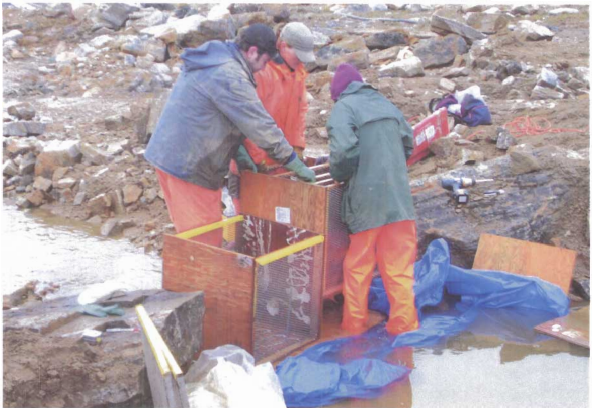
Photograph V-5: Installing the Filter Boxes in the Barrier
