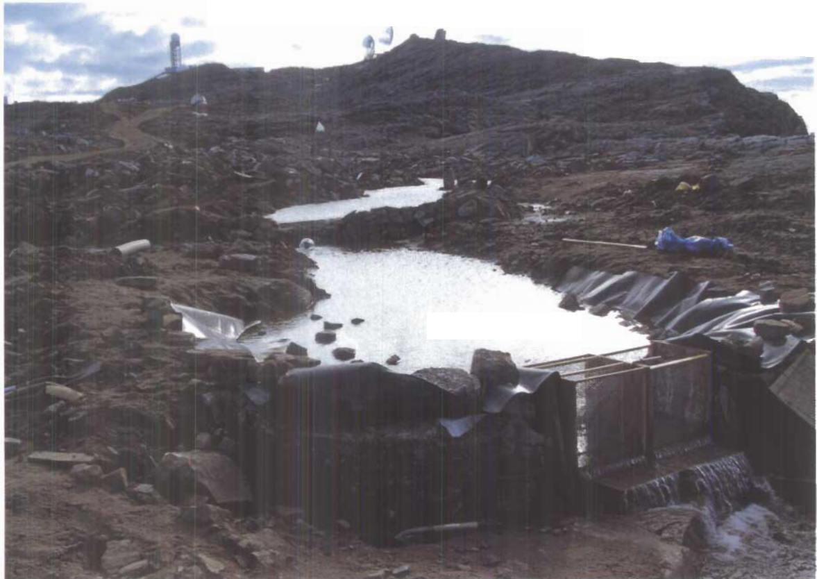
Photograph V-6: The Barrier in Position but Without Filters: The Pond is Shown in the Background
