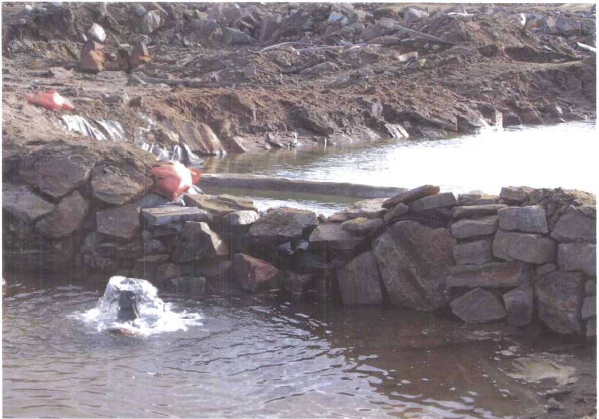
Photograph V-7: The Division Between the Pond, Which is Draining into a Second Pond Created by the Barrier, with Filters in Place
