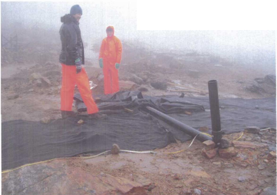
Photograph V-4: Constructing the Pond: The ABS Pipe Allows Water to be Siphoned Off From the Base of the Pond and Also Controls the Water Level in the Pond
