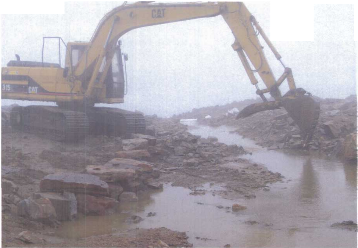
Photograph V-3: Excavating the Drainage Channel For the Pond and Barrier
