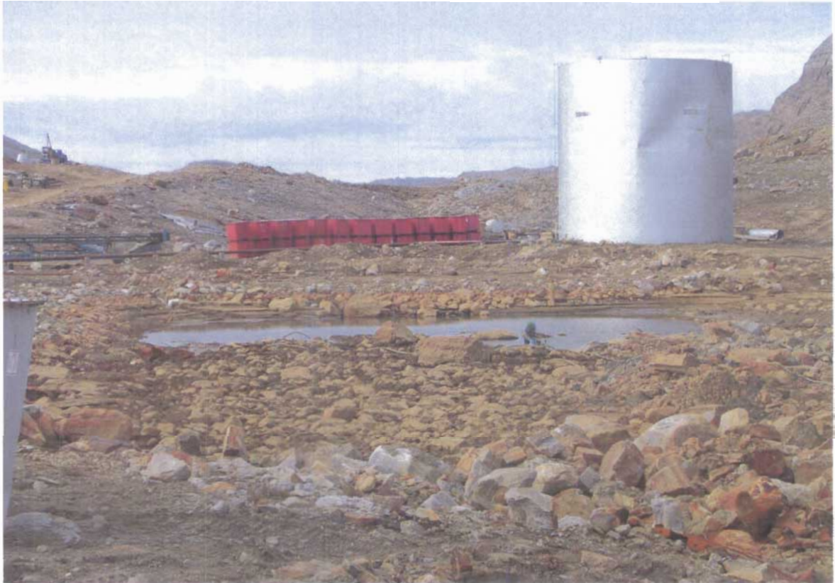
Photograph V-9: The Pond Between the Two POL Tanks After Draining: The Original Boundary of the Pond is Outlined by the Brown Staining
