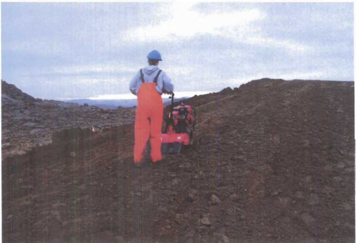
Photograph V-14: Rototilling the Main Landfarm
