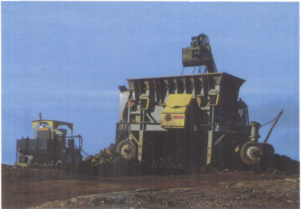
Photograph V-13: The Hydrocarbon Contaminated Soil Was Screened Prior to the Construction of the Main Landfarm
