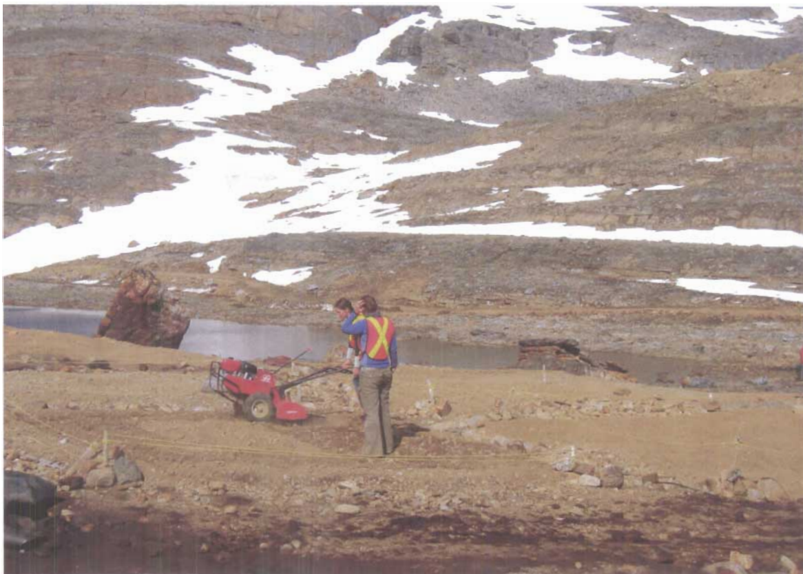
Photograph V-11: Rototilling the Trial Landfarm Plots
