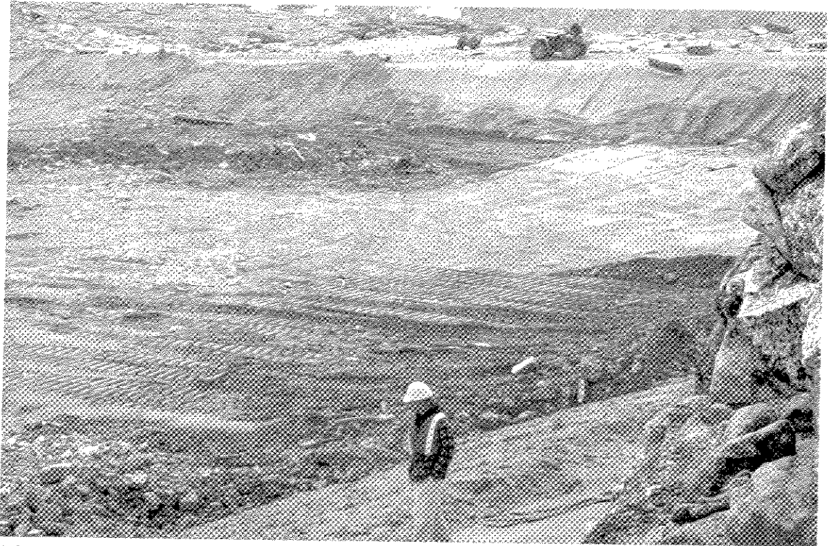
Photograph III-3: Contaminated Soil was Added to the Landfill in Lifts and Compacted
