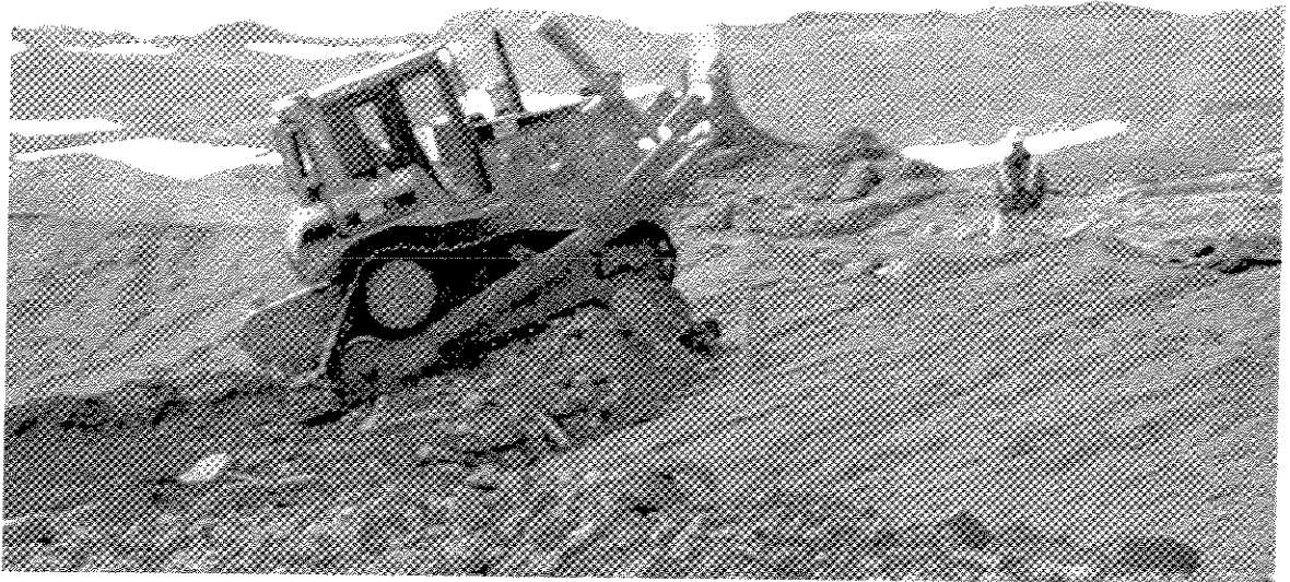
Photograph III-1: Soil was Transported From the Various Tier II Contaminated Areas and Placed Within the Lined Area of the Tier II Landfill
