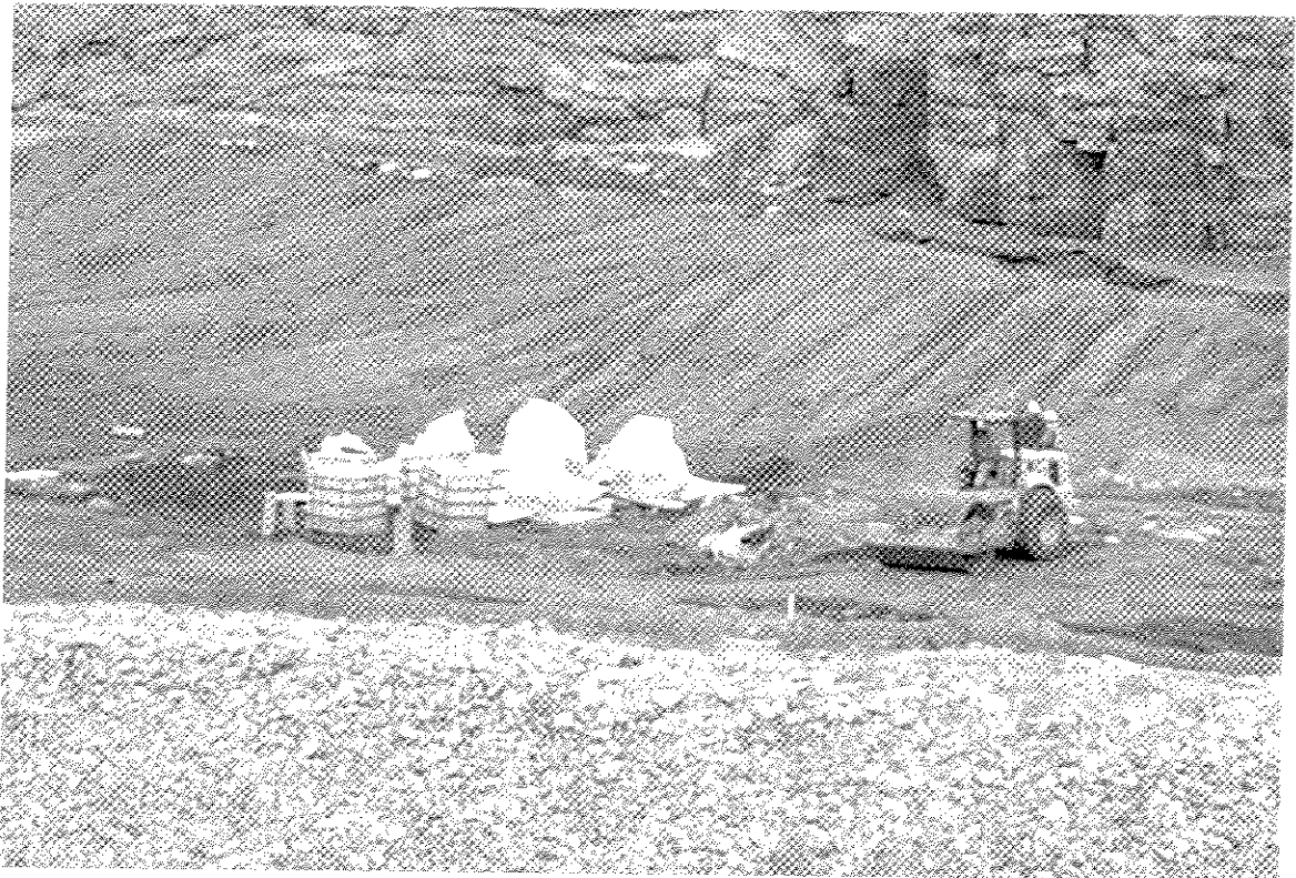
Photograph III-2: Soil Was Placed in Lifts in the Landfill and Compacted: Metal Contaminated Soils Previously Stored in Wooden Boxes Were Placed in the Landfill
