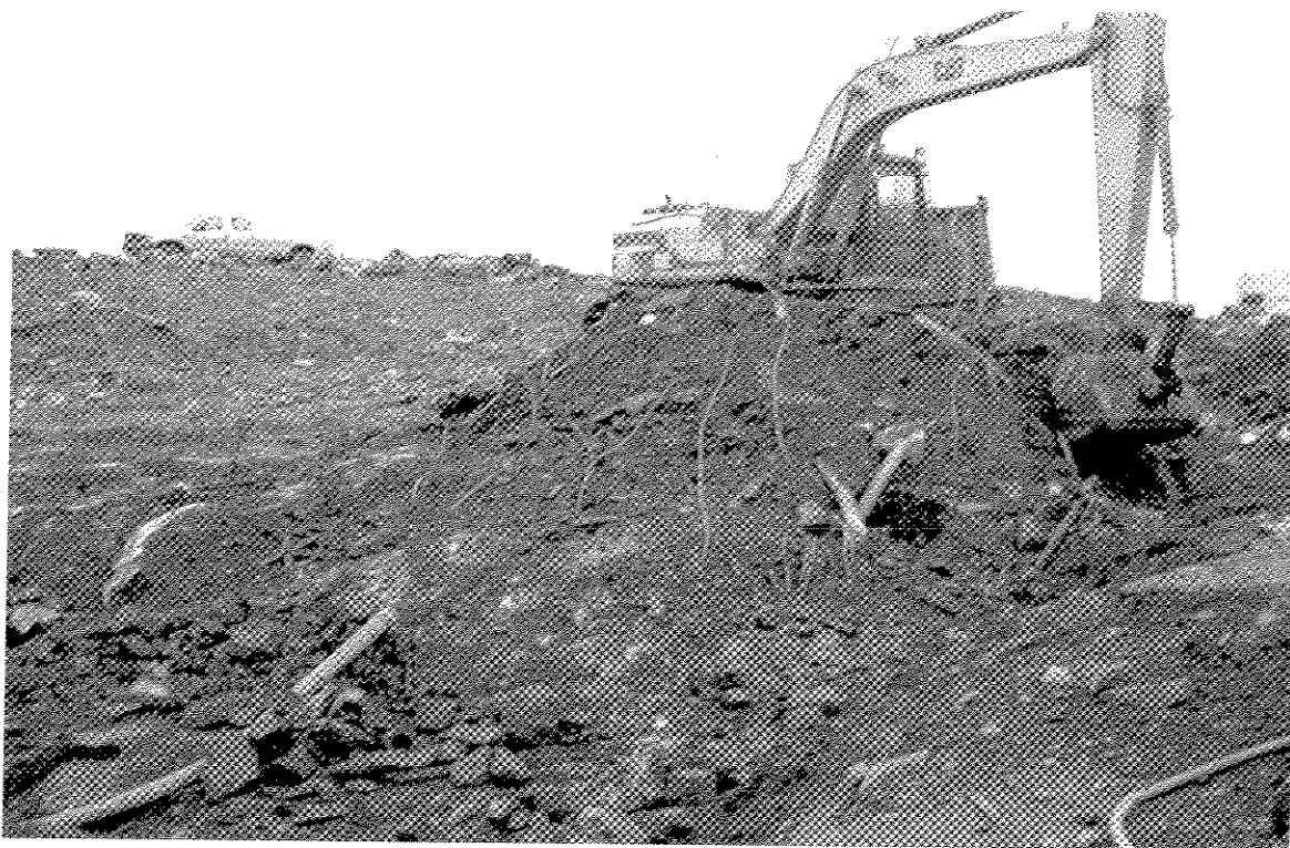
Photograph II-21: Excavating Metal Contaminated Soils at the Beach Dump
