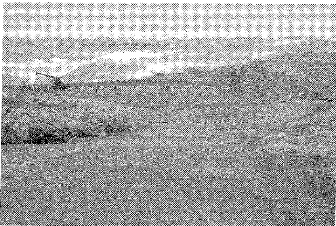
Photograph III-5: The Top Liner Was Added When All Contaminated Soil Was in Place
