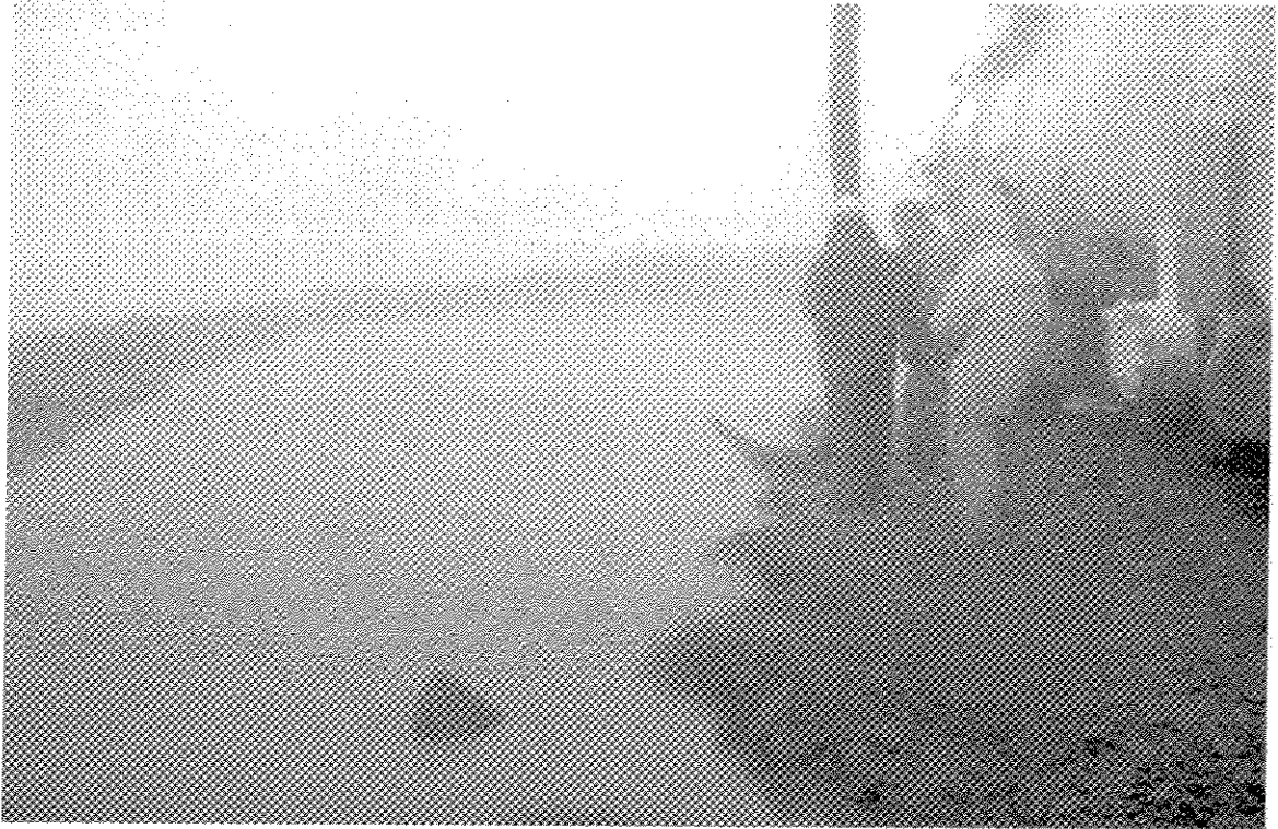
Photograph III-7: Torrential Rains Caused Flooding of the Landfill During Construction: The Water was Pumped Out and Discharged Through the PCB Barrier
