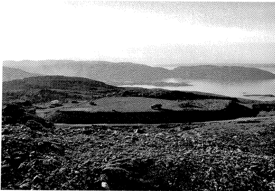
Photograph III-6: Finally a Cap of Clean Gravel Was Added to Ensure Freeze Back of All the Contaminated Material Within the landfill
