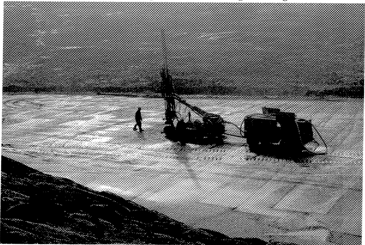
Photograph III-8: Thermister Strings Were Installed as Part of the Long Term Monitoring Program
