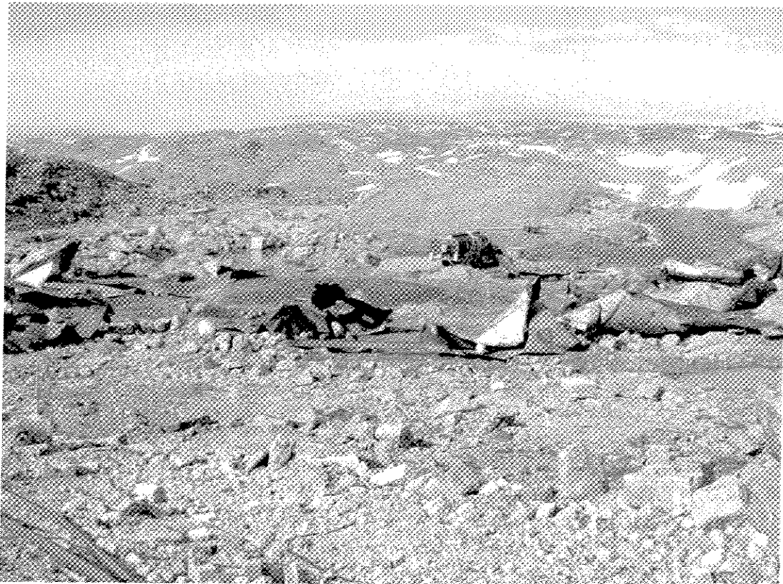
Photograph V-1: The Remains of the Imploded Tank After its Demolition: Note the Hydrocarbon Contaminated Pad and the Main Landfarm Beyond
