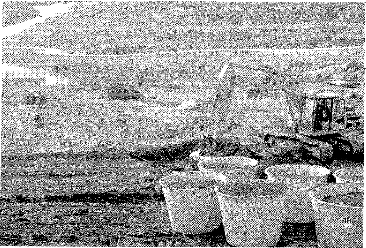
Photograph V-11: Excavating Plots For the In Situ Landfarm Experiment
