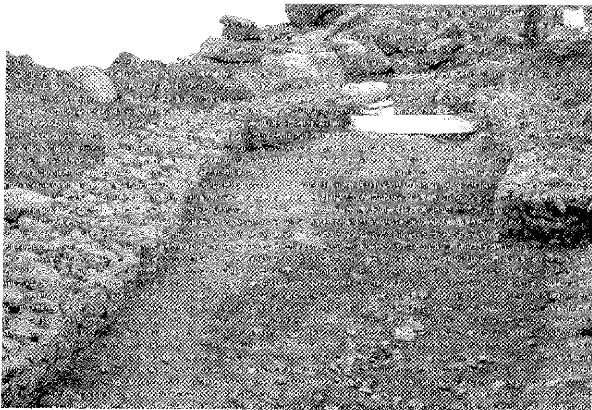
Photograph VI-9: Gabion Walls Were Constructed to Form the Channel Through Which Water From the S1/S4 Beach Area Then Was Forced to Flow
