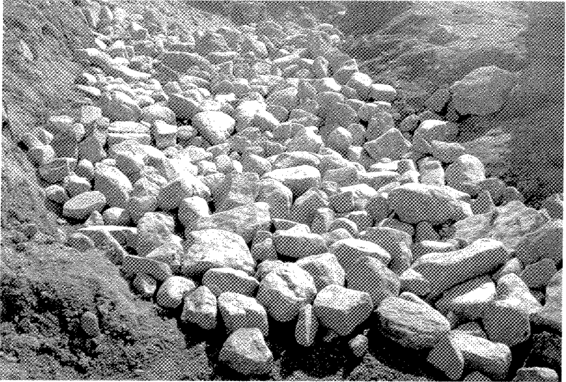
Photograph VI-13: The Channel Above the Top Gabion Sediment Trap Was Lined With Cobbles To Trap More Sediment
