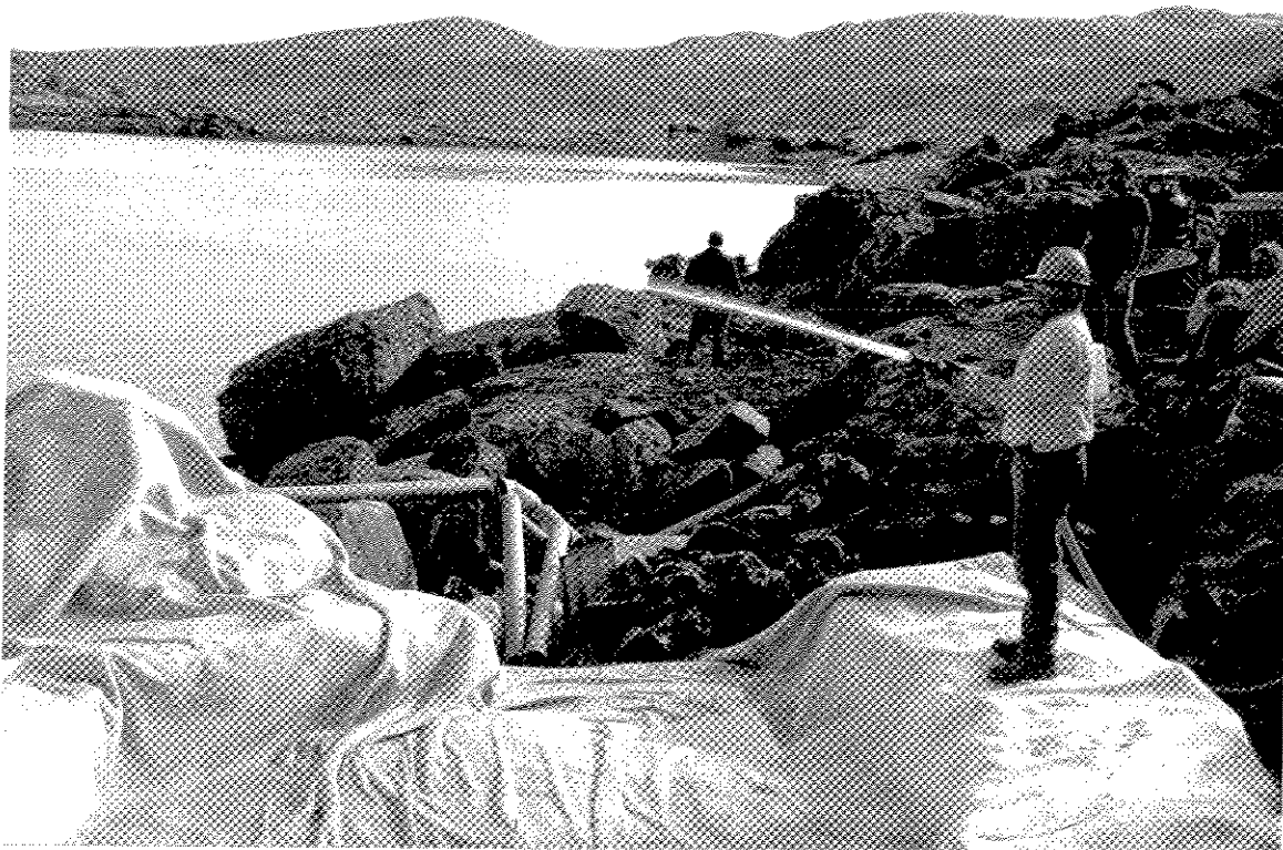
Photograph VI-10: After the Geocomposite Clay Liner was Placed in Position, It was Wetted to Form a Sealed Channel
