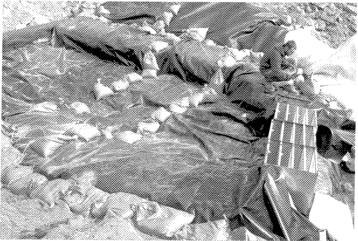
Photograph VI-11: A Black Liner Was Then Placed on Top of the GCL and Sealed Around the Filter Box. Sandbags Secured the Liner to the Contoured Channel
