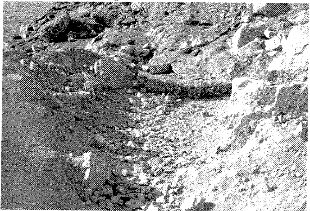
Photograph VI-12: Gabions Were Placed Across the Drainage Channel Above the Steep Slope Leading to the Barrier as an Additional Sediment Trap
