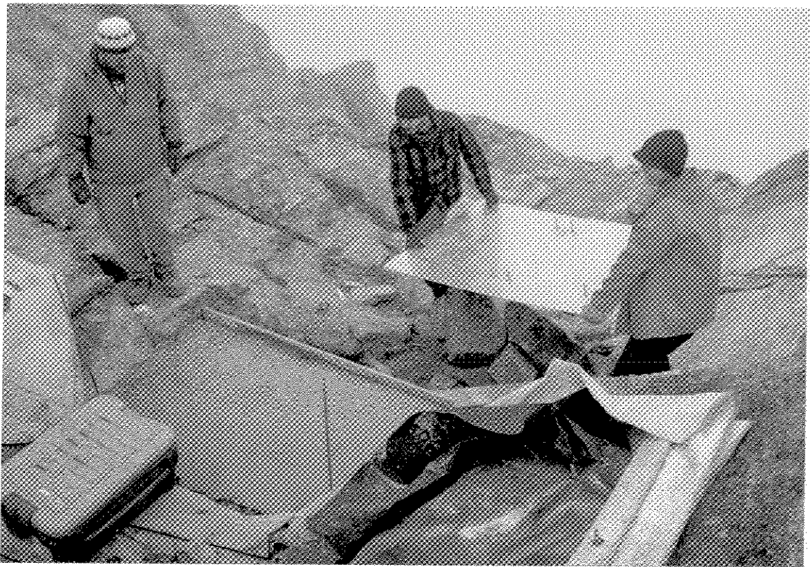
Photograph VI-15: After Removing the Wooden Filter Box, a Concrete Base was Poured and Rock Bolts were Positioned To Secure the Stainless Steel Base Plate in Place
