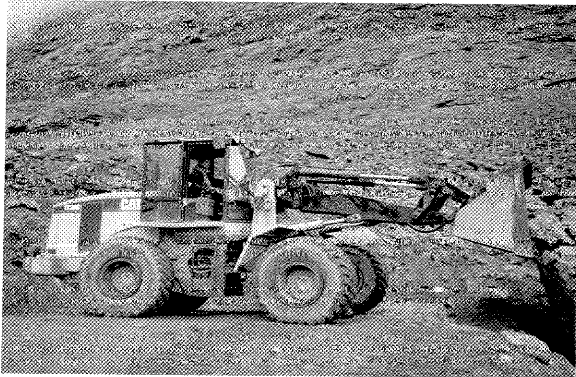
Photograph II-4: Heavy Equipment Working at the S1/S4 Beach Area
