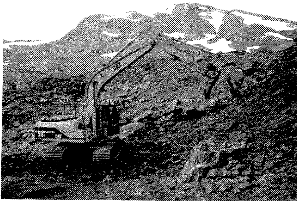
Photograph II-6: Excavating Tier II Soils From a Platform Close to the Cliff
