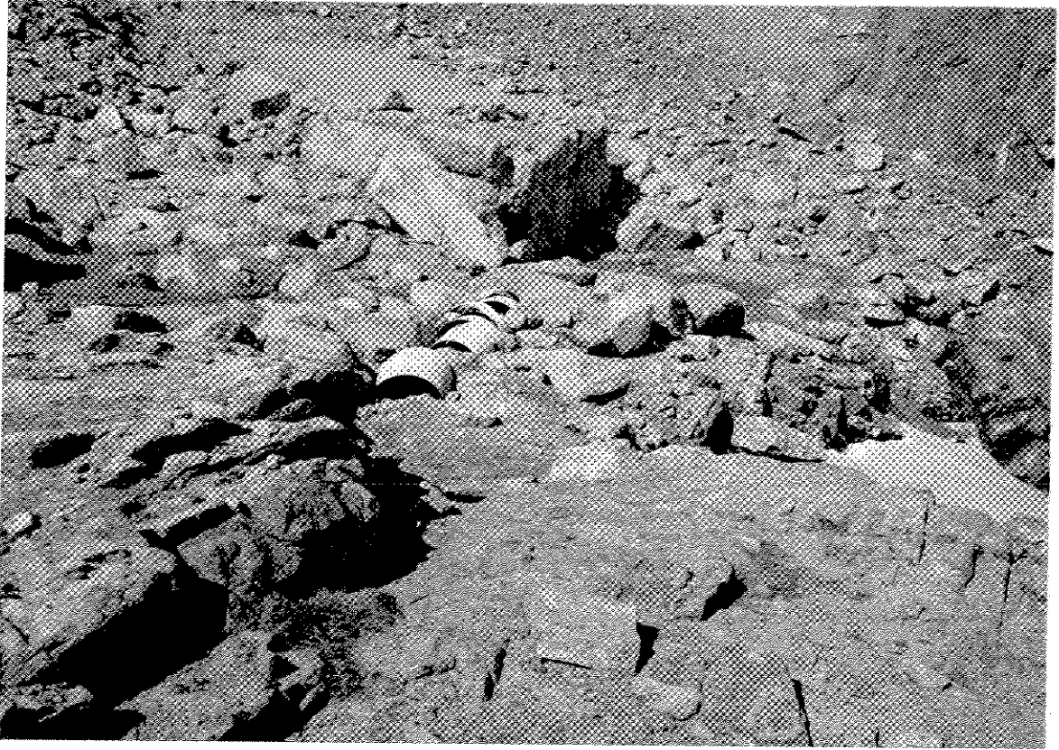
Photograph II-1: The 1994 Barrier Still in Place at the Start of the Season
