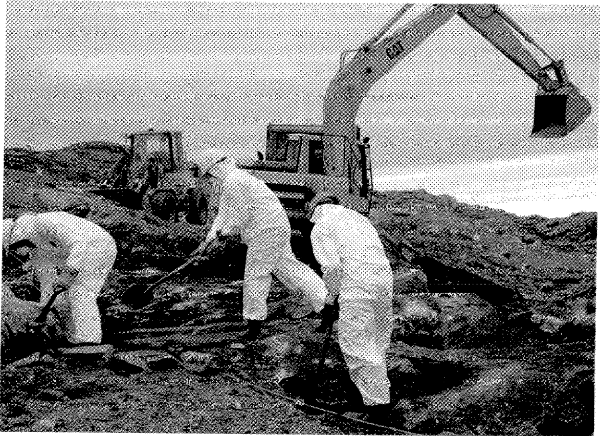
Photograph II-9: Removing the Last of the CEPA Soil by Hand From a Pocket of High Contamination Found Below Dish B
