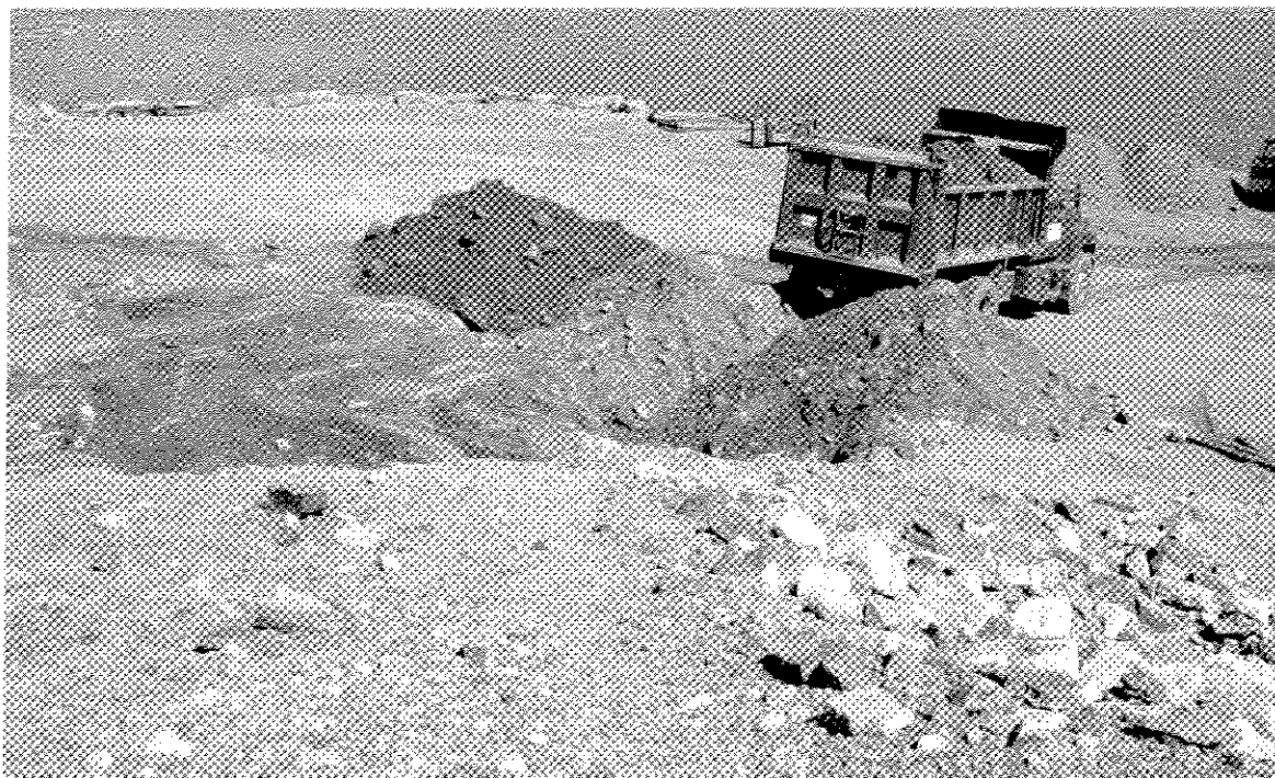
Photograph II-19: Excavating the PCB Contaminated Soil at the DND Helipad Site
