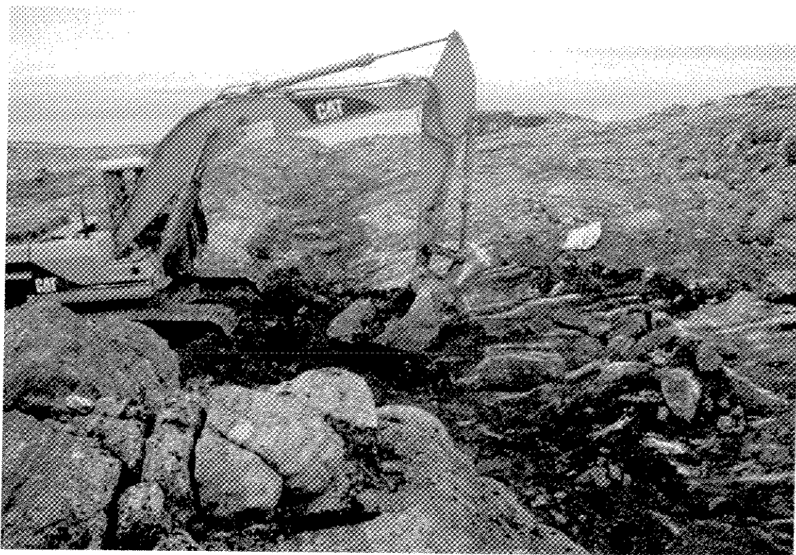
Photograph II-16: Excavating the Debris From the PCL Dump
