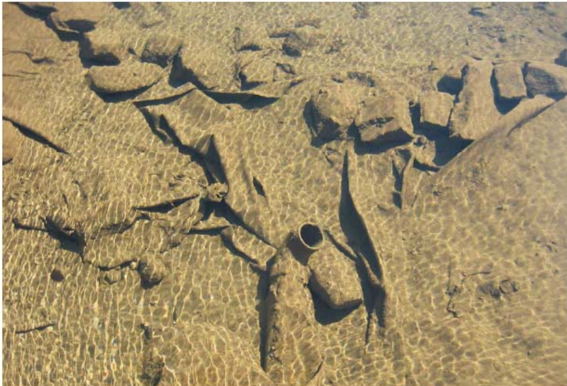
Photograph 13: The PVC Pond Liner Was Intact Below the Water Line Where it Was Covered With a Layer of Sediment
