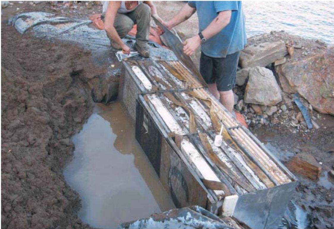
Photograph 16: Replacing the Lids on the Filter Box After Recharging the Filters With Fresh Materials
