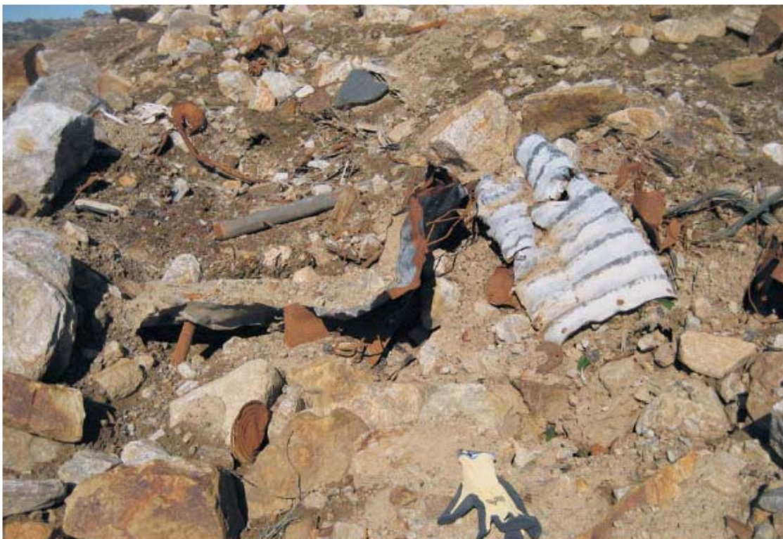
Photograph 6: Some Visible Debris at the Steep Edge of the Airstrip Dump was Not Covered During the Remediation Program
