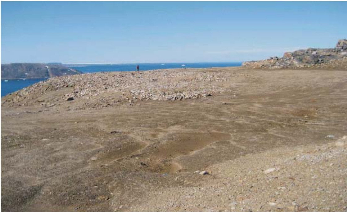
Photograph 5: The Airstrip Landfill Showing the Surface in Good Condition with Minimal Erosion Pathways
