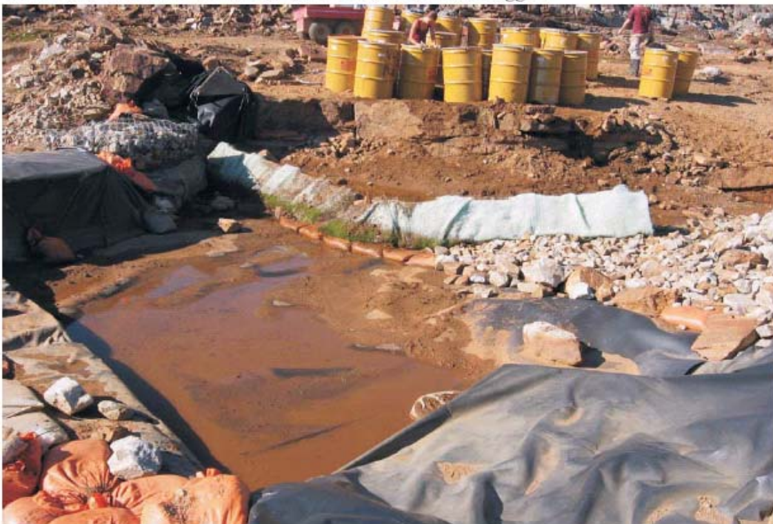
Photograph 15: The Valley Barrier After the Sediment Was Shoveled Out Into Thirteen Overpack Drums:
