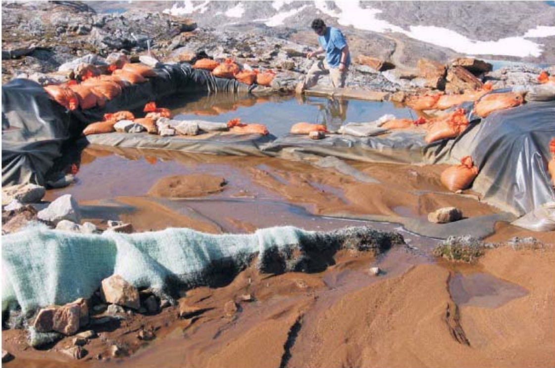
Photograph 14: The Valley Barrier at the Start of the Site Visit; Much More Sediment Was Present Than Last Year and the Filter Box was Clogged
