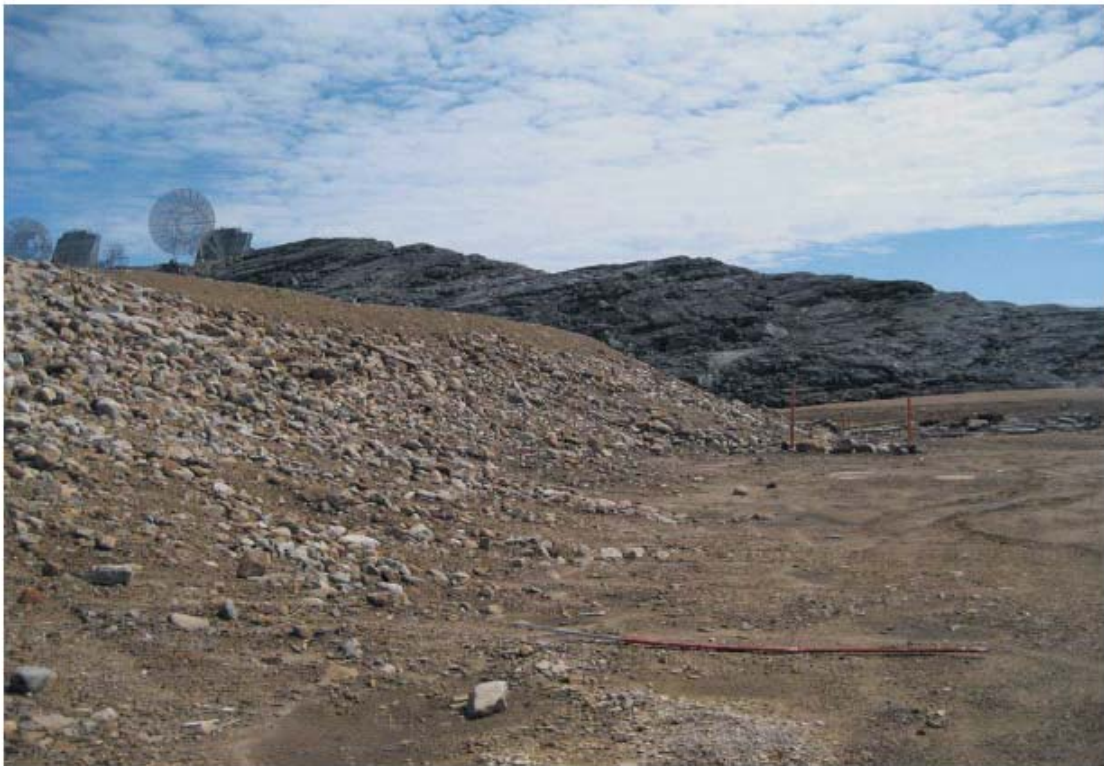
Photograph 2: View of the South Berm Showing Areas of Erosion and Ponded Water
