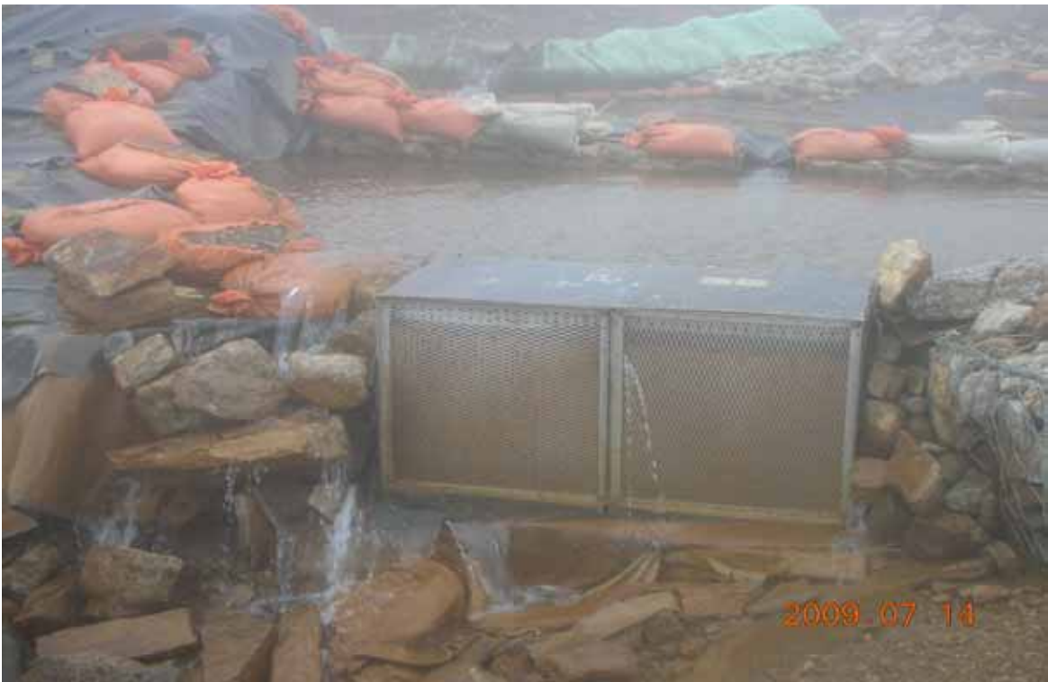
Photograph 21: The S1/S4 Valley Barrier on 14 July Overflowing Due to Snow Melt
