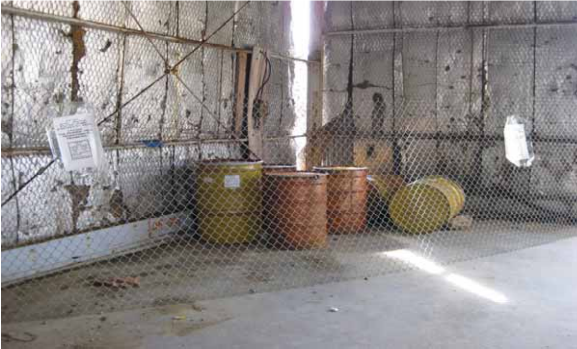
Photograph 18: The PCB Storage Facility Nearing its Completion Within Building B2: Only the Four Drums Containing CEPA Soil Were Left in the Building on its Completion
