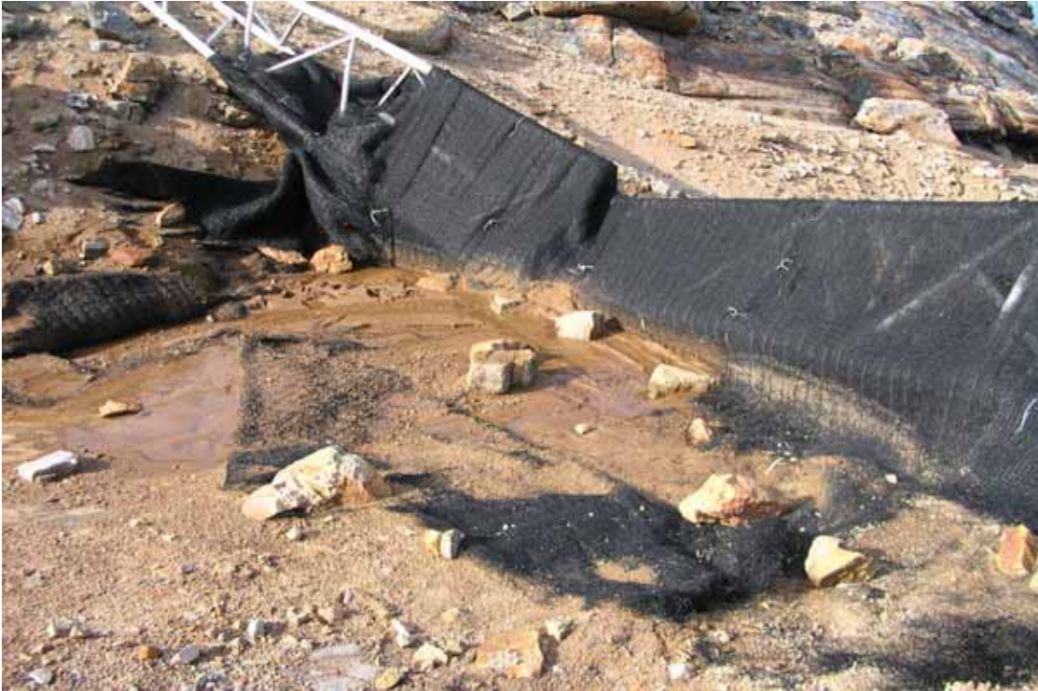
Photograph 26: Sediment Collected Above the Silt Fence at the Furniture Dump
