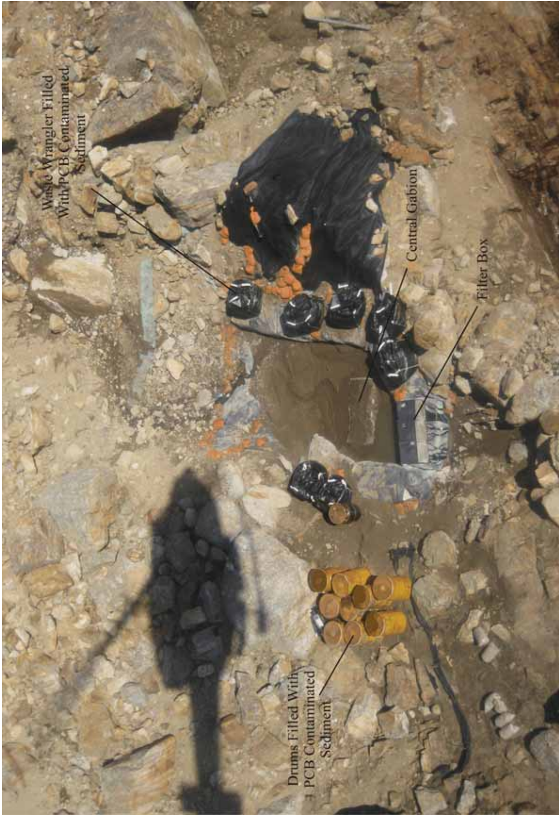
Photograph 23: The S1/S4 Beach Barrier From the Helicopter Showing Drums and Waste Wranglers Filled in 2007 and 2008 With PCB Contaminated Sediment
