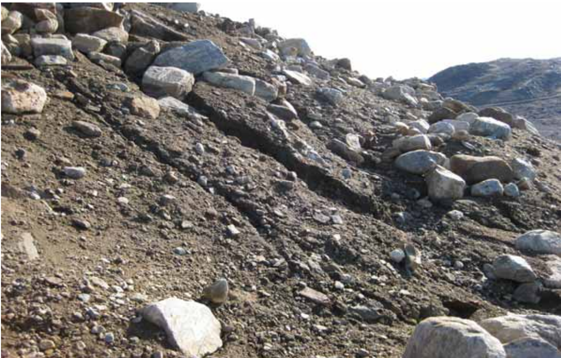
Photograph 12: Erosion Channels Have Developed in Some Areas of the Toe of the Airstrip Landfill
