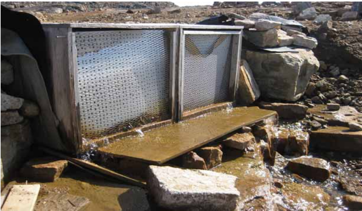
Photograph 17: Water Was Flowing Freely From the Base of the Filter Box
