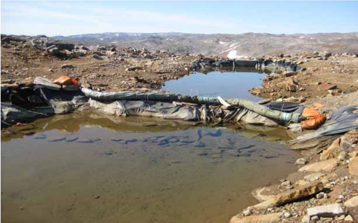
Photograph 16: The Ponding and Barrier System Put in Place to Remove Hydrocarbons From the Drainage Channel Leading From the Camp and Main Landfarm was in Excellent Condition
