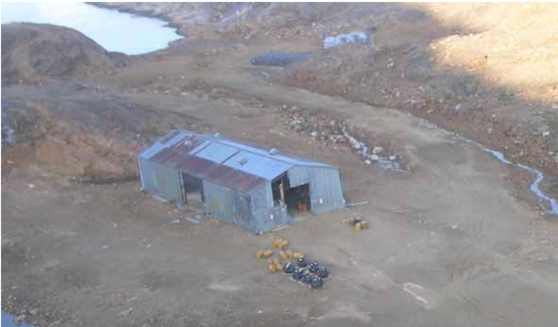
Photograph 19: Waste Wrangler Containers on Pallets and Overpack Drums Filled in 2007 and 2008 With PCB Contaminated Soil from the Barriers. This Photograph Was Taken When 15 of the 34 Drums Had Been Moved to the Area. Building B2 Lost an Additional Panel of Cladding by the Door Over the Past Winter
