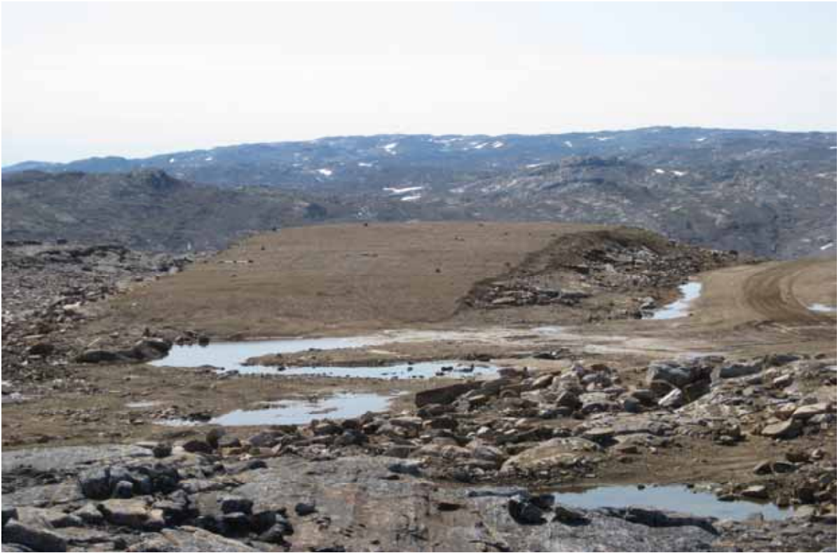
Photograph 15: The Main Hydrocarbon Landfarm Showed No Signs of Erosion
