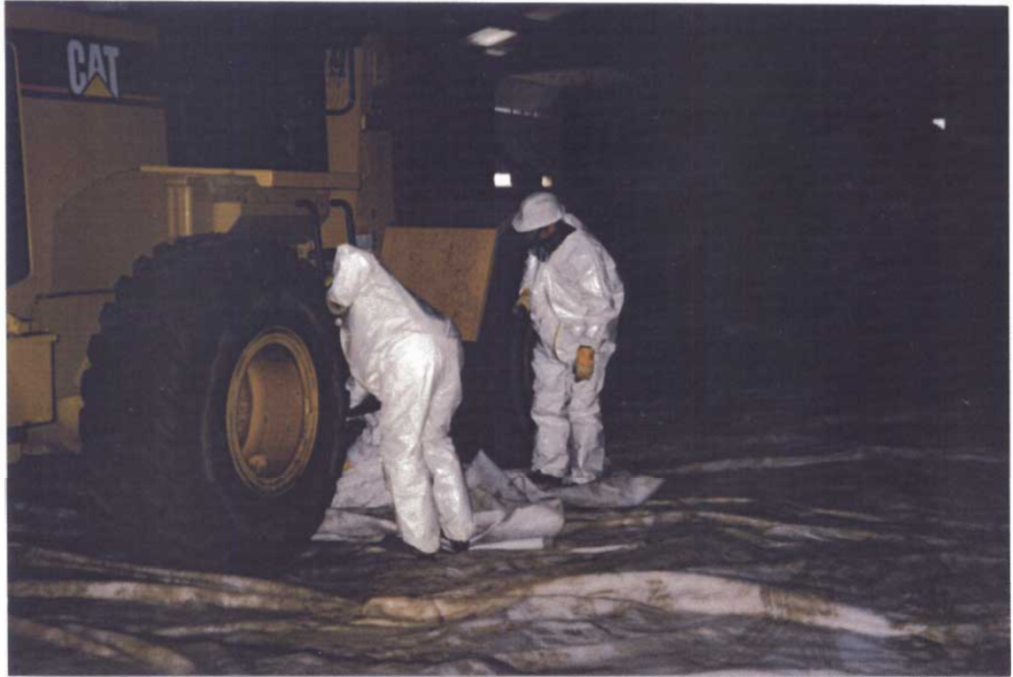
Photograph II-1: Decontaminating the Wheels of a loader in the Main PCB Storage Facility
