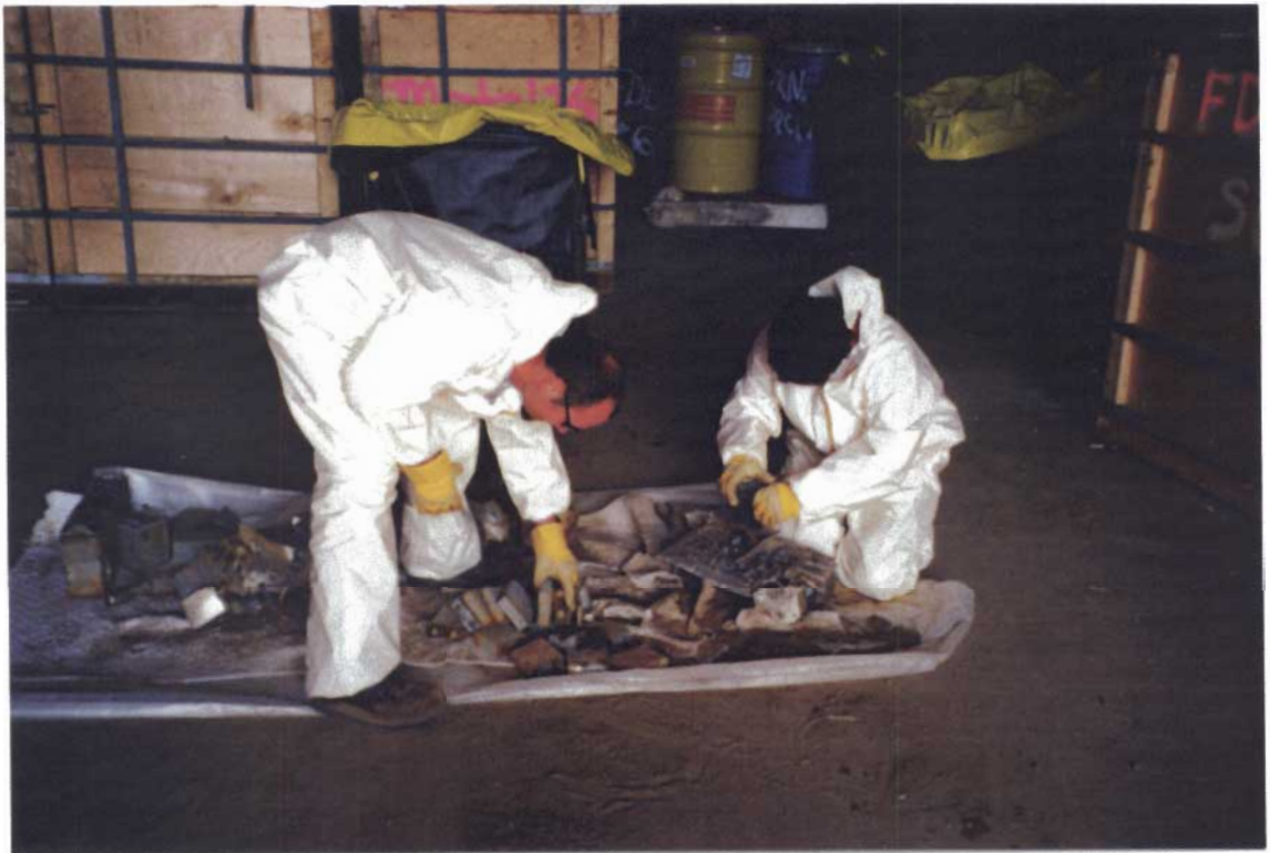
Photograph III-5: Removing Small Capacitors From Electrical Racks Taken From the Furniture Dump in 2000.
