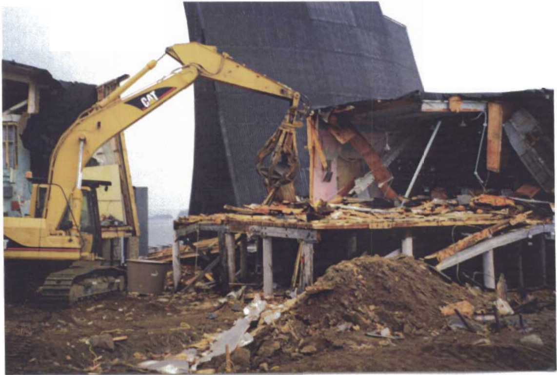
Photograph II-13: Demolishing Building S1; Note the Steel “Flower Pot” Used for Containerising > 2000 ppm PCB Soils
