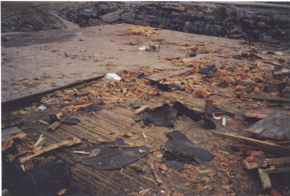
Photograph II-16: The PCB Contaminated Floor and Tar Paper; Note The Highly Contaminated Top Layer Which is Clearly Separated from the Lesser Contaminated Lower Layer of the Floor
