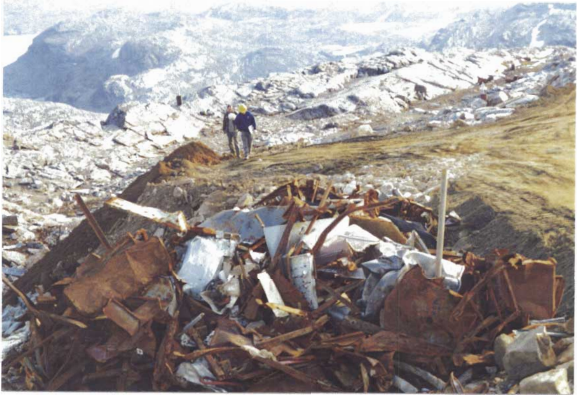
Photograph II-3: Metallic Debris and Tier II Soils from the Furniture Dump were Stockpiled on Tier II Soils in the S1/S4 Valley by the Road to S4.
