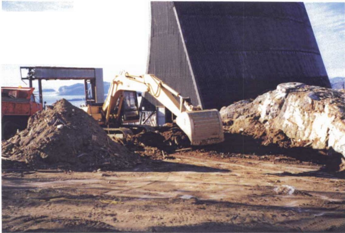
Photograph II-21: Excavating Contaminated Soil From the Area Between S1 and S2
