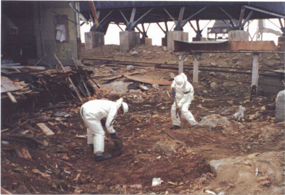
Photograph II-15: Excavating the > 2000 ppm PCB Area by S3
