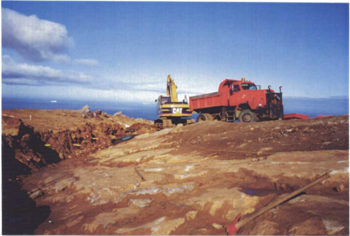
Photograph II-7: Excavation of the Furniture Dump Drainage Pathway: Note the Sloping Bedrock and Posts in the Bank Marking Sampling Points
