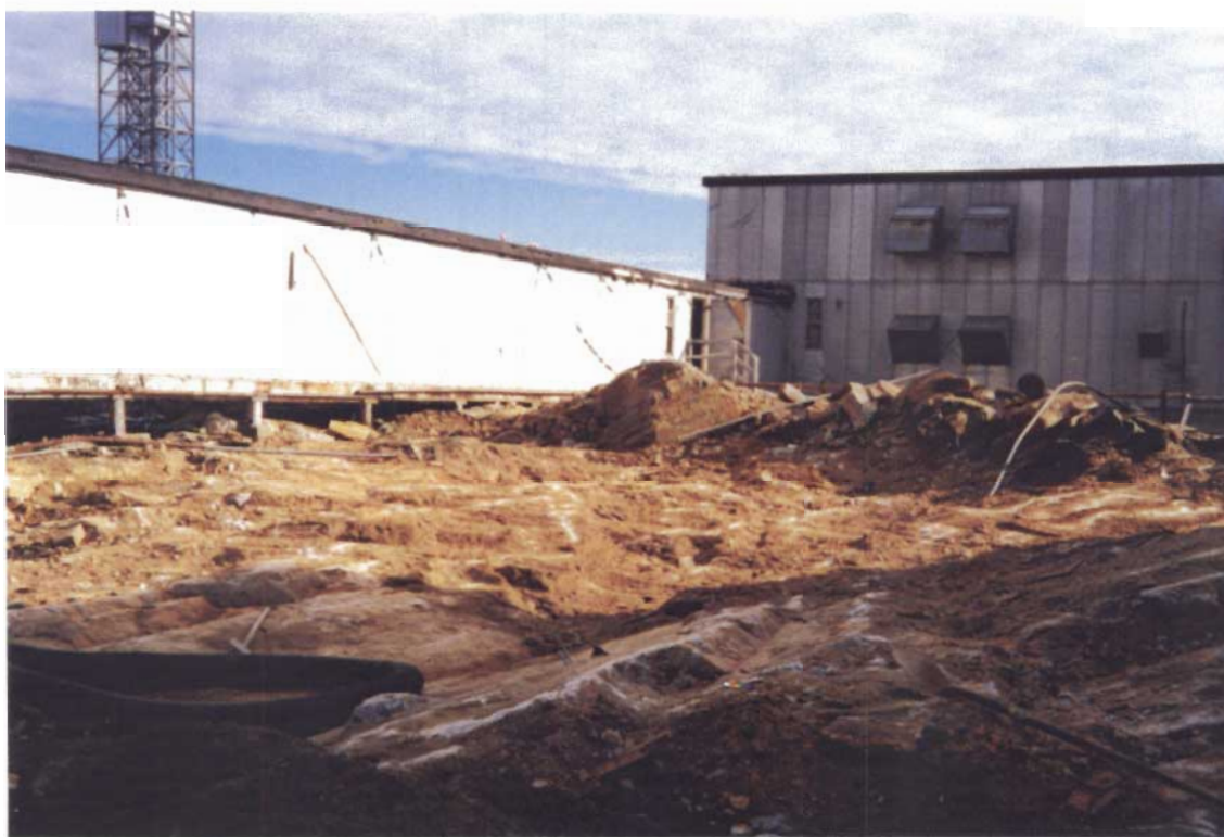
Photograph II-18: The Same Area After Excavation of the Contaminated Soil; The Clean Bedrock in the Foreground has been Vacuumed
