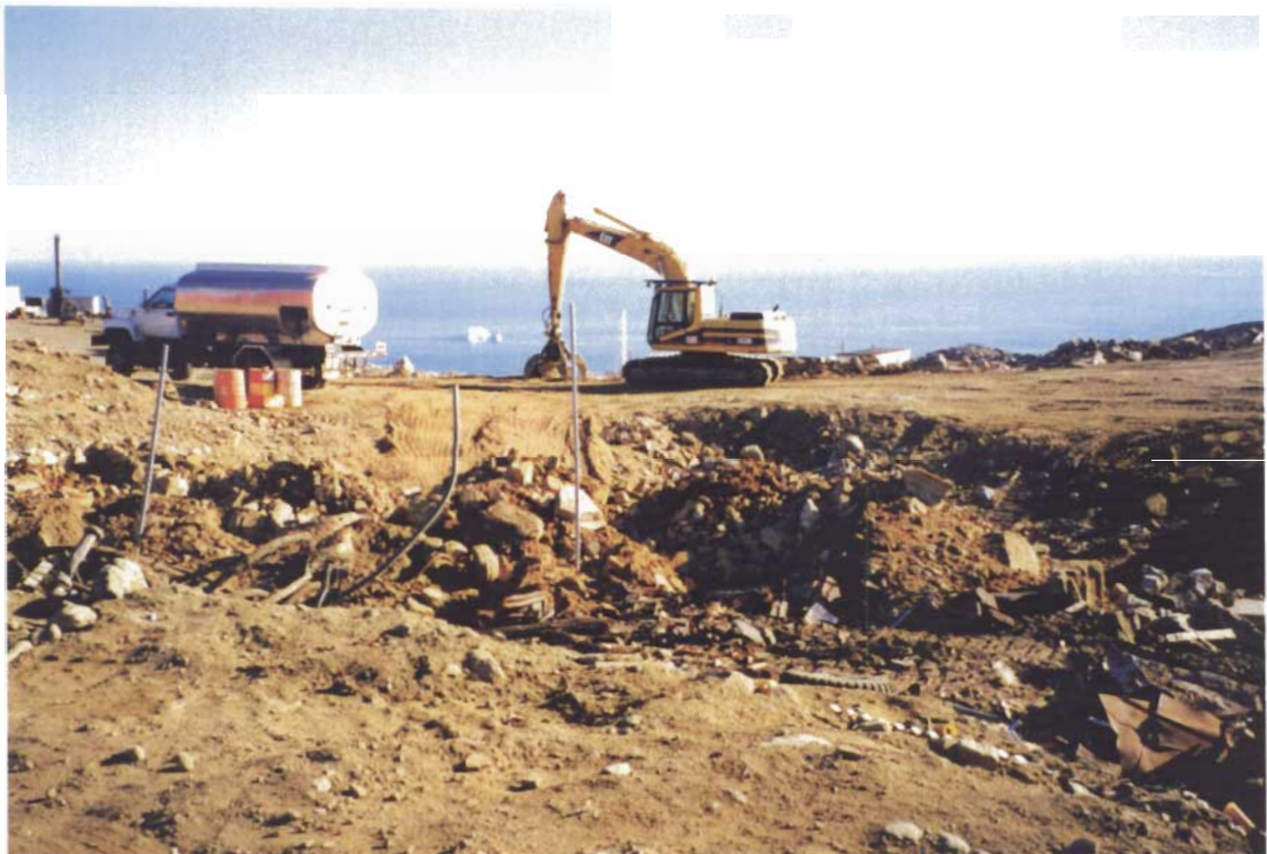
Photograph II-4: Tier I Soils from the Furniture Dump and Drainage Pathway Were Placed in a Separate Cell in the Landfill by the Core Camp
