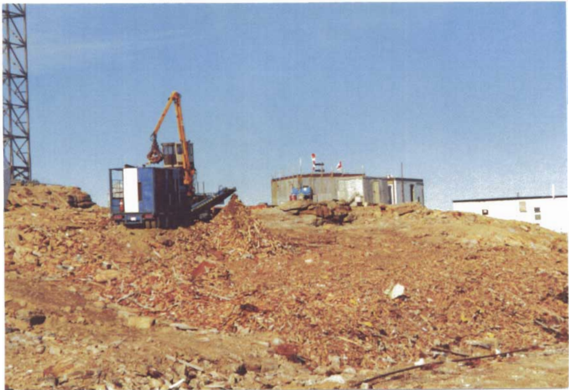
Photograph II-14: Shredding Non-Hazardous Demolition Debris Directly into the Landfill
