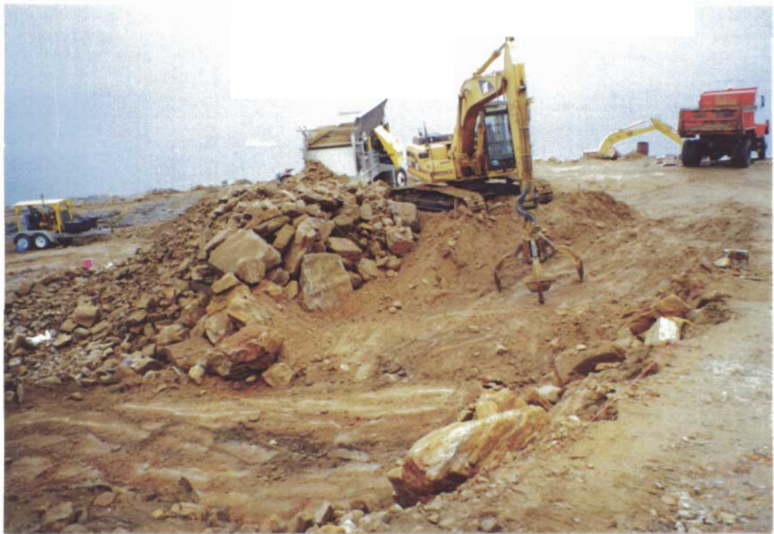
Photograph II-6: The Furniture Dump After Removing Most of the Buried Material: Note the Pile of Tier II Rocks Which Did Not Pass Through the Screener
