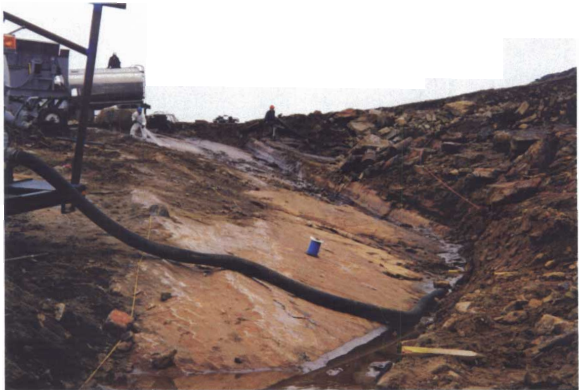
Photograph II-8: Washing the Fine Material From the Rocks to the Vacuum Truck
