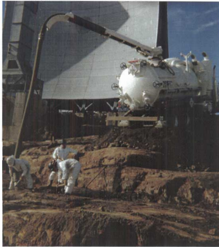
Photograph 3.3 Vacuuming of soil down the road from former building S2
