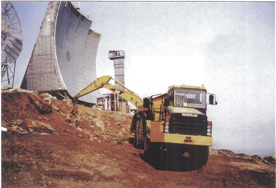
Photograph II-5: Excavating Large Boulders From the Steep Slope Along the Road From the Screening Plant Below the Buildings Area.
