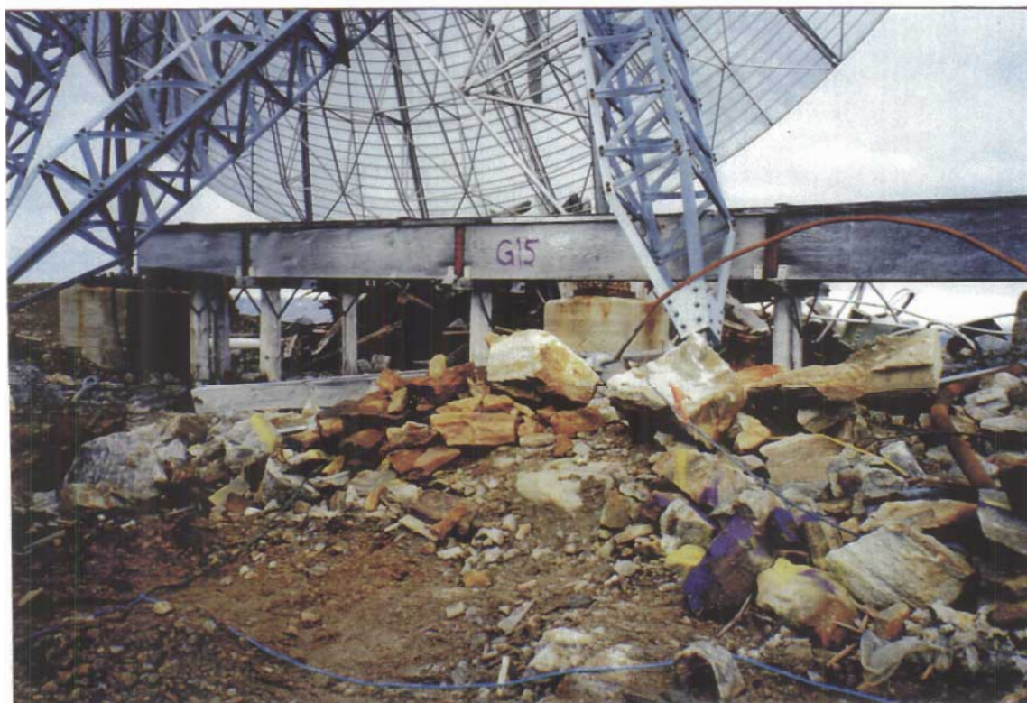
Photograph II-10: The Whole Contaminated Area Was Gridded at 20 Meter Intervals; Grids Where Labels (G15) and Corners Marked With Purple Paint.
