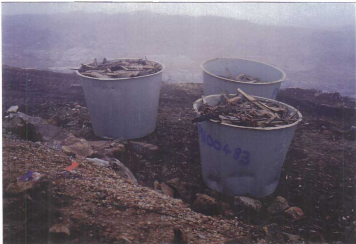
Photograph II-7: Contaminated Wood Lying on Soil Contaminated with PCBs Above the 2000 ppm Level was placed in Steel Containers.
