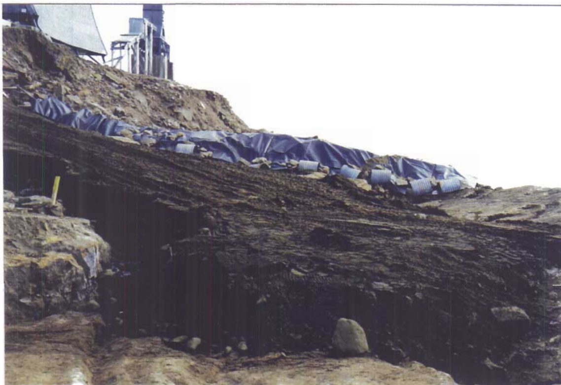
Photograph II-9: Uncontaminated Soil was Placed on Cleaned Ground and a Berm Constructed to Prevent Recontamination of the Area Over Winter.
