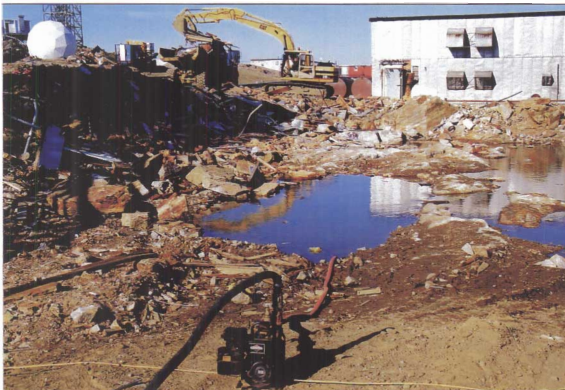
Photograph II-1: Demolition of the Corridor That Links Buildings S3 and S4; and Pumping Water From the S3 Area.
