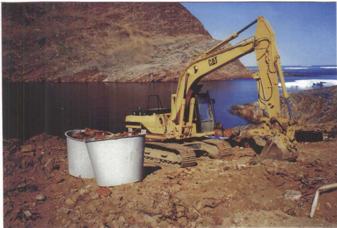
Photograph II-14: Placing Material Contaminated with a Formulation Containing Amyl Acetate into Steel Containers.
