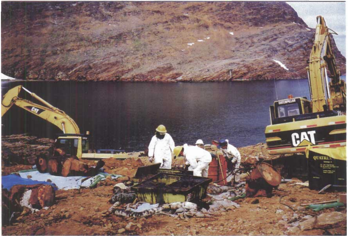
Photograph II-13: Pumping the Contents of Rusty Fragile Barrels into Sound Barrels at the Beach Dump.
