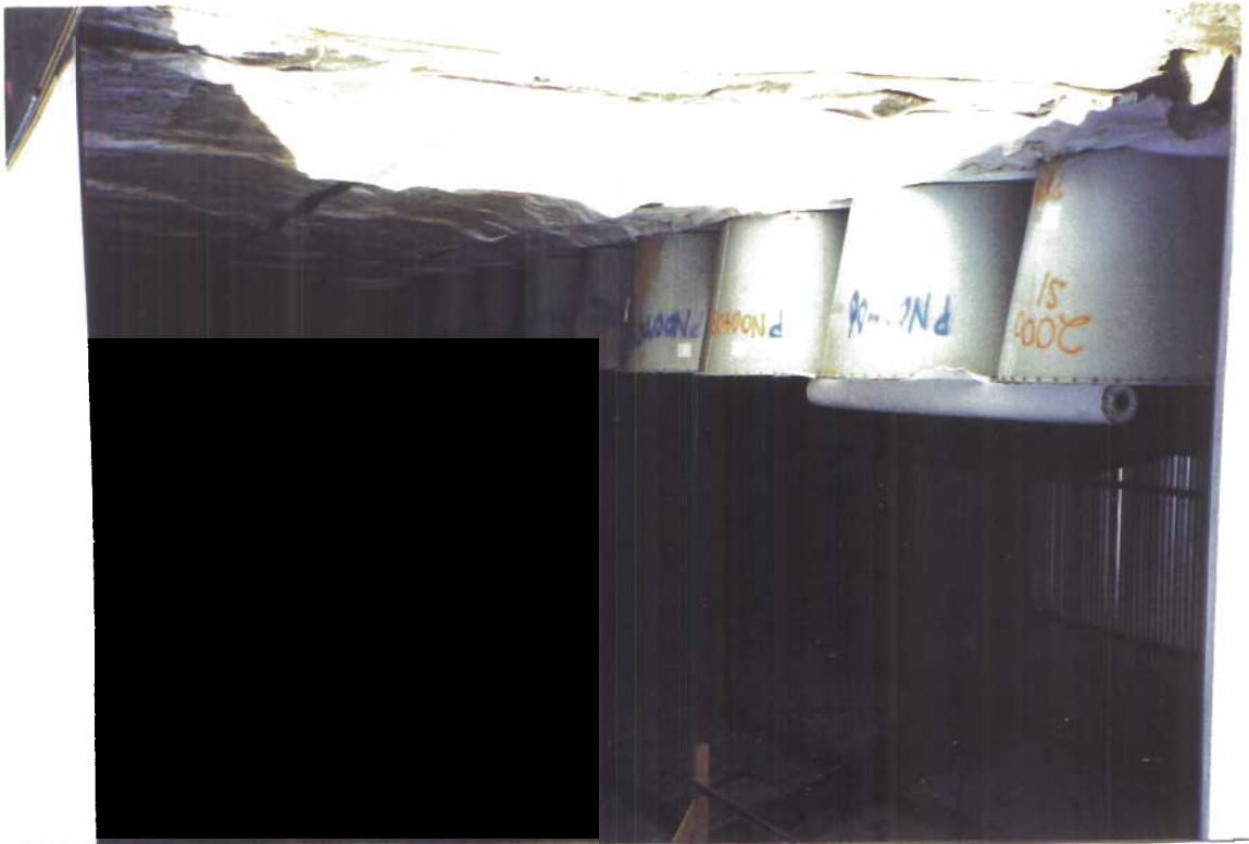
Photograph III-2: Steel Containers Within the Building at the Main PCB Storage Facility; These Containers Leaked and Were Therefore Placed Inside on the Liner.
