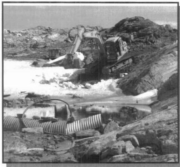
Photograph 3.1 Removing snow and water from S1/S4 valley prior to excavation
