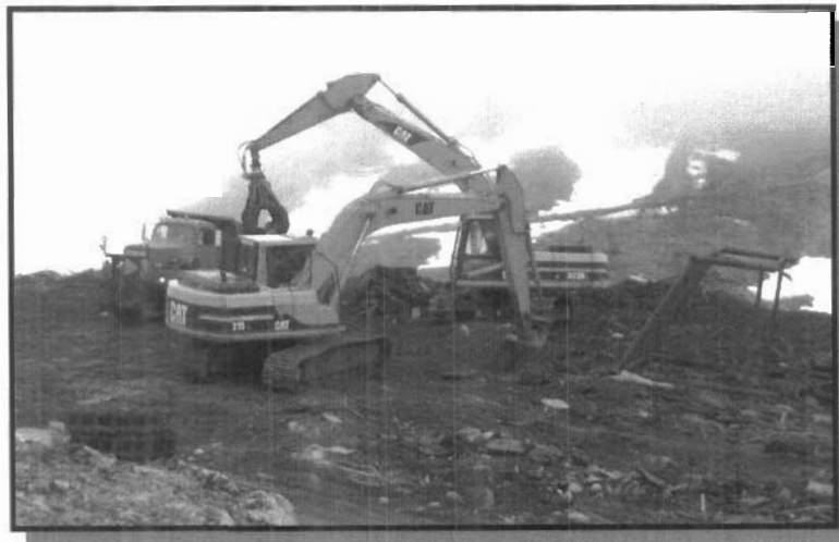
Photograph 3.2 Excavation of CEPA soil at the Airstrip Dump
