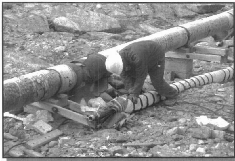
Photograph 5.3: Removal of asbestos insulation from old fuel line
