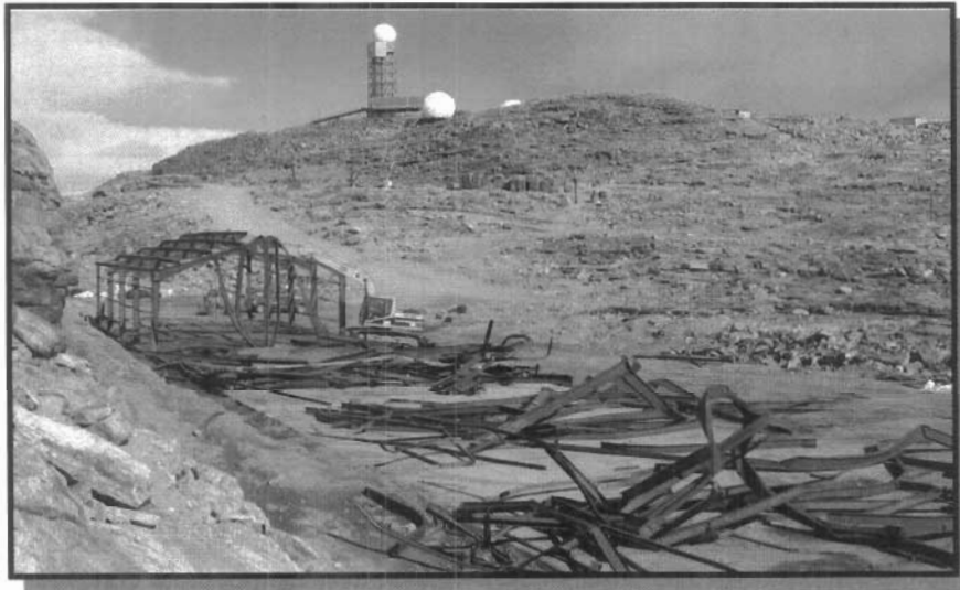
Photograph 5.2: Demolition of building structural steel frame
