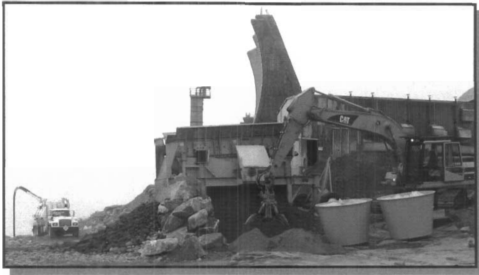
Photograph 4.1 Containerization of CEPA soil from S1/S4 screener
