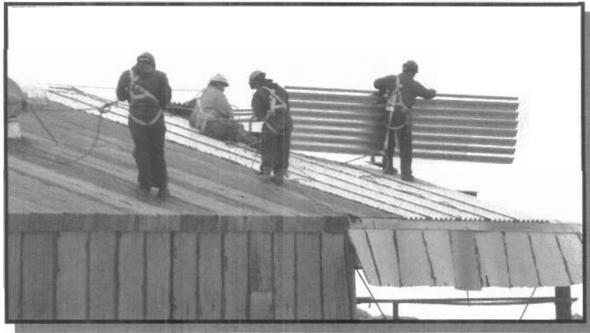
Photograph 5.1: Removal of steel cladding from PCB building roof
