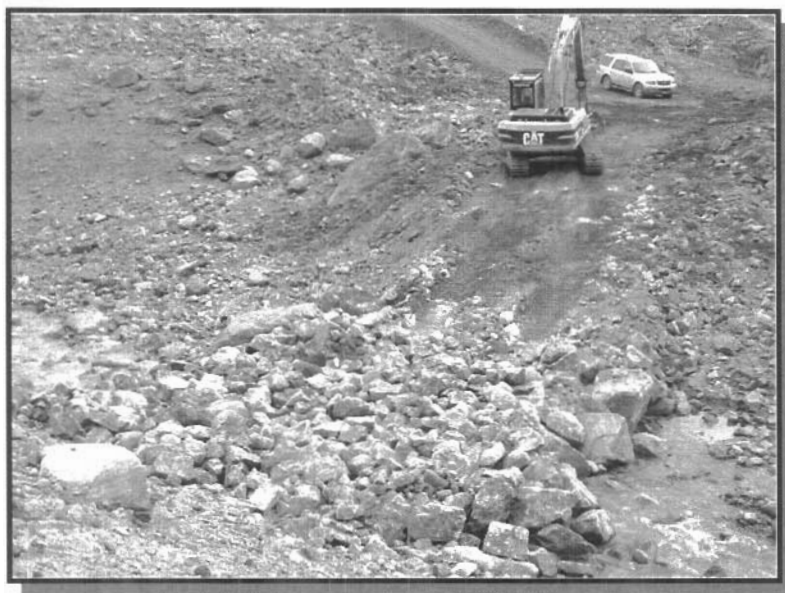
Photograph 8.1 Layer of boulders across streambed
