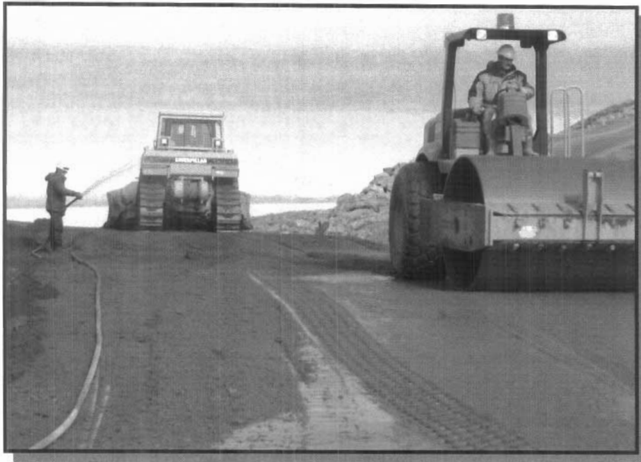
Photograph 7.3: Construction of the south berm core
