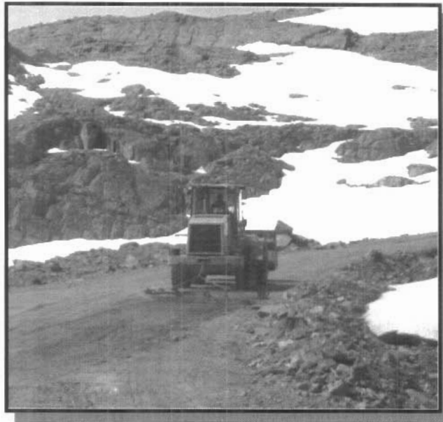
Photograph 8.2 Grading of main site road
