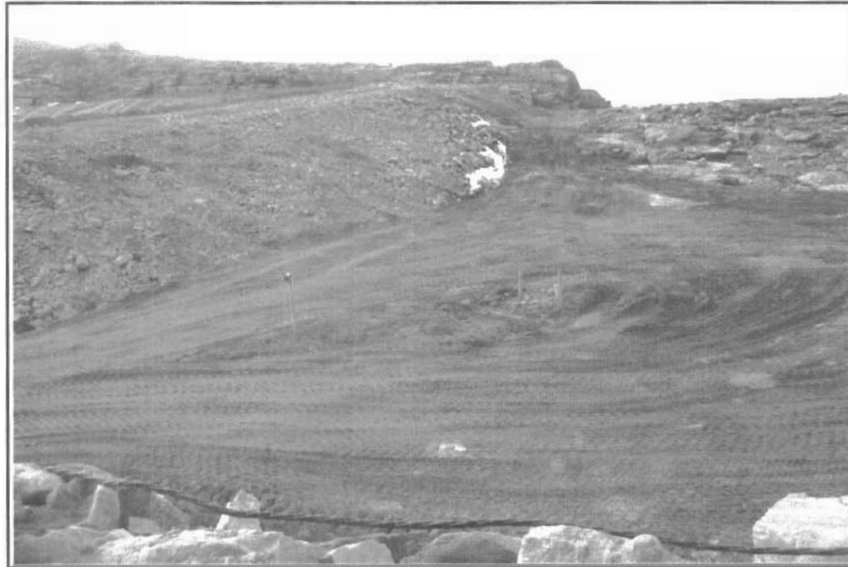
Photograph 5.3: Area east of East berm backfilled and sloped towards the southwest; monitoring well MW-1 approximately 10 m from the toe of berm
