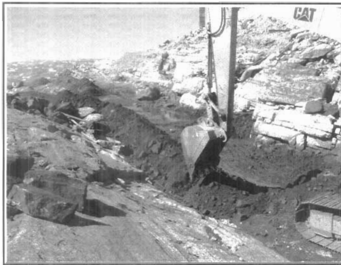
Photograph 3.2: Excavation of PCB Tier II soil - S1/S4 Valley
