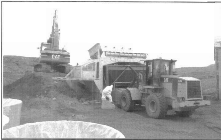
Photograph 4.1: CEPA soil screening and containerization behind B2 building
