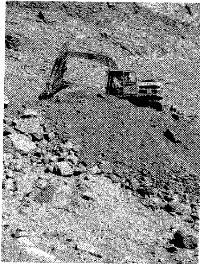
Photograph 3.1: Excavation of CEPA soil at the bottom of the cliff - S1/S4 beach
