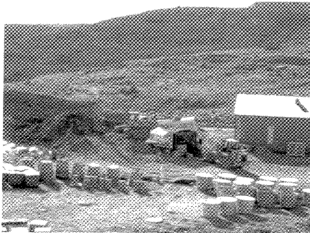
Photograph 4.1: CEPA soil screening and containerization behind B2 building
