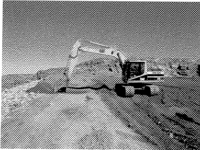
Photograph 5.5: Soil removing from the berms
