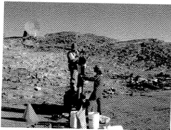
Photograph 5.8: Thermistor installation and filling
