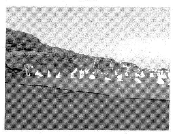
INSTALLATION OF GEOSYTHETICS PRODUCTS HDPE 1,5 MM (60 MIL) SMOOTH
