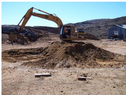
Photograph 5.1.: HC contaminated soil excavation
