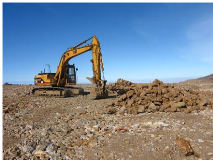
Photographs 4.18 to 4.19: Spreading of type 1
