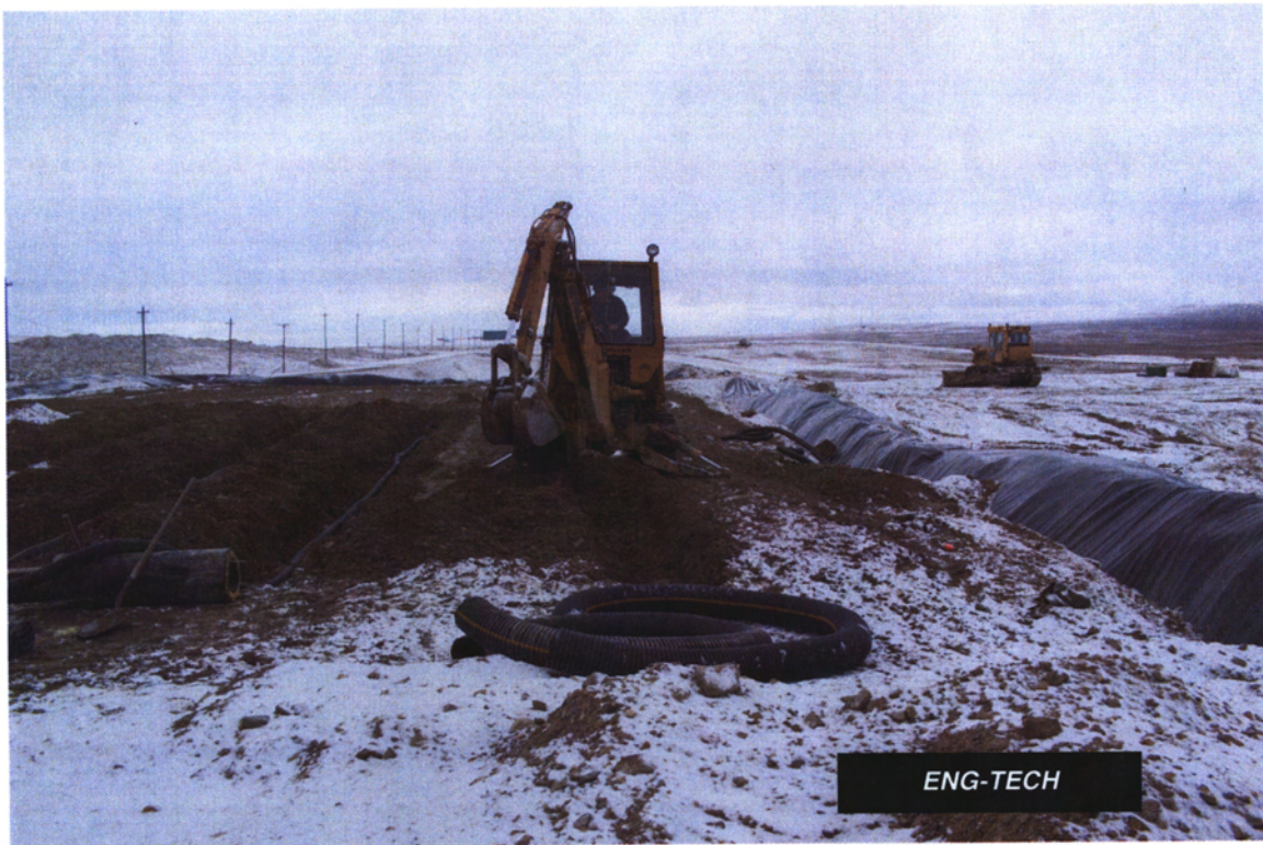
Photograph 1 – Excavation for pipe installation of ground heating system.
