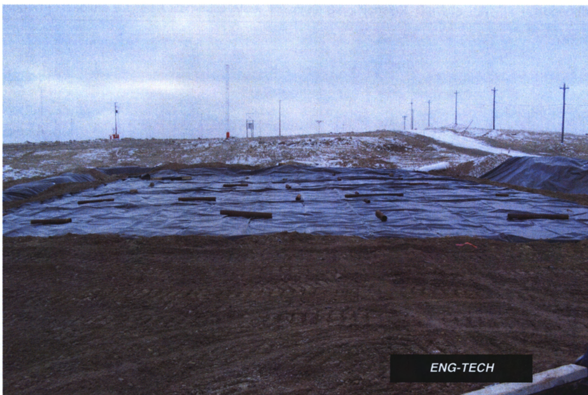
Photograph 5 – Final cover over ground heating system.
