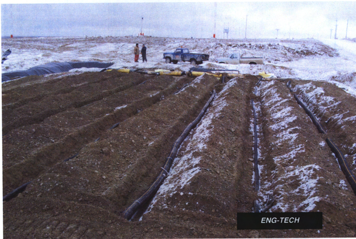
Photograph 2 – Pipes set in ground for heating system.
