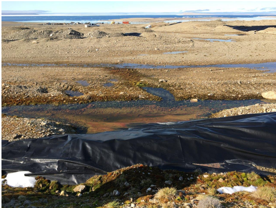
Photograph 2: Potential berm breach along west berm of LTU 2, August 22, 2018.
