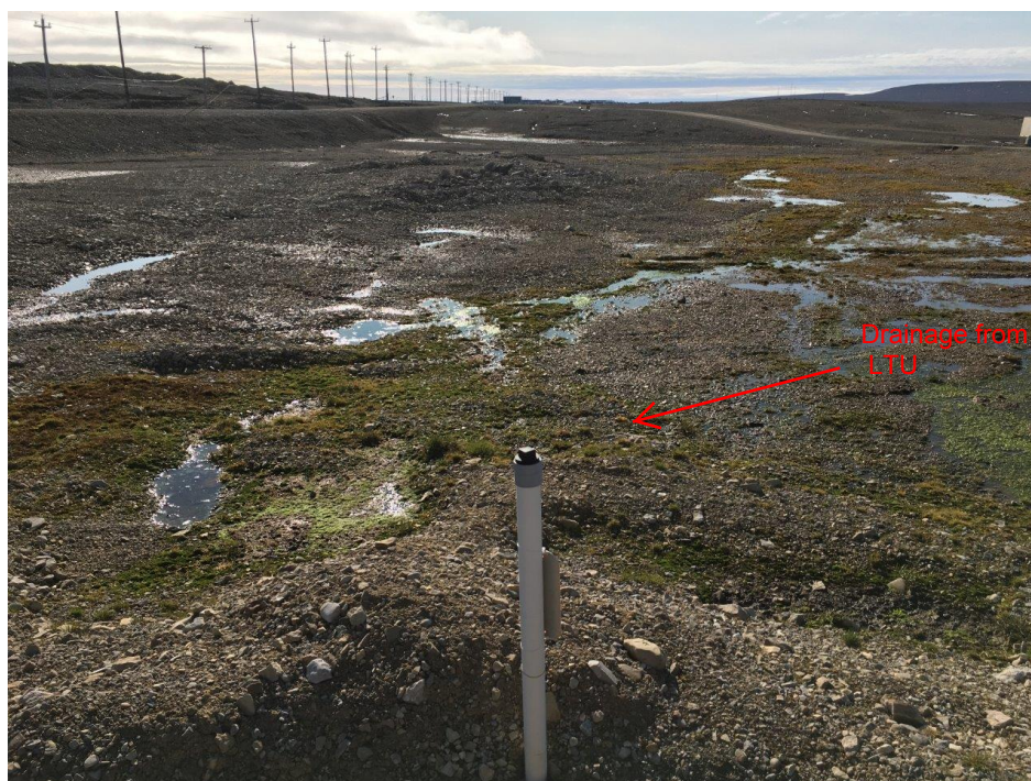
Photograph 4: South view of potential berm breach in southwest corner of LTU 2, August 22, 2018.
