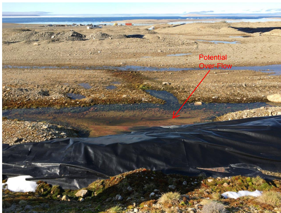
Photograph 5: Potential berm breach along west berm of LTU 2, August 22, 2018.
