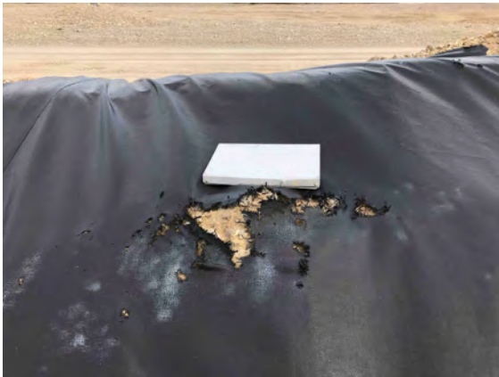
Photo 25 Liner tear 5 m south of northeast corner of LTU 2 (Liner Deficiency 14)
