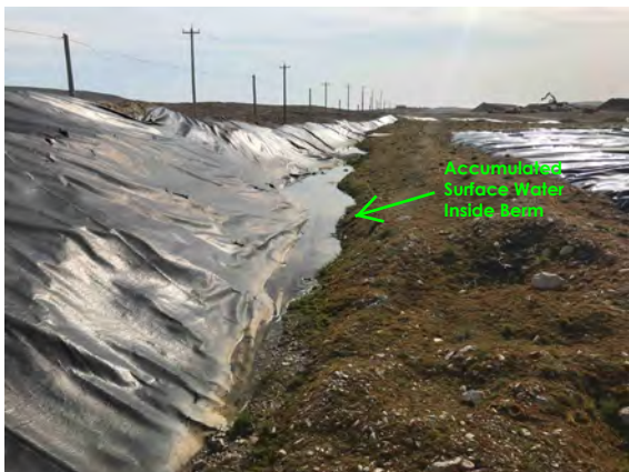
Photo 11 View of accumulated surface water in LTU 2 (along east berm) looking south (Liner Deficiency 20)
