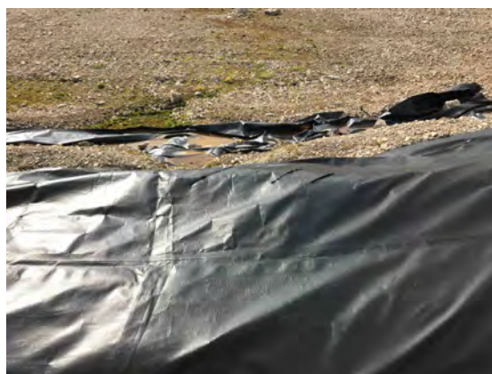
Photo 14 Liner tears near northwest corner of LTU 1 (Liner Deficiency 2)
