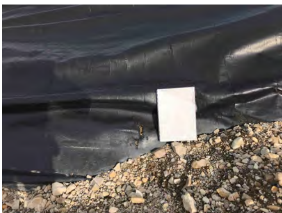
Photo 17 Liner tear north of southeast corner of LTU 1 (Liner Deficiency 5)
