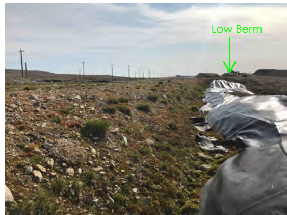
Photo 30 North view of low berm north of access to LTU 2 on west berm (Liner Deficiency 19)
