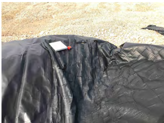
Photo 13 Liner tears near north corner of LTU 1 (Liner Deficiency 1)
