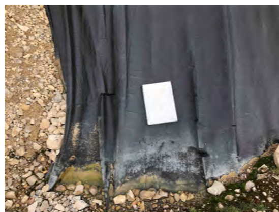
Photo 24 Liner tears 2-2.5 m south of northeast corner of LTU 2 (Liner Deficiency 13)
