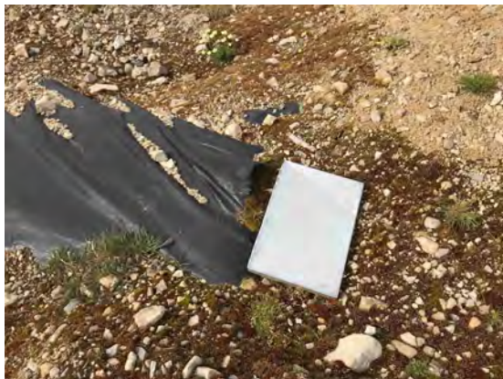
Photo 19 Liner tear 11.5 west of the northeast corner of LTU 2 (Liner Deficiency 7)
