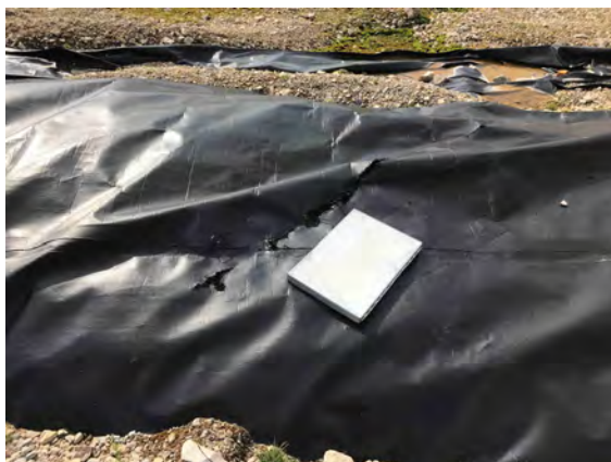
Photo 15 Liner tears near northwest corner of LTU 1 (Liner Deficiency 3)
