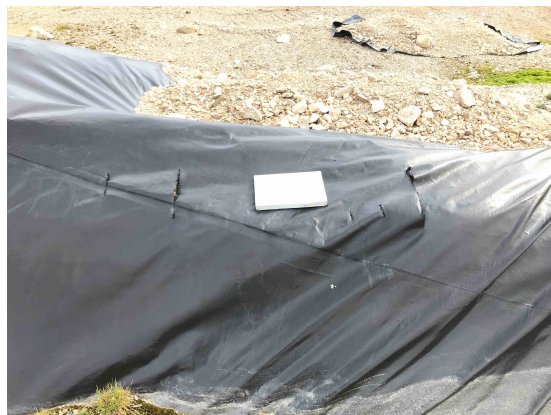
Photo 22 Liner tears 16-17 m east of southwest corner of LTU 2 (Liner Deficiency 11)
