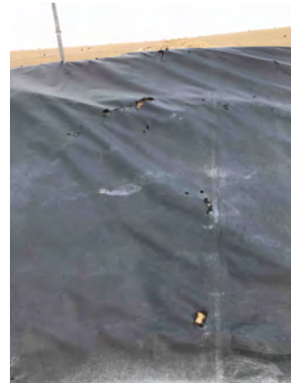
Photo 26 Liner tears 7 m south of northeast corner of LTU 2 (Liner Deficiency 15)
