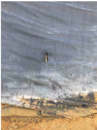
Photo 27 Liner tear 9 m south of northeast corner of LTU 2 (Liner Deficiency 16)
