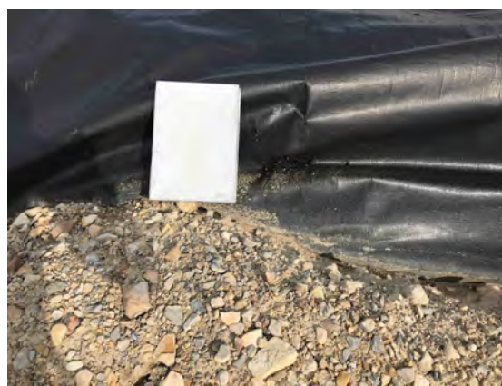
Photo 18 Liner tear north of southeast corner of LTU 1 (Liner Deficiency 6)
