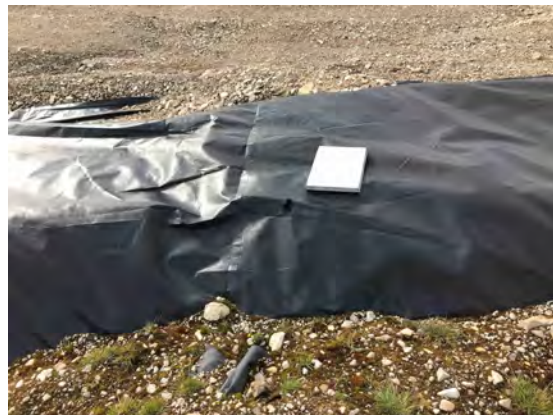
Photo 20 Liner Tear 13 m south of northwest corner of LTU 2 (Liner Deficiency 8)
