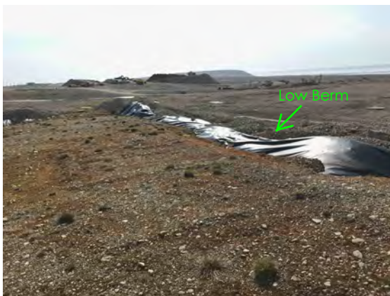
Photo 29 West view of low berm area south of access to LTU 2 on west berm (Liner Deficiency 18)
