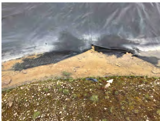
Photo 23 Liner tear 13-17 m south of northeast corner of LTU 2 (Liner Deficiency 12)
