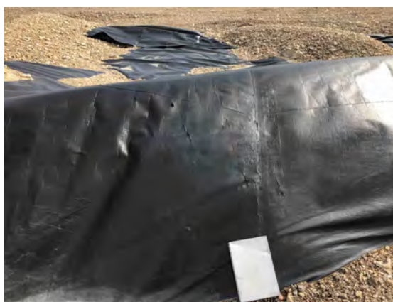
Photo 16 Liner tears near southeast corner of LTU 1 (Liner Deficiency 4)
