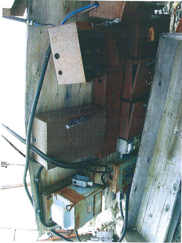
Photo 29: Dry transformer and electrical panel in Garage
