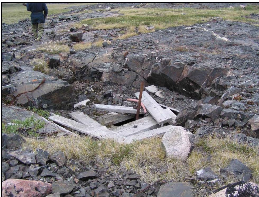
Photo 34. Partially covered vent raise
