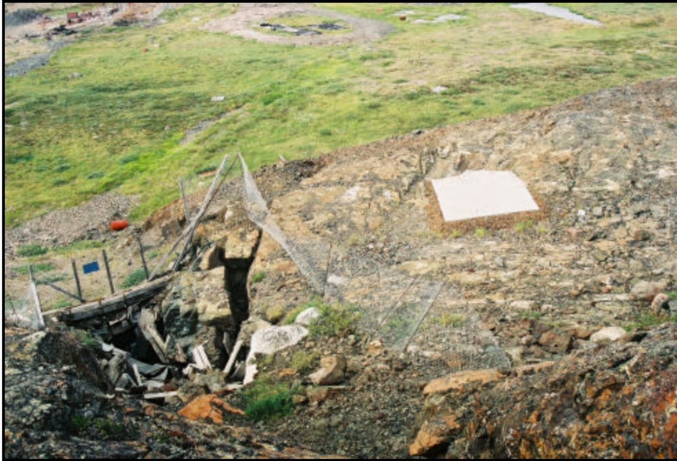
Photo 27. Mine shaft and concrete covered ventilation raise.
