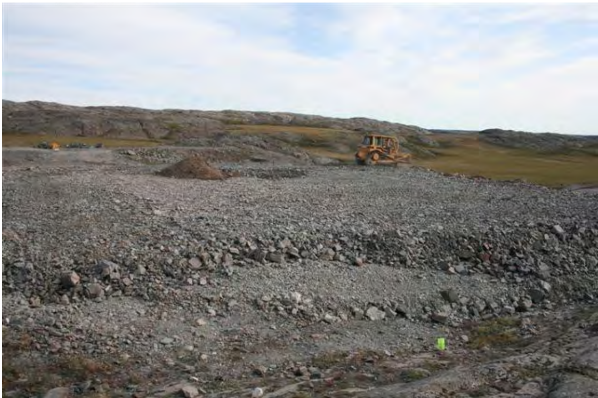
Placement of final cover on Solid Waste Disposal Facility (at the former tailings containment area) – post remediation
