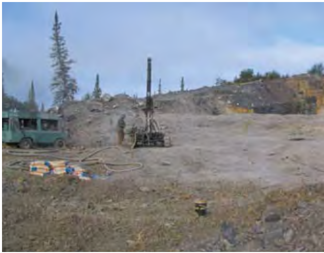
FIGURE 22. Extraction of rock involves drilling and blasting.
