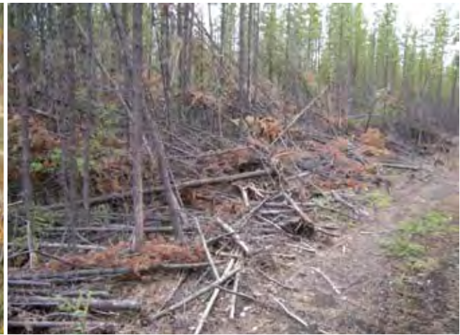
FIGURE 18. Leaning trees should be cut down and stacked into windrows.
