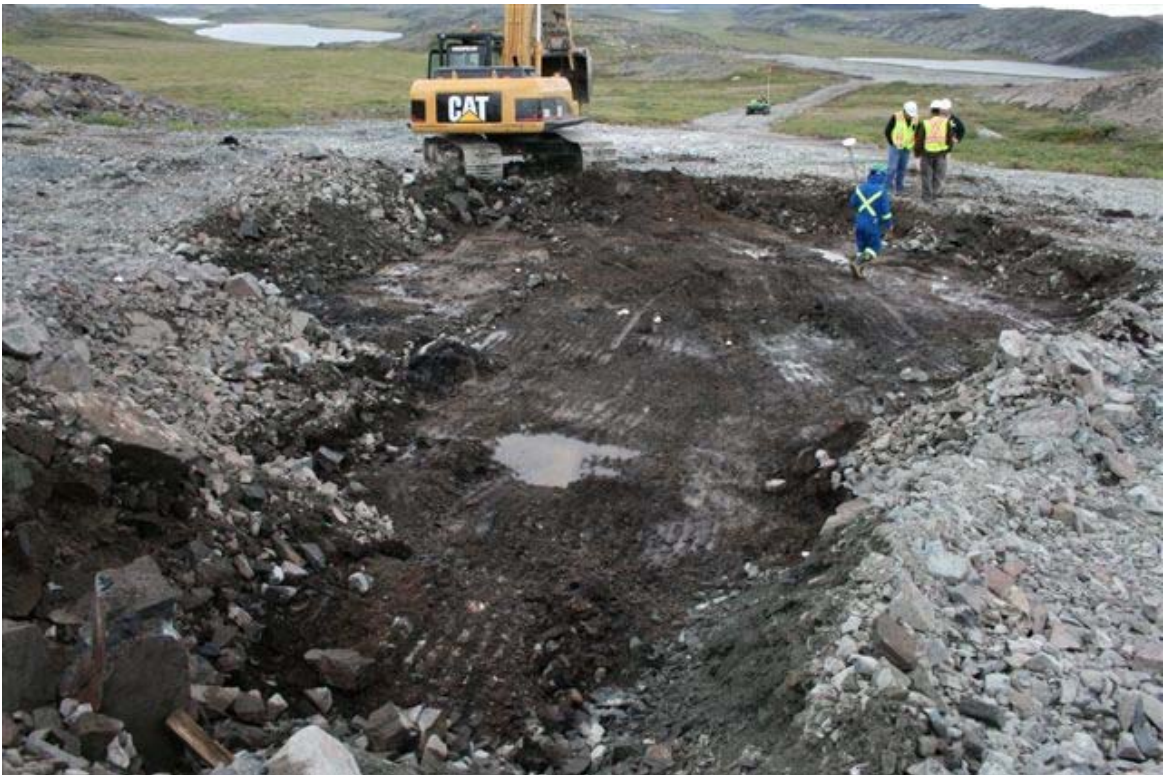
Photograph No. 52: Petroleum Hydrocarbon remediation at Garage Area of Roberts Bay
