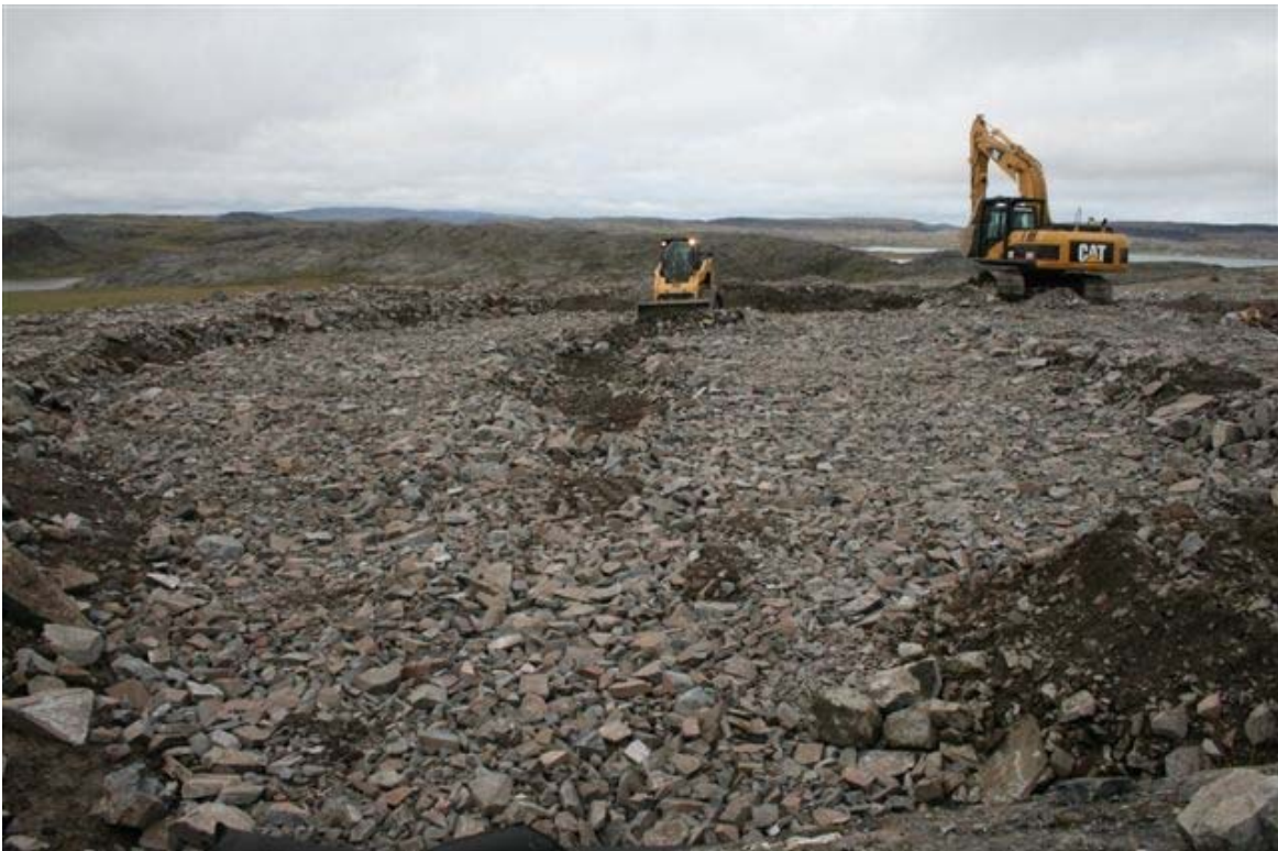
Photograph No. 68: Final Cover Placement Works
