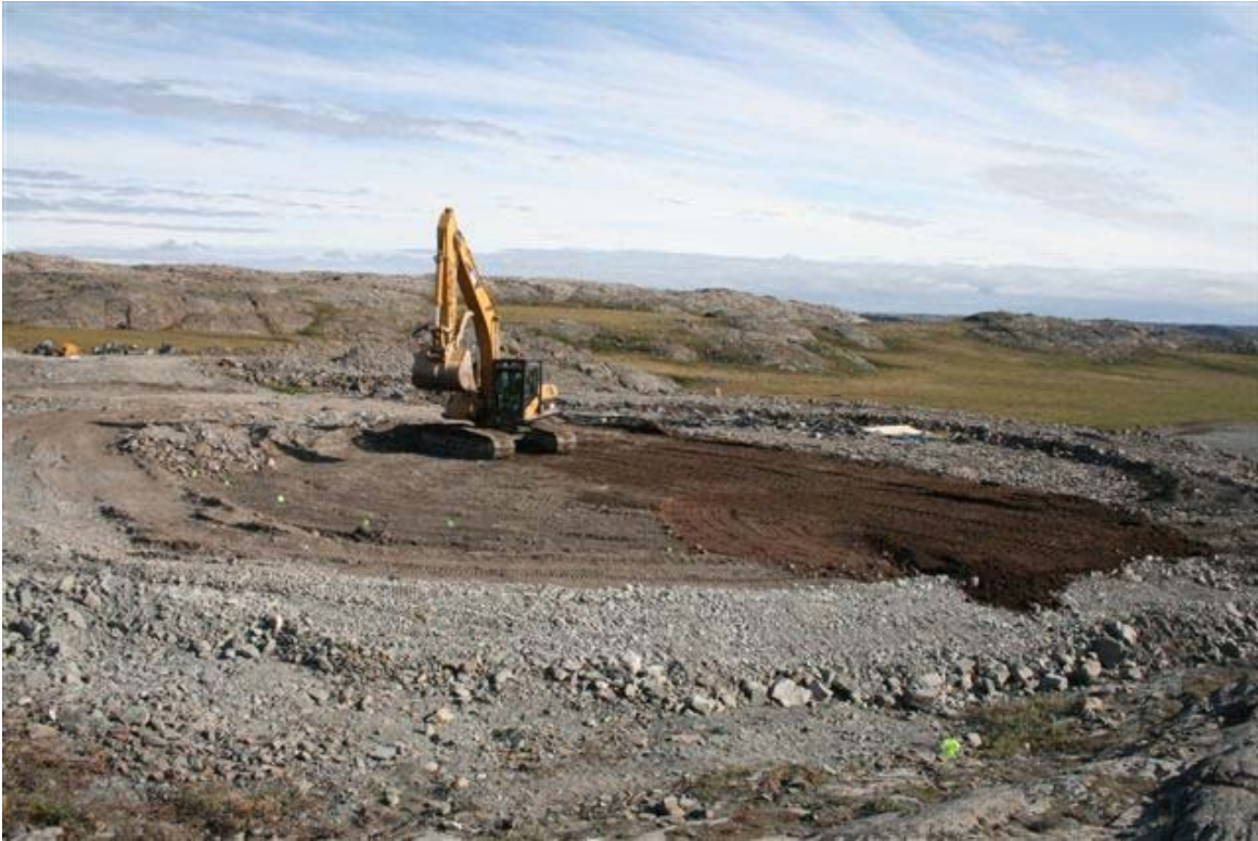
Compacting Type 2 material over the debris in the dry cell.
