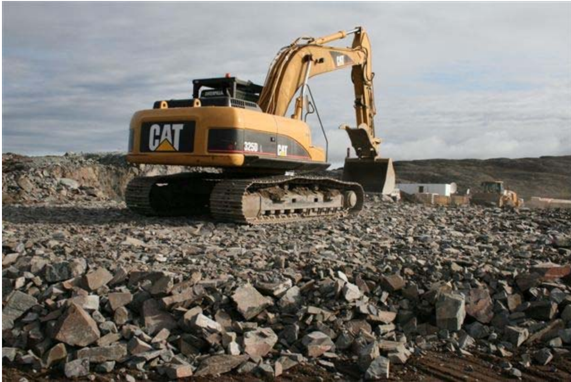
Compacting type 1 cap over the dry cell
