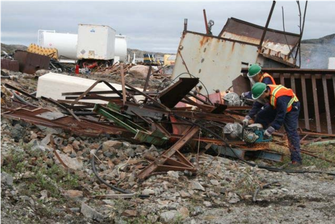
Cutting crew cutting debris hauled from the vicinity of the mill
