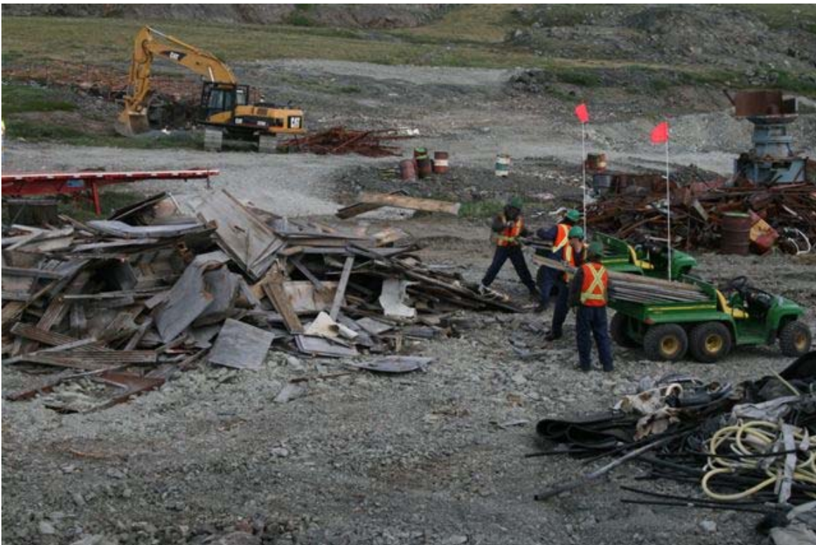
Two “Gators” were used to haul debris. Crew is offloading wood debris
