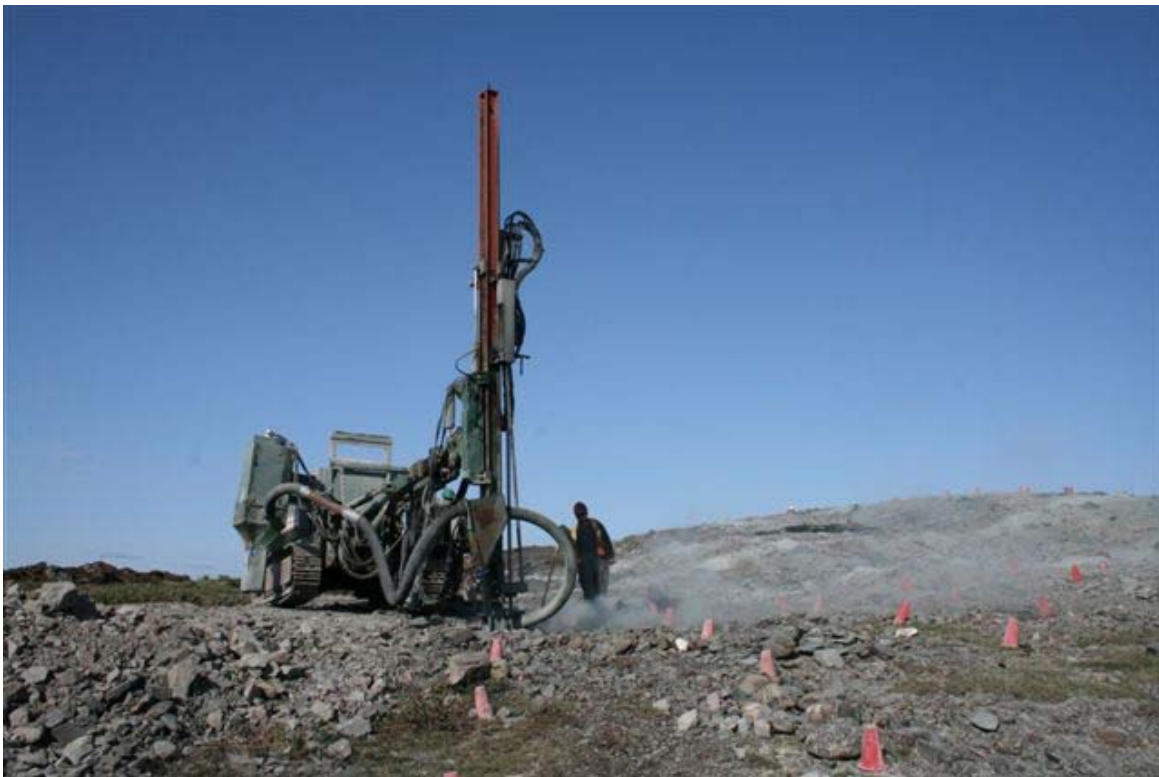
Neyo Drilling and Blasting north of the tailings pond.
