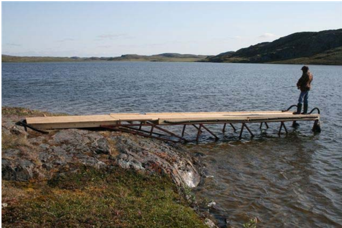
New dock constructed at Roberts Lake. Frame is trusses from the mill.
