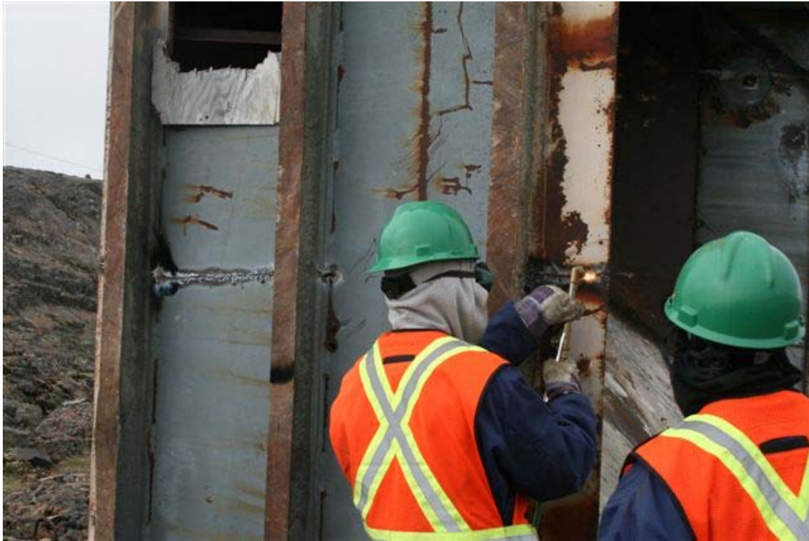
Workers cutting hopper with torch.
