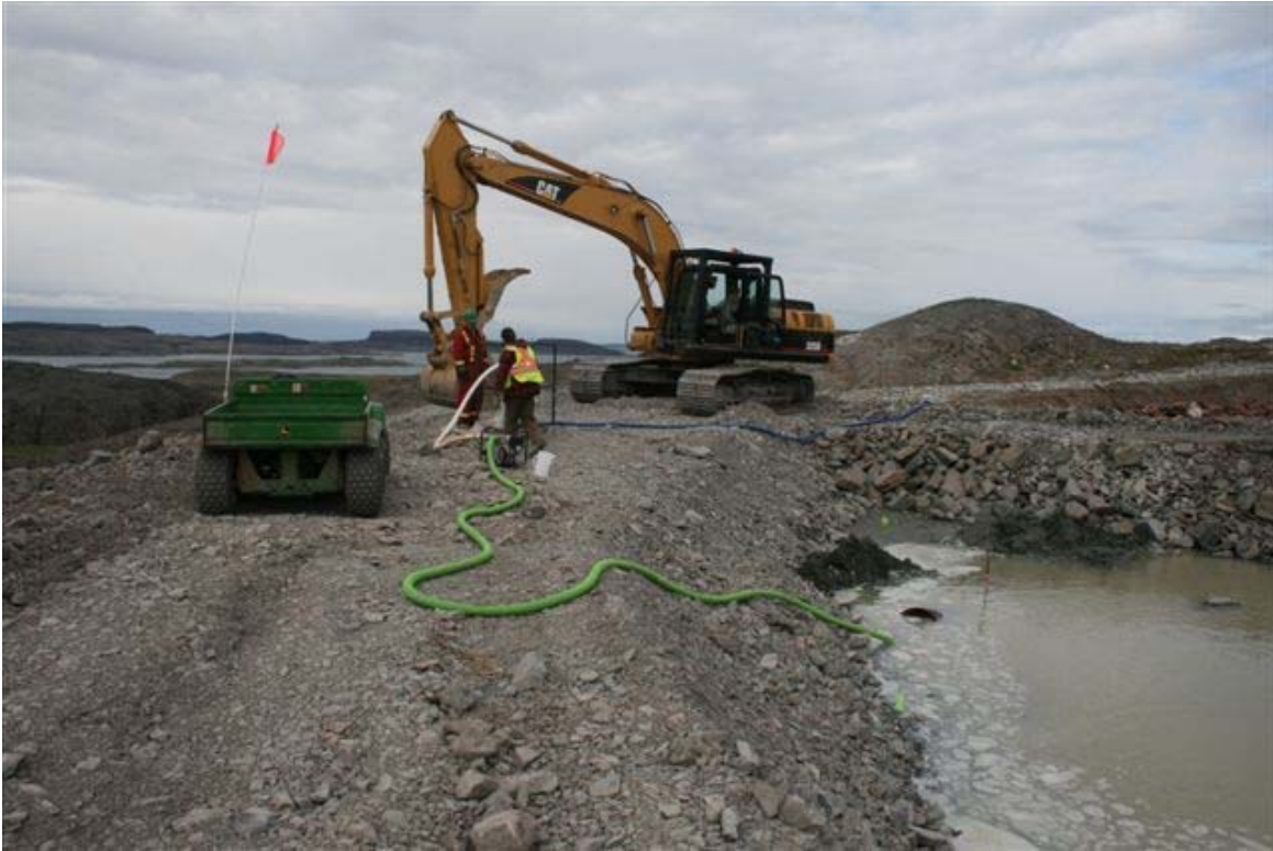
Pumping system set up. Worker is at the filtering device
