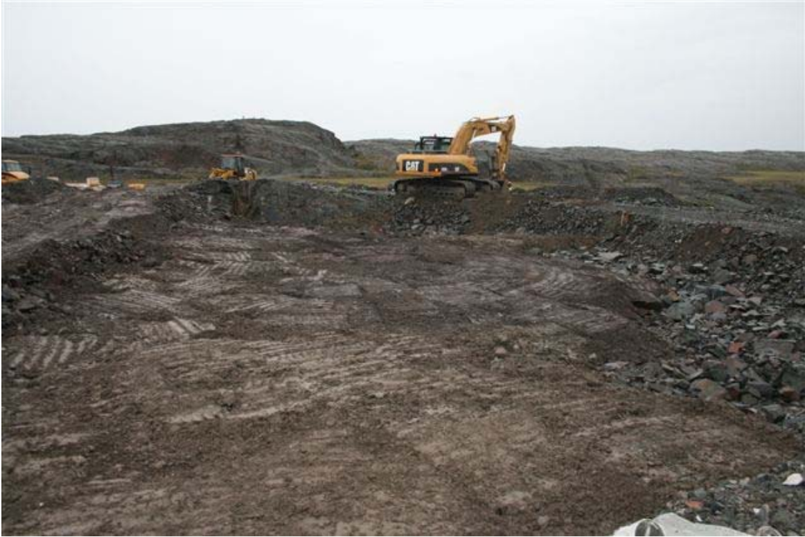
Photograph No. 65: Capping of debris in SWMF during construction
