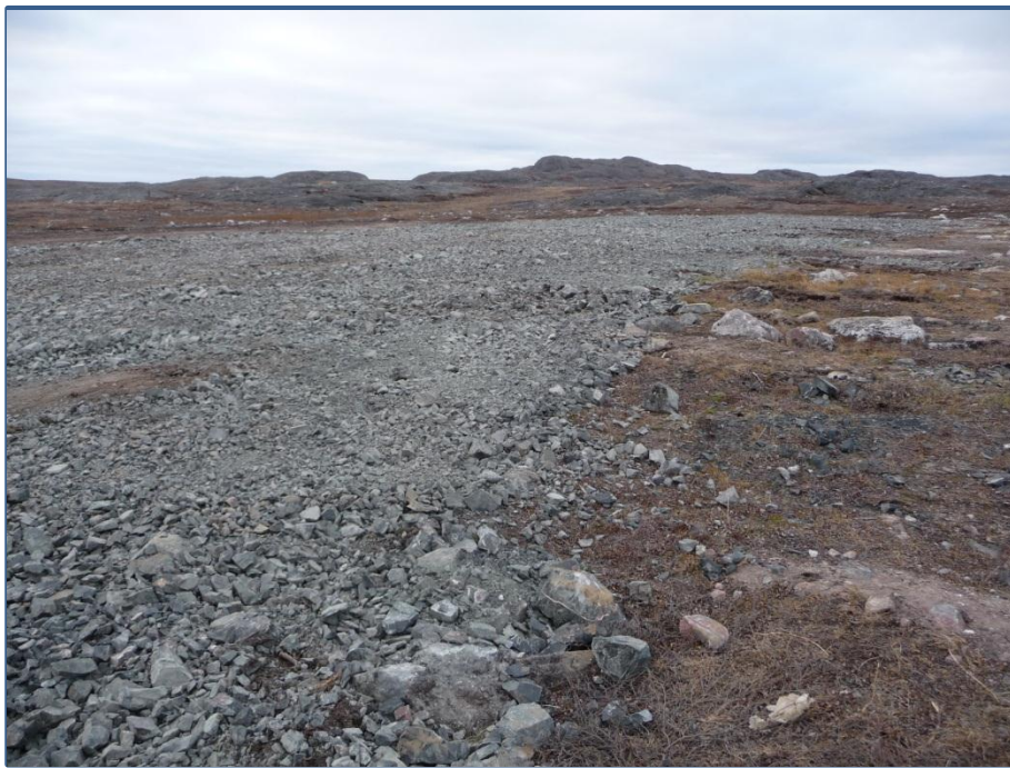
Wasterock Feathered Out to Match Topography from Southeast - After
