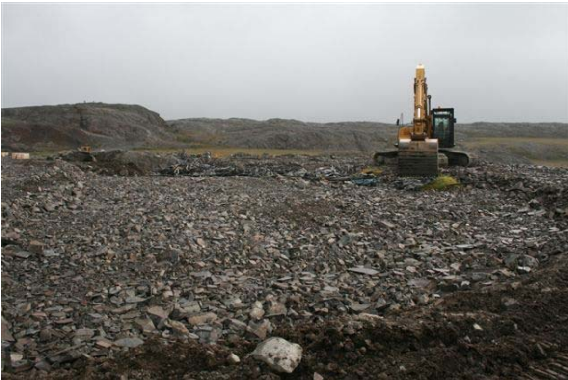
Debris placement in wet cell.
