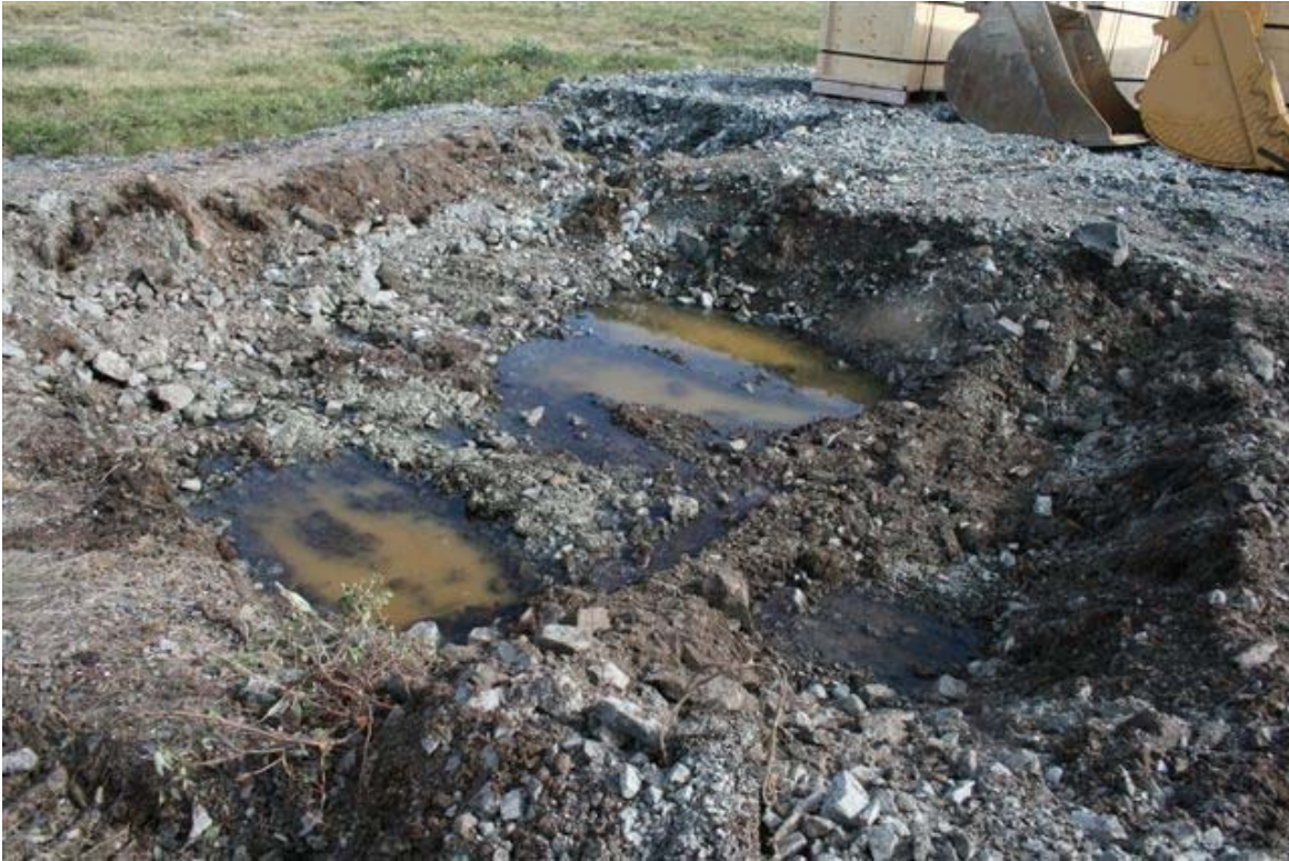
Excavation in muskeg area. Volume 18 cu.m.
