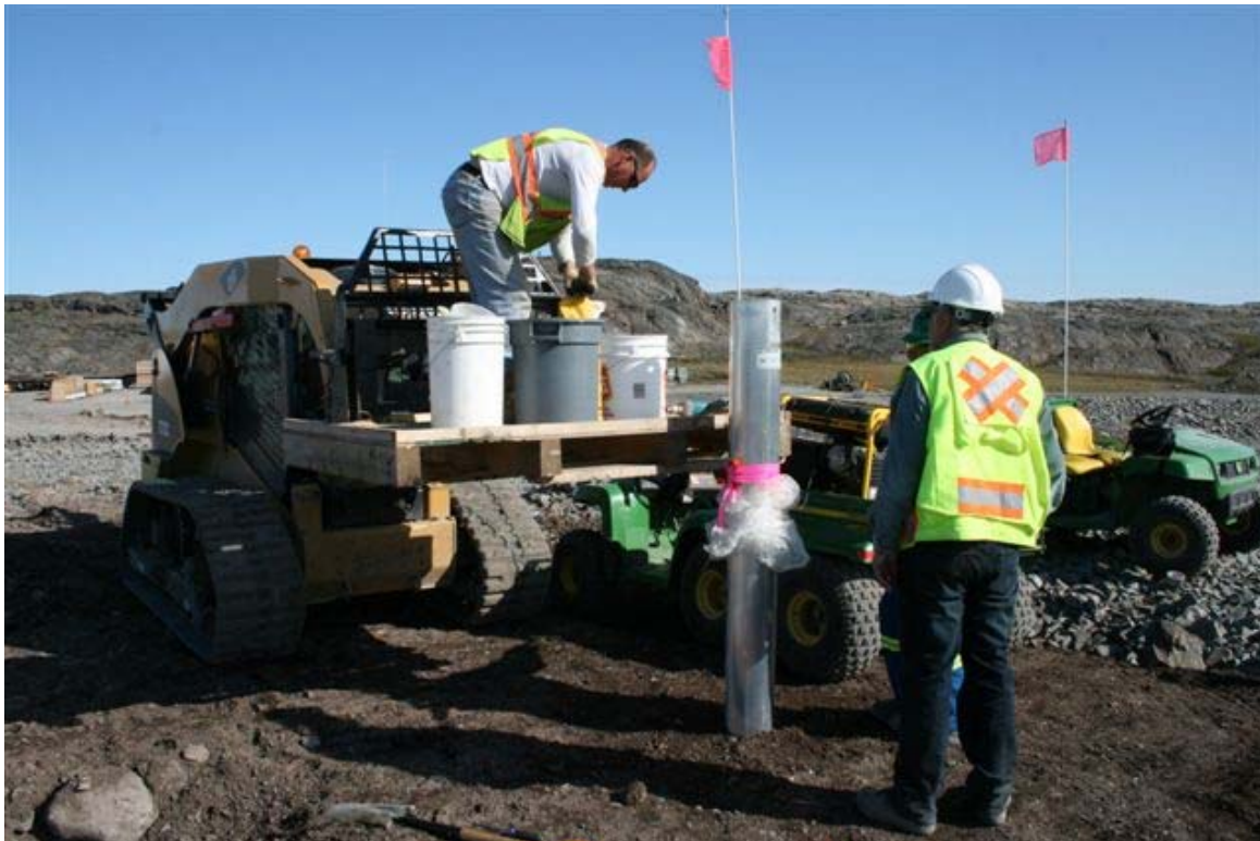
Preparing to grout thermistor A
