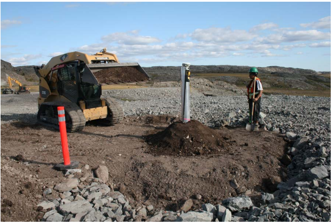
Photograph No. 73: Thermistor Installation
