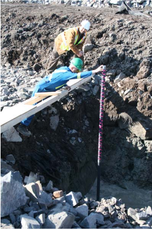
Photograph No. 72: Thermistor Installation
