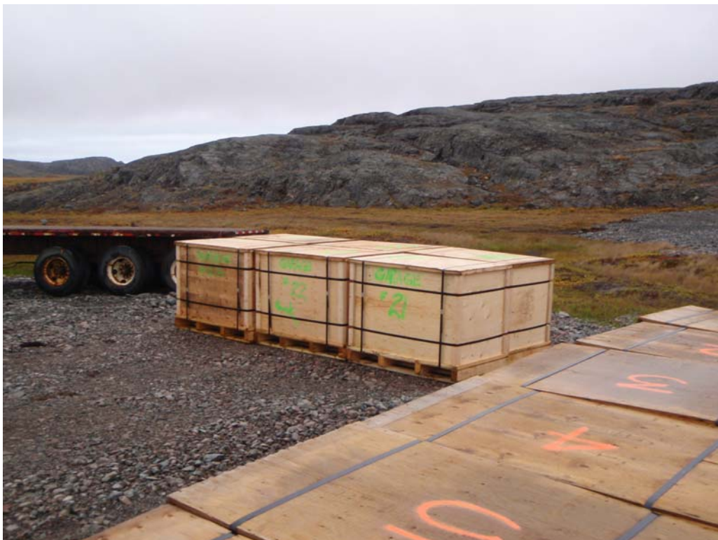
Containerized Impacted Soils.
