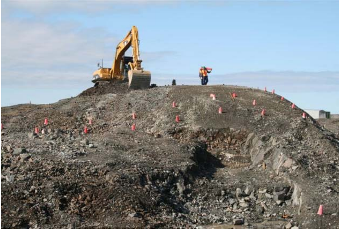
Neyo Drilling and Blasting laying out drill hole patterns
