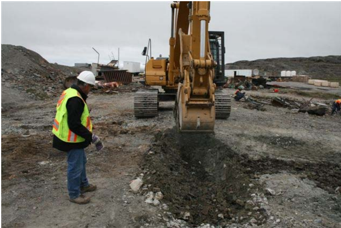
Test strip at mill site. Bedrock is ~ 300 mm depth. All material within the footprint of the mill will be excavated down to bedrock and removed off site.
