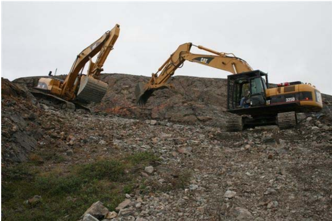
Excavators backfilling at vent raise and adit 2
