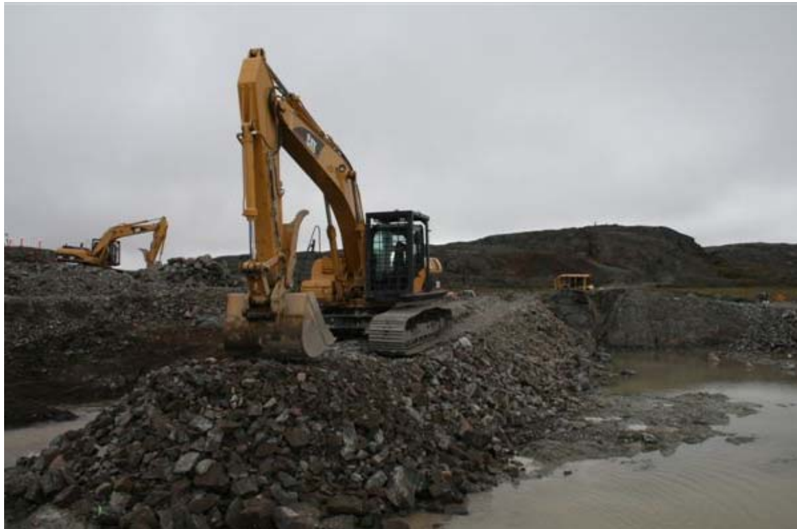
Intermediate berm under construction
