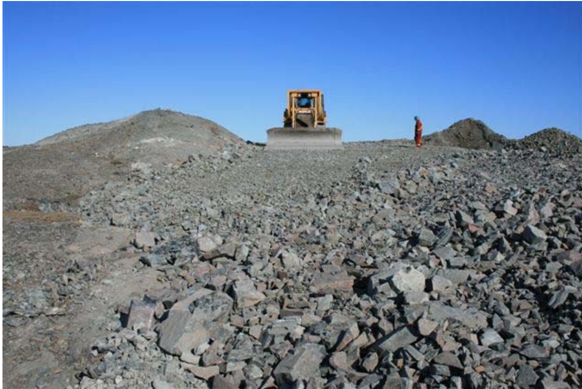
Gully on west side of landfill between landfill and rock outcrop filled to provide positive drainage
