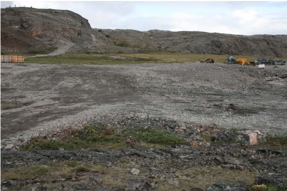
Photograph No. 12: Adit #1 at Roberts Bay post blasting and backfilling (7 August 2009)
