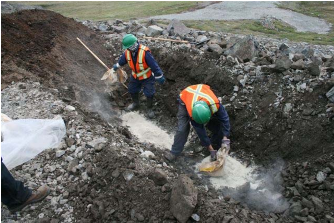
Spreading bentonite for bentonite seal.
