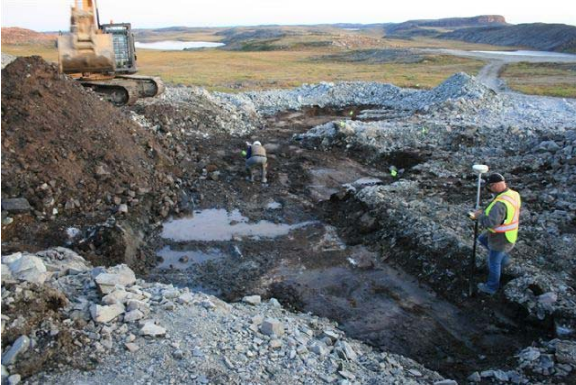
Photograph No. 53: Petroleum Hydrocarbon remediation at Garage Area of Roberts Bay
