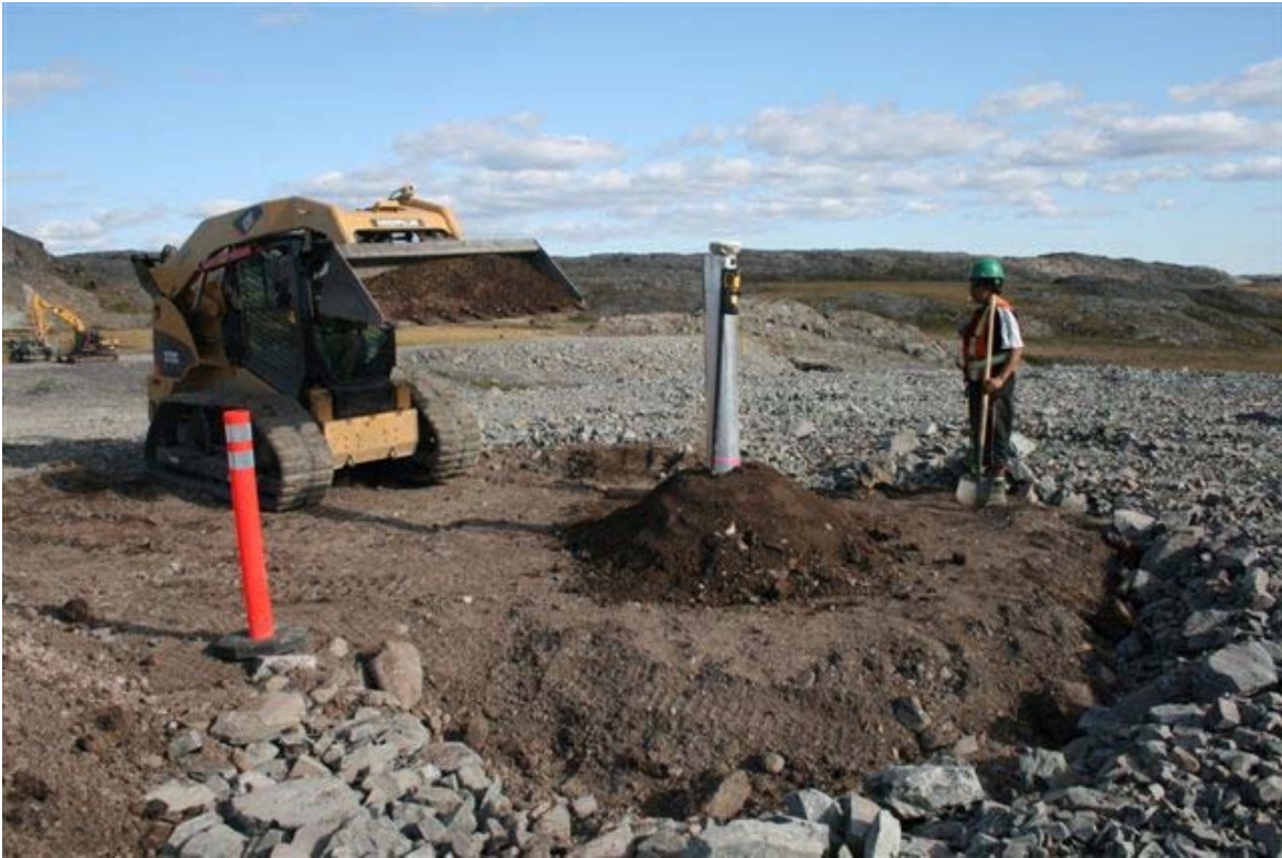
Thermistor A. Ground rod installed, grout placed. Type 2 protection placed. All three thermistors at this stage. Beads and sand in the pipe will be installed when final cap completed.
