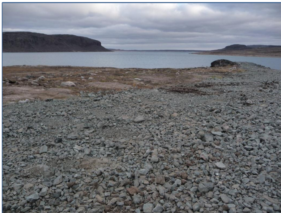
Wasterock Feathered Out to Match Topography from Northwest - After
