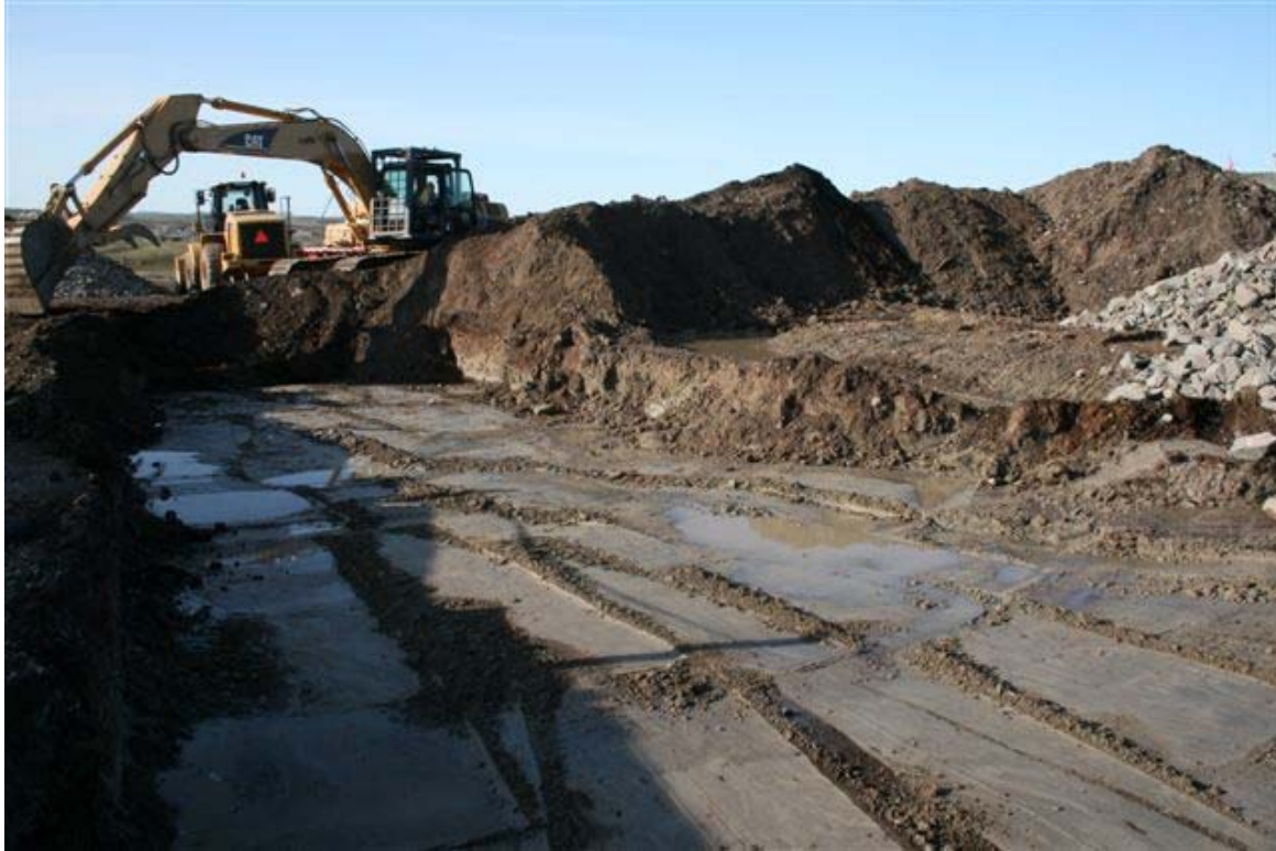
Excavation and stockpiling at borrow source 4
