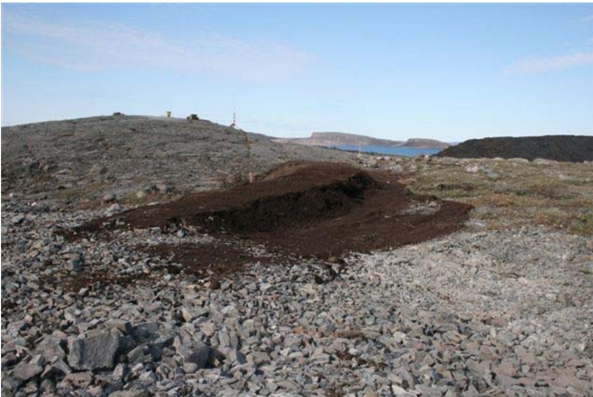
Berm at north west corner of landfill. Void to the south will be filled with type 1 material.
