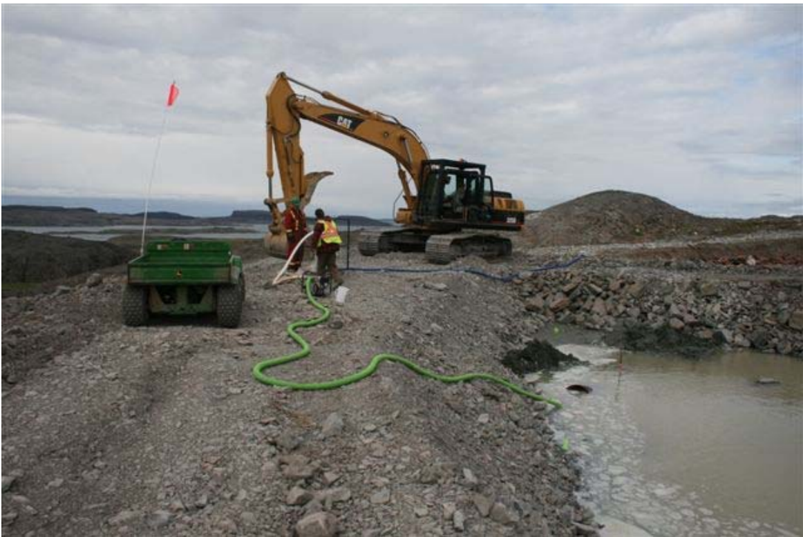
Photograph No. 64: Decanting water above tailings to dry side of SWMF
