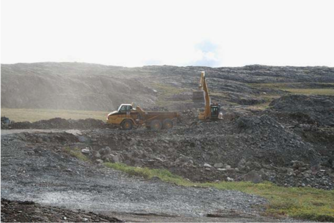
Hauling Type 1 material from blasted area south of adit 1. This source is nearly depleted.
