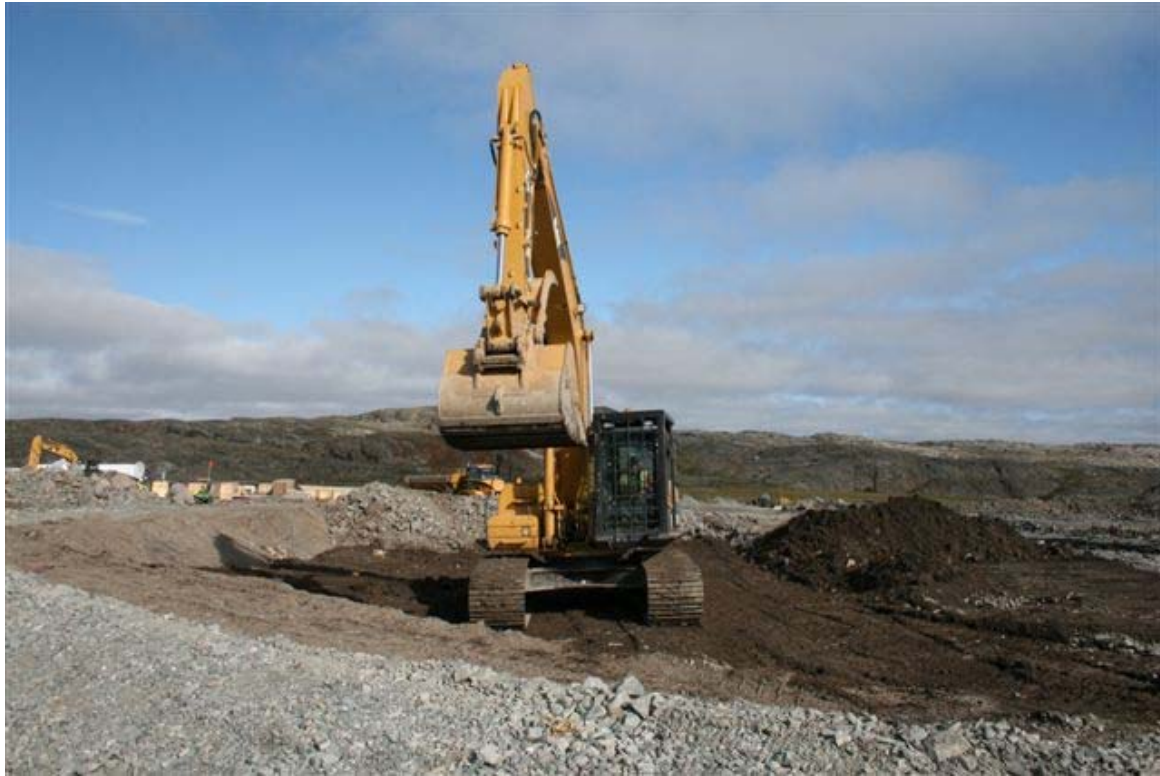
Compacting type 2 material over debris in the dry cell
