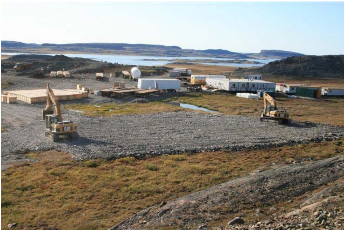
Borrow source backfilled. Excavators are compacting with their tracks
