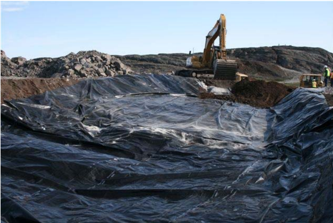
Photograph No. 62: Landfill (SWMF) during construction (placement of geotextile)
