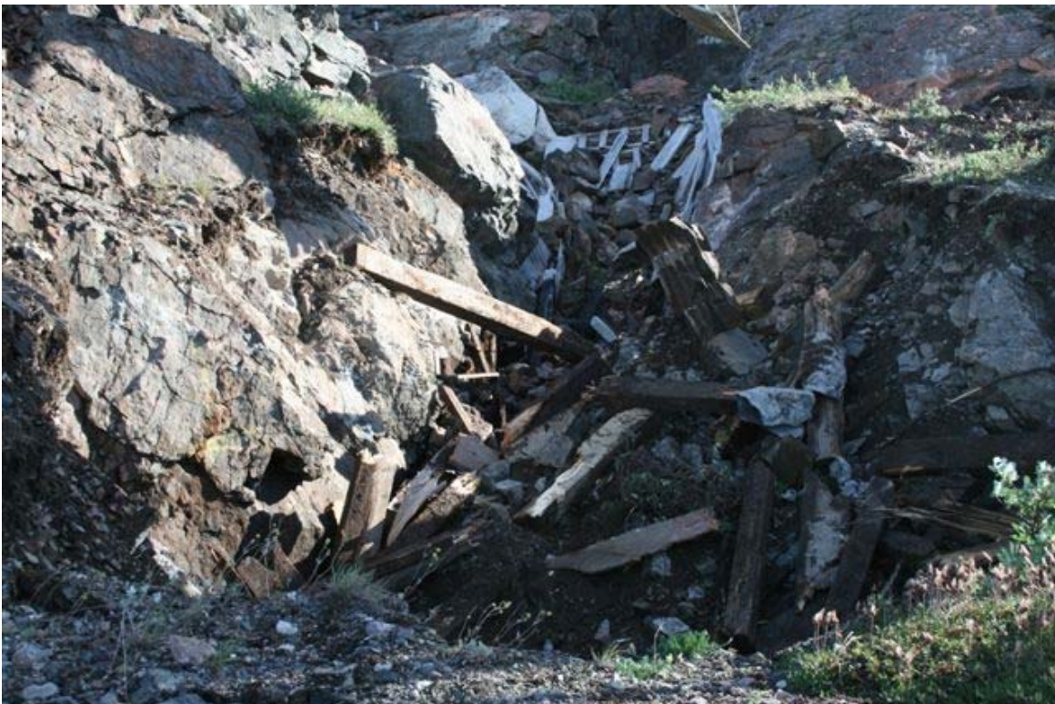
Adit #2 after shaft collapsed and before timber removed
