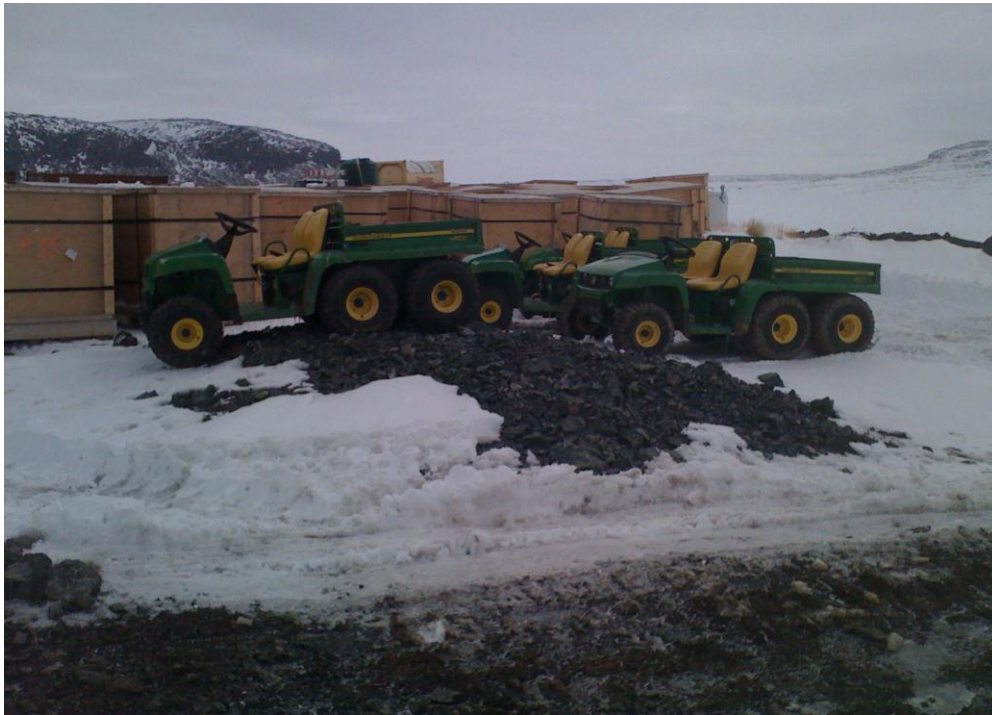
Photo 5: Stock pile of scrapped potentially contaminated soil, covered with 4" gravel.
