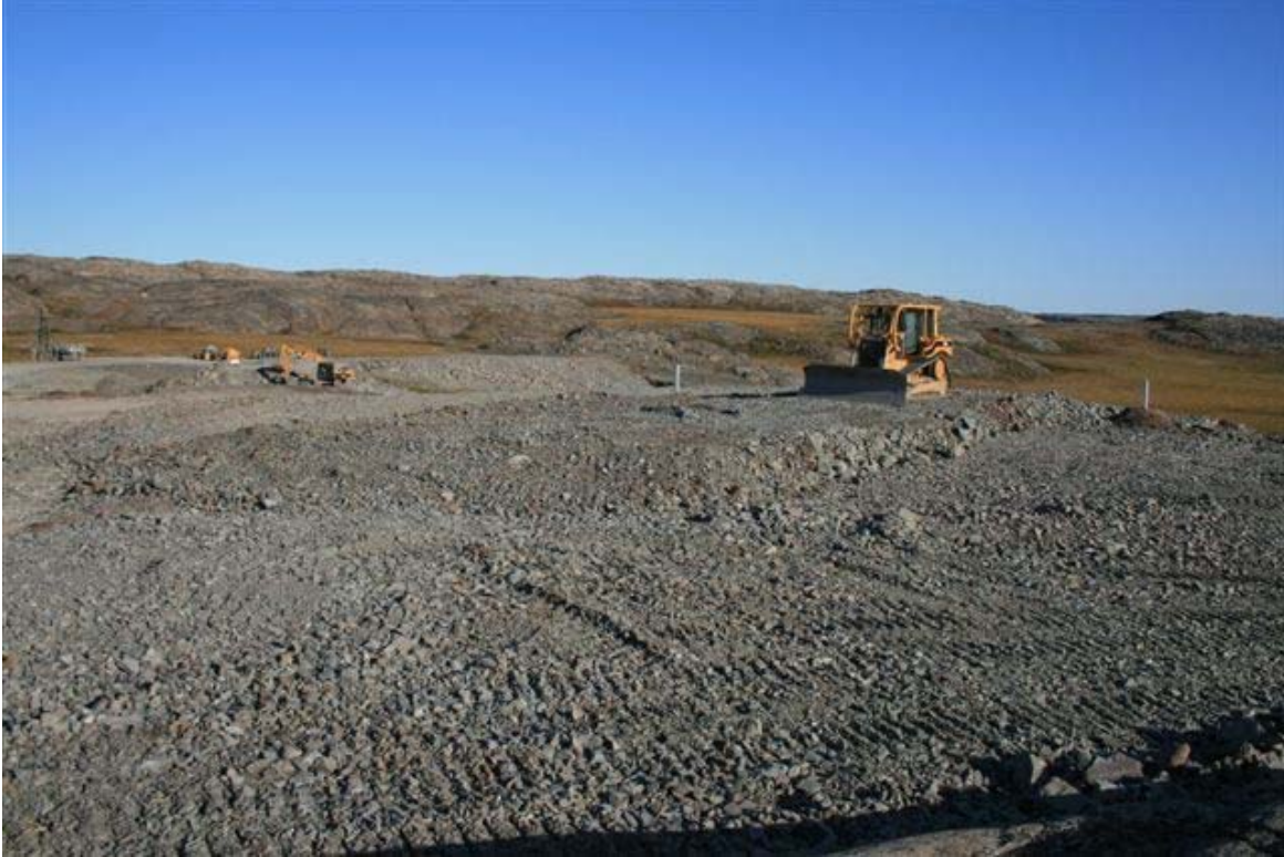
Start placement of final crown
