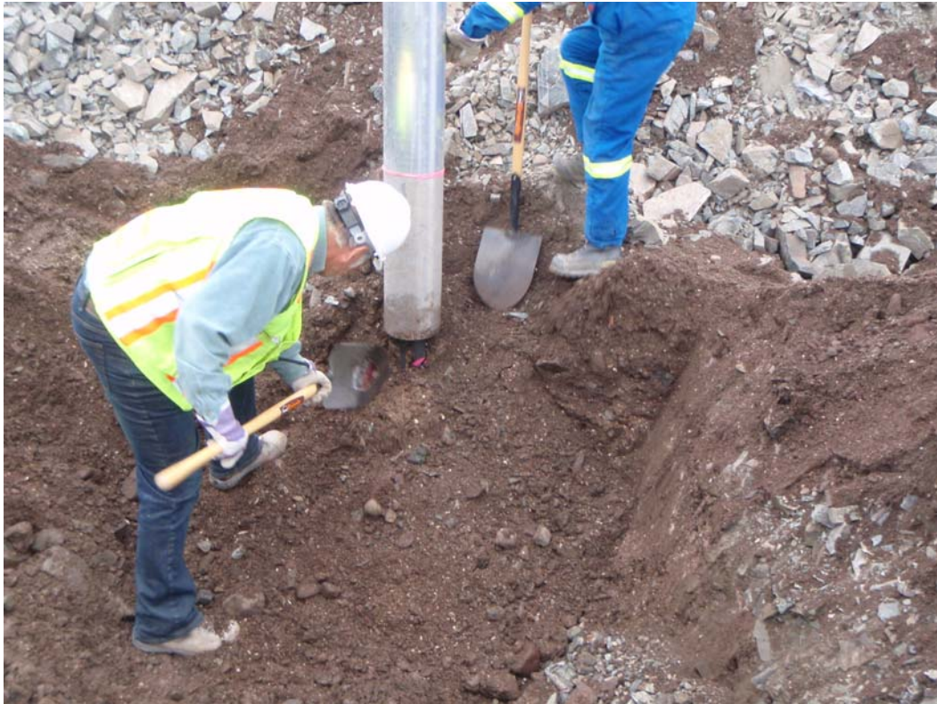
Excavation of Thermistor A housing.
