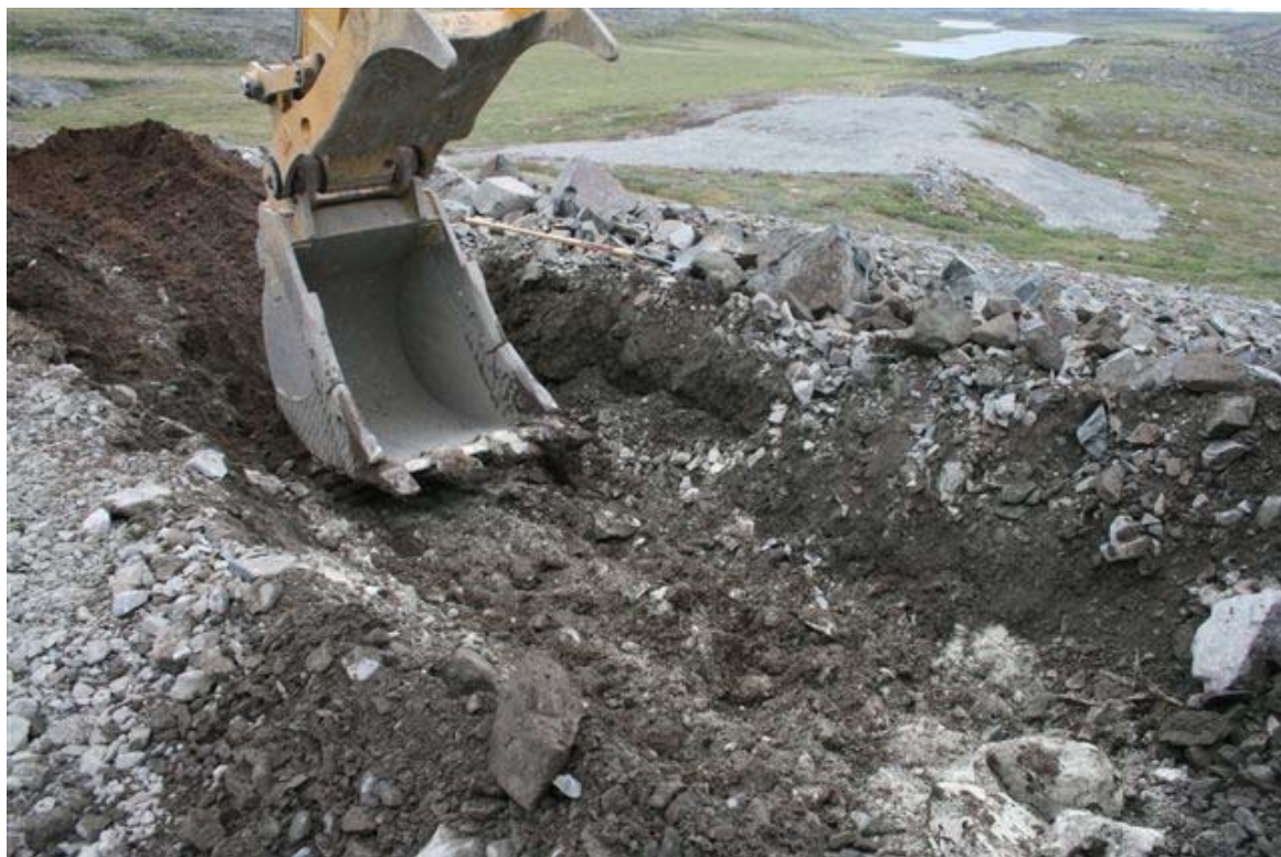
Mixing and compacting thin lifts of bentonite seal.
