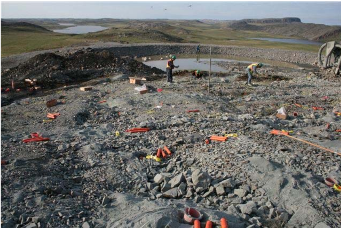
Workers installing dynamite
