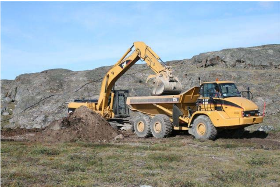
Excavating type 2 material from borrow source 4
