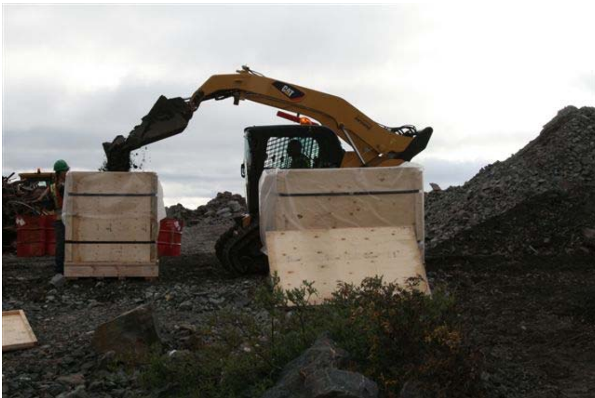
Contaminated soil loaded into boxes
