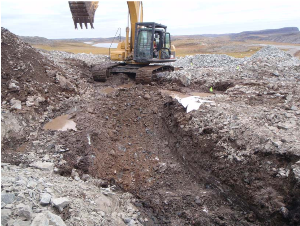
North end of Contaminant Zone Advanced to Bedrock.
