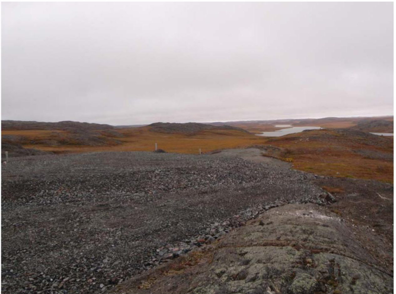
Photograph No. 71 Final Cover Placed with thermistors.
