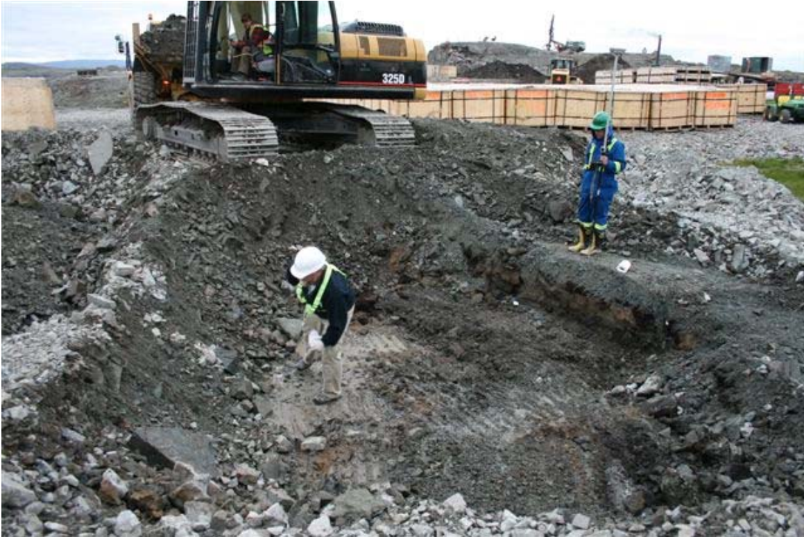
Photograph No. 49: Petroleum Hydrocarbon remediation at the POL Area of Roberts Bay
