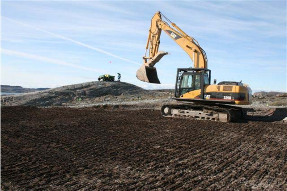
Photograph No. 69: Final Cover Placement Works
