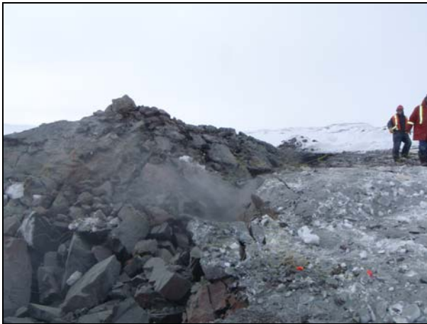
April 23, 2009 – IBMS: Collapsed Adit.
