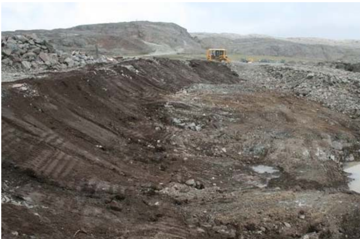
Slopes of dry cell being lined with Type 2 material to receive 20 mil liner.
