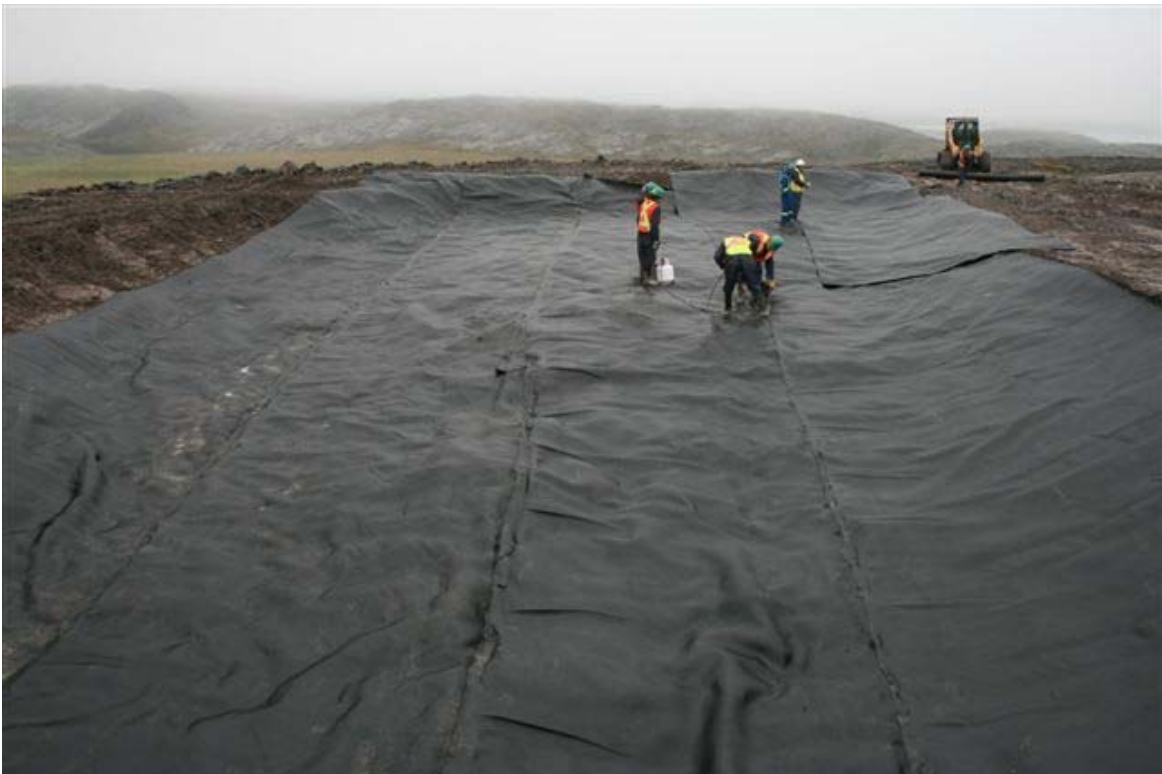
Photograph No. 66: Placement of liner inside SWMF during construction
