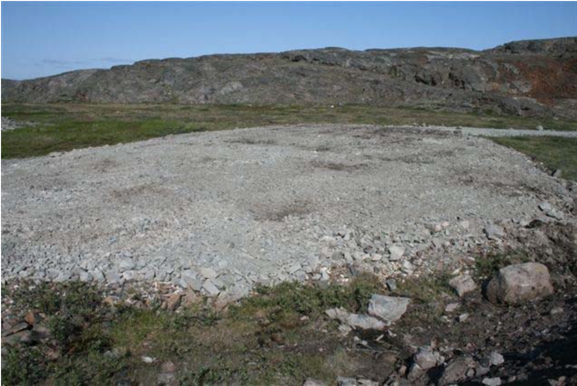
Pad constructed overlapping the fuel bladder area. Pad will be used to stage contaminated soil boxes.
