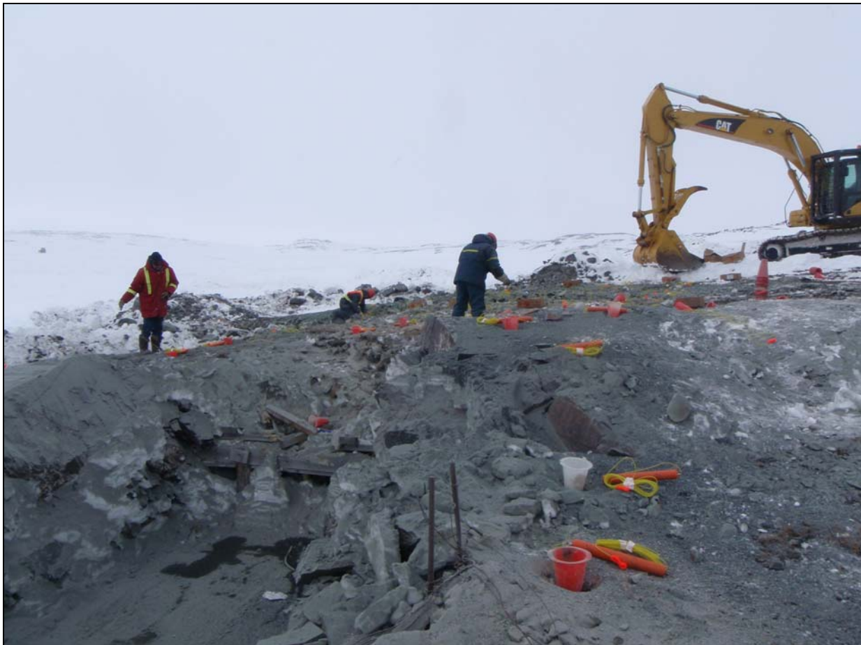
April 23, 2009 – IBMS: Drilling and Setting up Blast at Adit.
