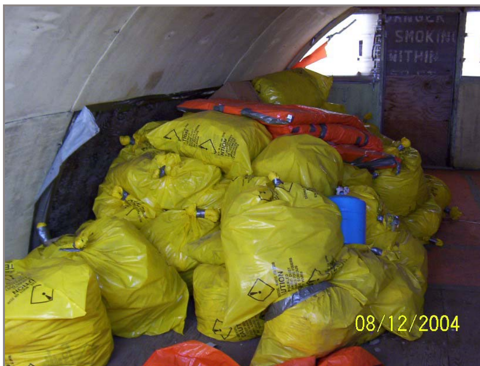
Photo 20 - Asbestos Containing Materials inside Quonset Building
