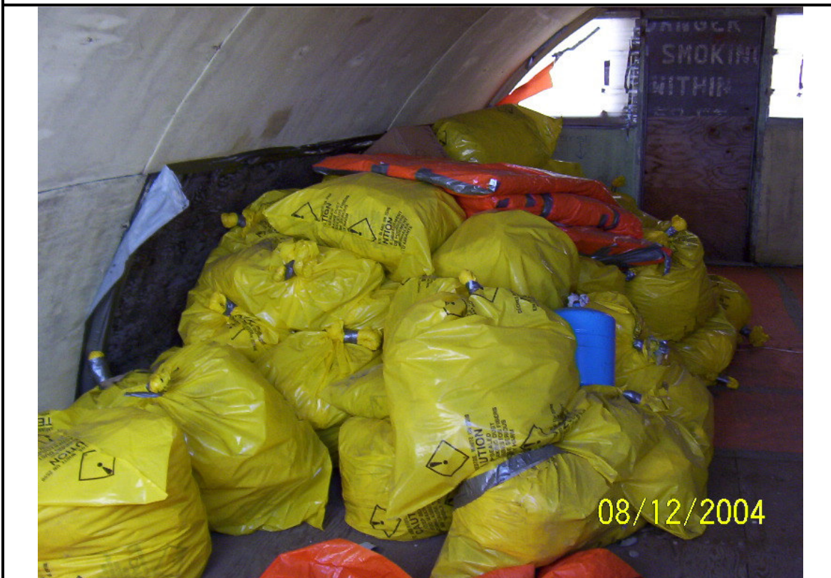
Photo 20: Asbestos containing materials inside Quonset building.
