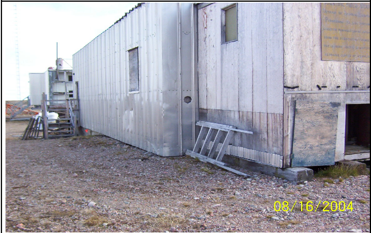
Photo 4: Warehouse view north east towards Module Station.
