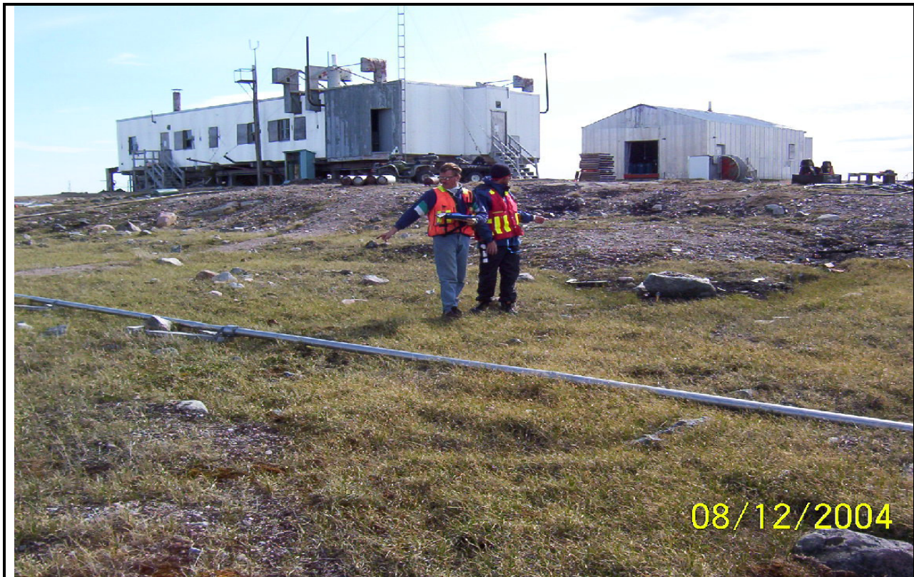
Photo 1: Module Station view south.
