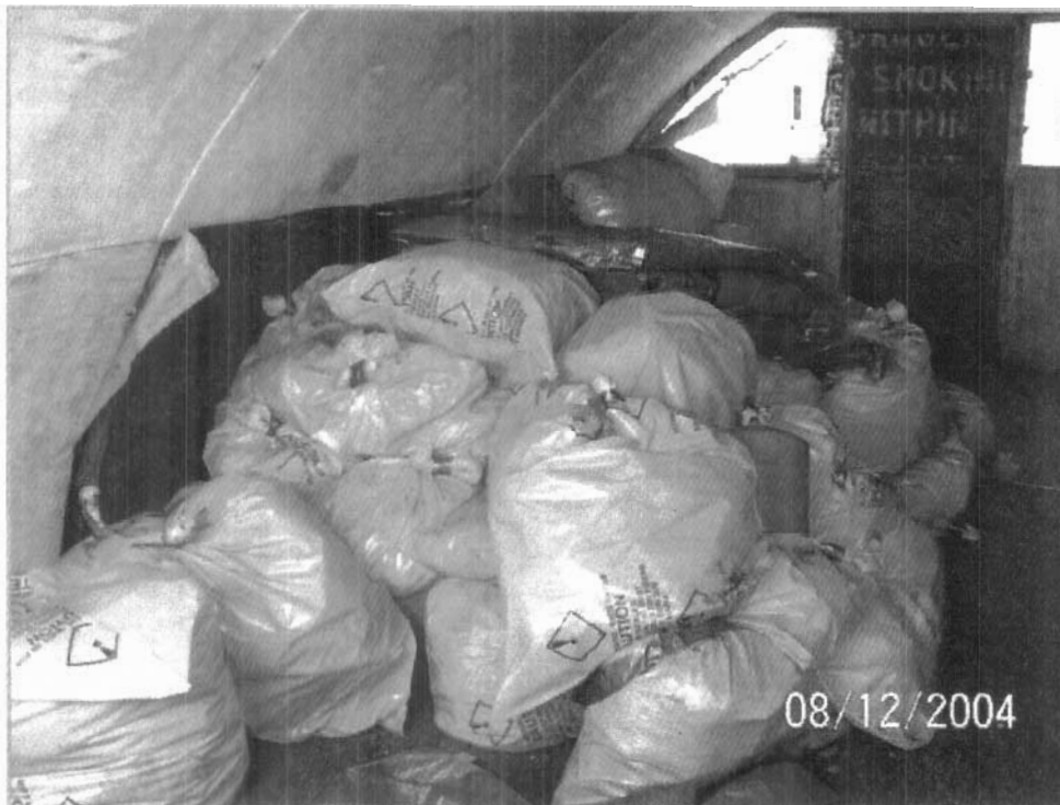
Photo 20 - Asbestos Containing Materials inside Quonset Building
