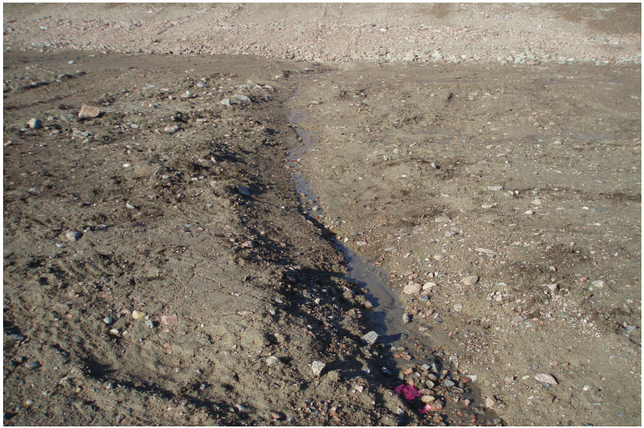
Photo 7: Picture 23 SSDF – Erosion Channel at the Toe of South Facing Slope (Figure A1)
