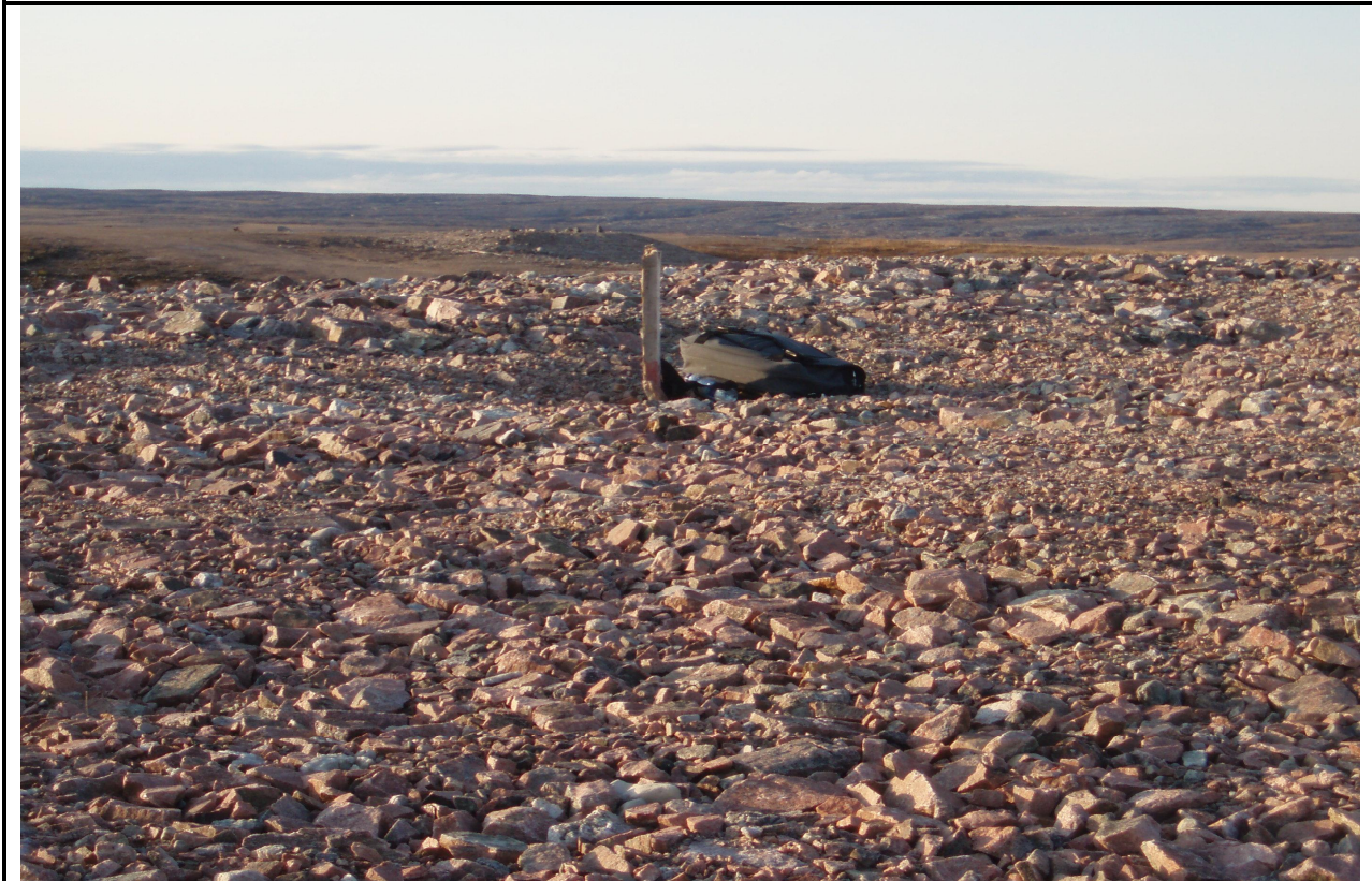
Photo 6: Picture 40 NHWLF – Settlement (4mx2m) on the Landfill Surface, (Figure A2)
