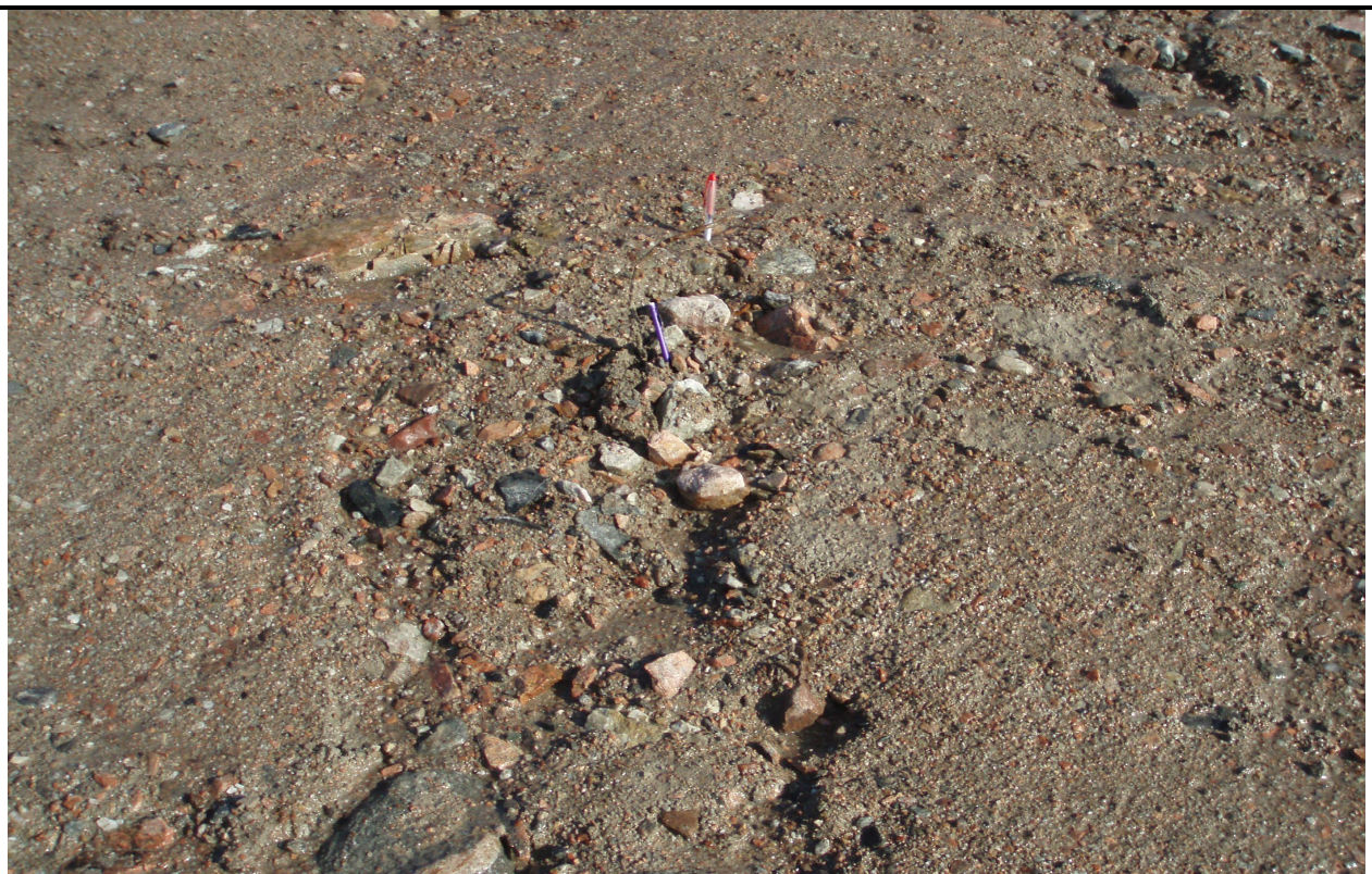
Photo 6: Picture 10 SSDF – Seepage/Erosion on West Facing Slope (Figure A1)
