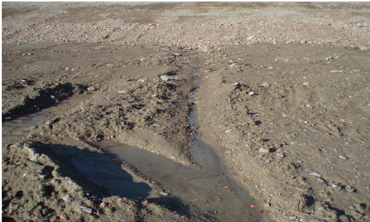
Photo 8: Picture 24a SSDF – Erosion Channel at the Toe of South Facing Slope (Figure A1)
