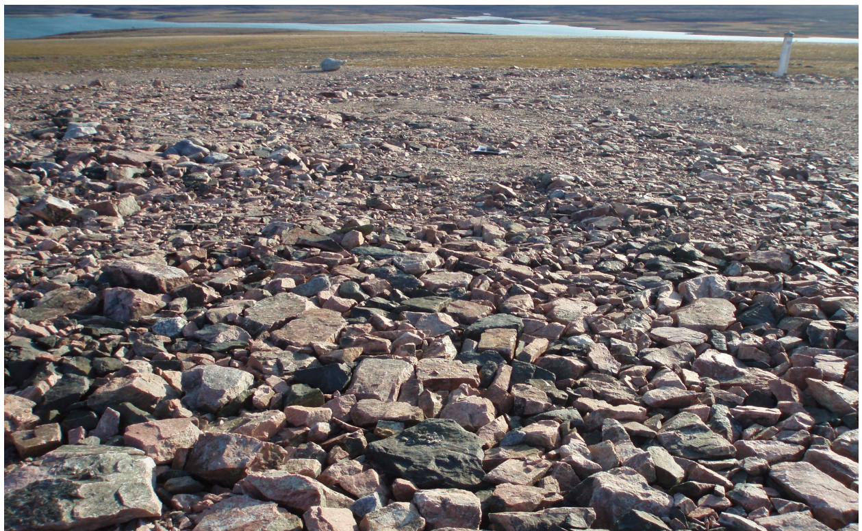
Photo 12: Picture 63 SSDF – Minor Settlement (15mx15mx0.10-0.15m) on Landfill Surface (Figure A1)
