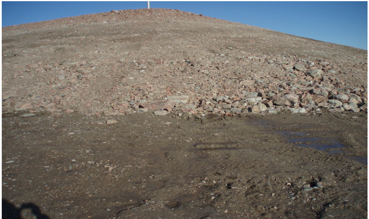
Photo 10: Picture 15 SSDF – Erosion Channel at the Toe of South Facing Slope (Figure A1)
