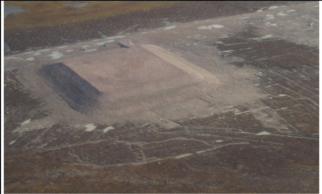
Photo 1: Picture 66 SSDF – Aerial View of the Landfill; Seepage on Sideslopes, Ponding Near the Landfill and Erosion Channels Near the South Facing Slope
