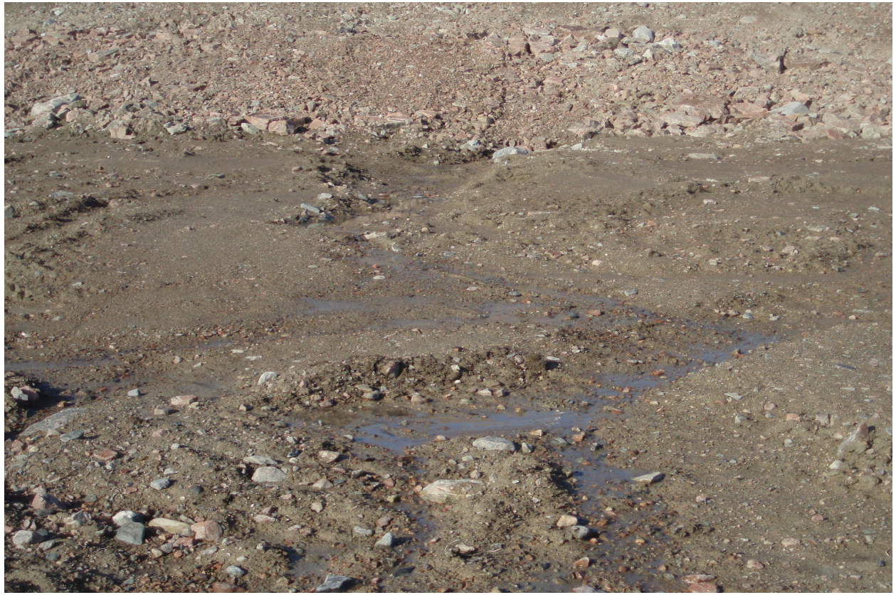
Photo 9: Picture 24b SSDF – Erosion Channel at the Toe of South Facing Slope (Figure A1)
