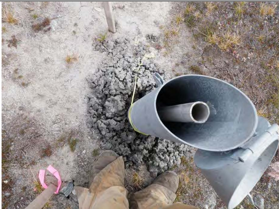
Photo 24. MW06-02 near the NHL with signs of a deteriorating bentonite surface seal (picture # P8250298).
