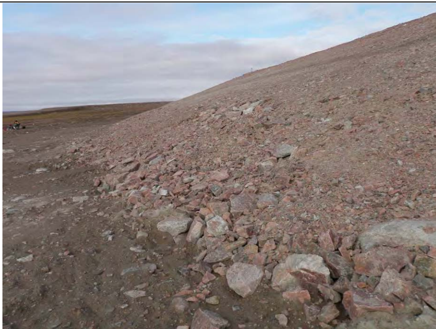
Photo 12. Exposed riprap on southern side slope of the SSDF. Direction photo taken: W (picture # P8250171).
