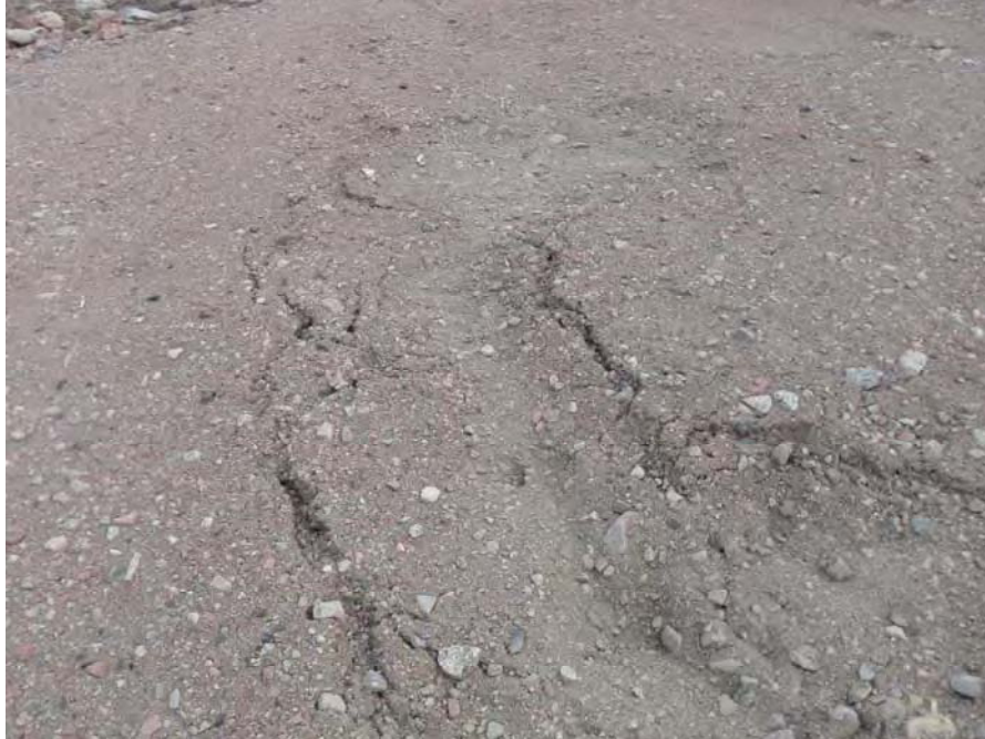
Photo 23. Close-up of depression, approximately 5 m long, to the western side of the southern corner of the NHL (picture # P8250302). Refer to Figure A-1, Appendix A, for exact location.
