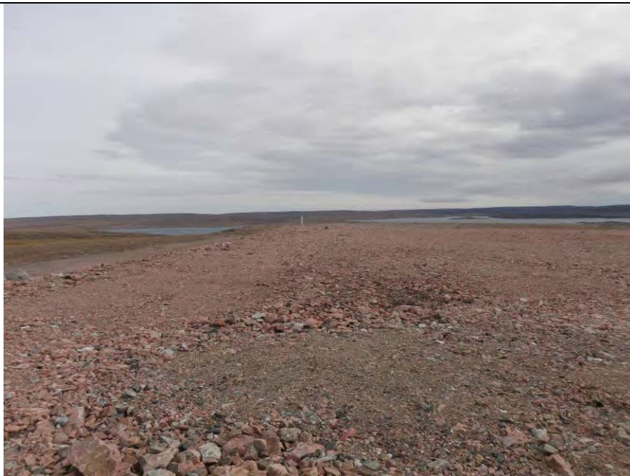
Photo 14. Minor erosion of fines and very slight depression on the top of the SSDF; picture viewpoint number 56 (Figure A-1, Appendix A). Direction photo taken: SE (picture # P8240119).
