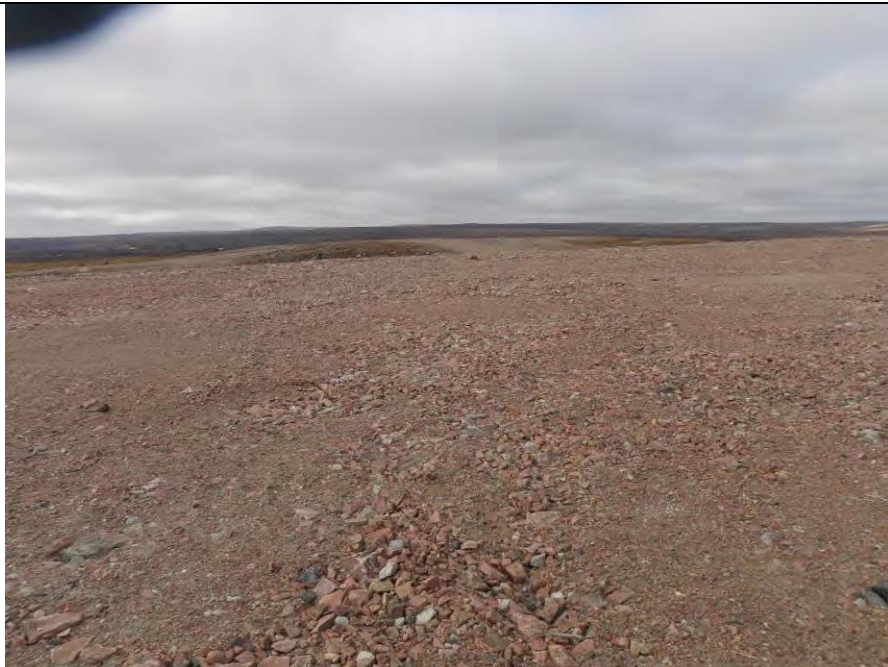
Photo 22. Top of NHWL showing minor erosion of fines revealing gravel and cobbles; picture viewpoint number 39 (Figure A-1, Appendix A). Direction photo taken: NW (picture # P8250274).
