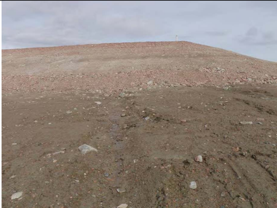
Photo 7. Rivulet (erosion channel) on south side of SSDF; picture viewpoint number 24a (Figure A-1, Appendix A). Direction photo taken: N (picture # P8240086).
