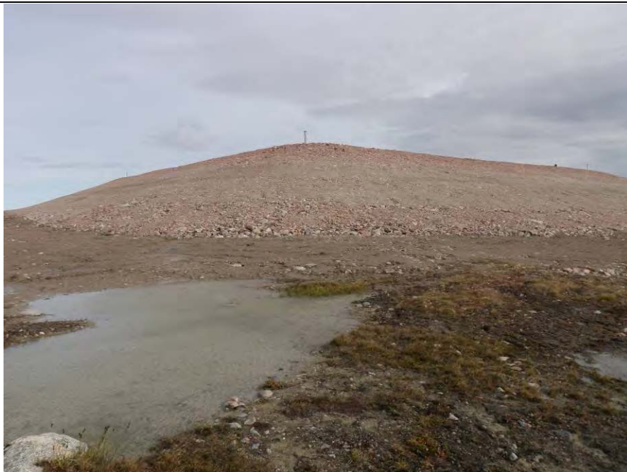
Photo 10. Ponding at the SW corner of the SSDF. A small rivulet (erosion channel) is also seen coming from the SSDF. Picture viewpoint number 15 (Figure A-1,Appendix A). Direction photo taken: NE (picture # P8240073).
