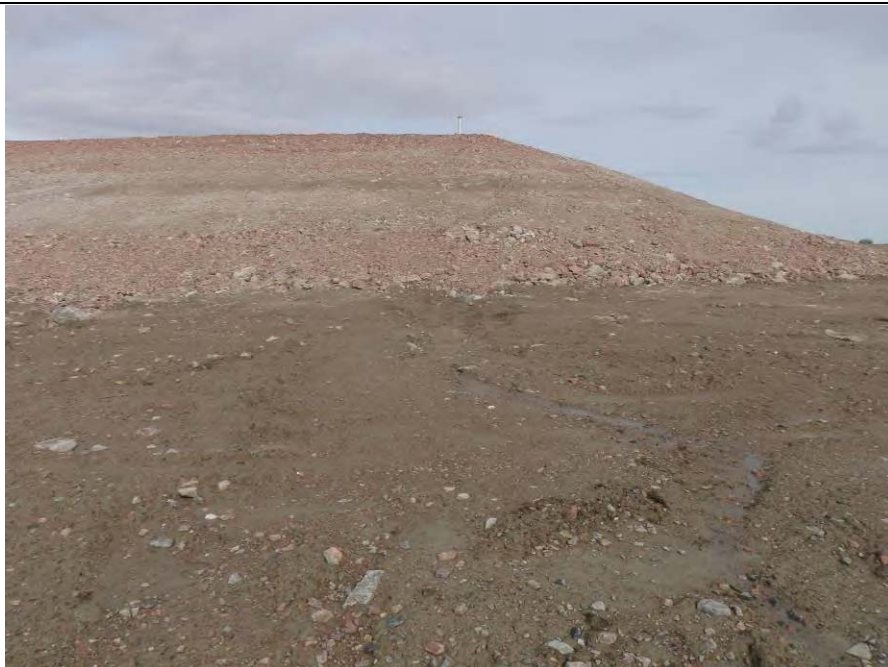
Photo 8. Rivulet (erosion channel) on south side of SSDF; picture viewpoint number 24b (Figure A-1, Appendix A). Direction photo taken: N (picture # P8240087).
