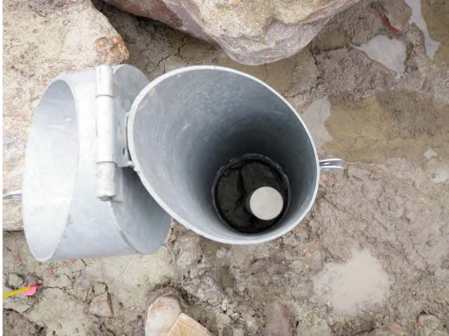
Photo 15. MW0604 on the north side of the SSDF showing bentonite upwelling and slight cracking. Ponding is also evident (picture # P8250155).
