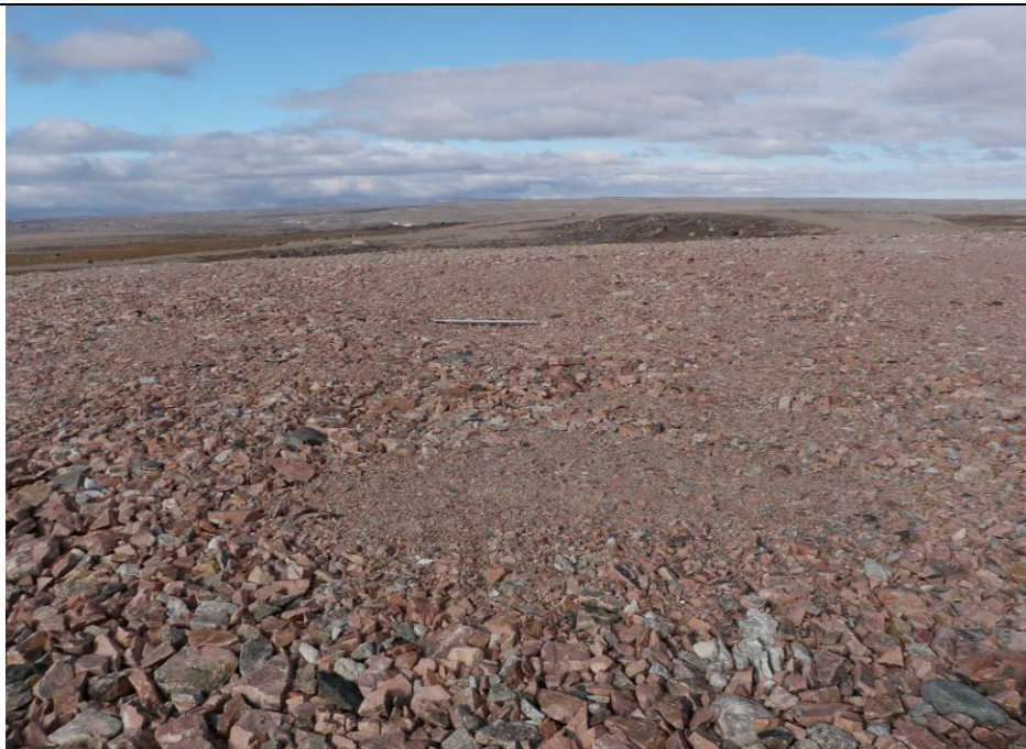
Photo 14. Top of NHWL showing minor depression and erosion of fines revealing gravel and cobbles; picture viewpoint number 35 (Figure A-2, Appendix A). Direction photo taken: NW (picture # P9080503).
