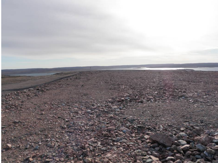
Photo 5. Minor erosion of fines and slight depression on the top of the SSDF; picture viewpoint number 56 (Figure A-1, Appendix A). No significant change since previous inspection. Direction photo taken: SE (picture # P9090677).
