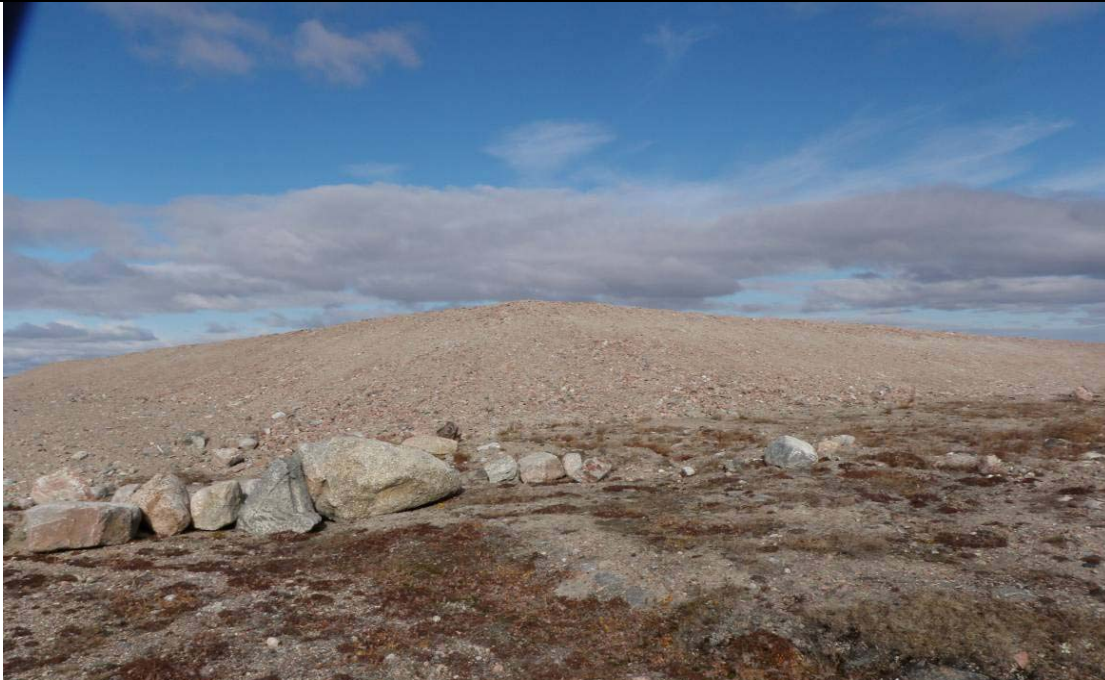
Photo 13. The south-eastern and south-western sides of the Non-Hazardous Waste Landfill (NHWL) shown from picture viewpoint number 23 (Figure A-2, Appendix A). Typical of all sides of the landfill, the NHWL shows little sign of erosion, seepage or settlement. Direction photo taken: N ( picture # P9080513).
