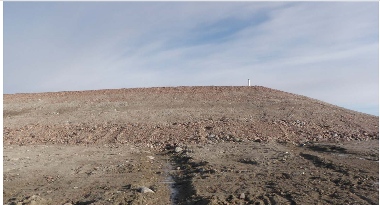
Photo 2. Rivulet (erosion channel) on south side of SSDF; picture viewpoint number 24a (Figure A-1, Appendix A). Direction photo taken: N (picture # P9090571).
