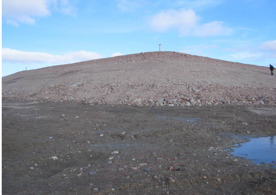
Photo 3. Picture viewpoint number 15 (Figure A-1, Appendix A) of the SW corner of the SSDF. Seepage points A, B and C can be seen on the far left; ponded surface appears in the lower right; and exposed riprap can be seen along the southern edge of the landfill toe. Direction photo taken: NE (picture # IMG_2499).
