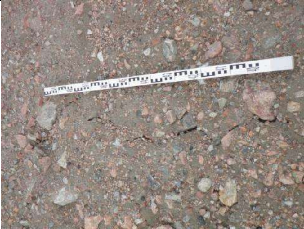
Cracking on west slope of SSDF. Viewpoint 59 (Figure A-2; Appendix A). Photograph reference P8270156 (CD-ROM). Direction photo taken: E
