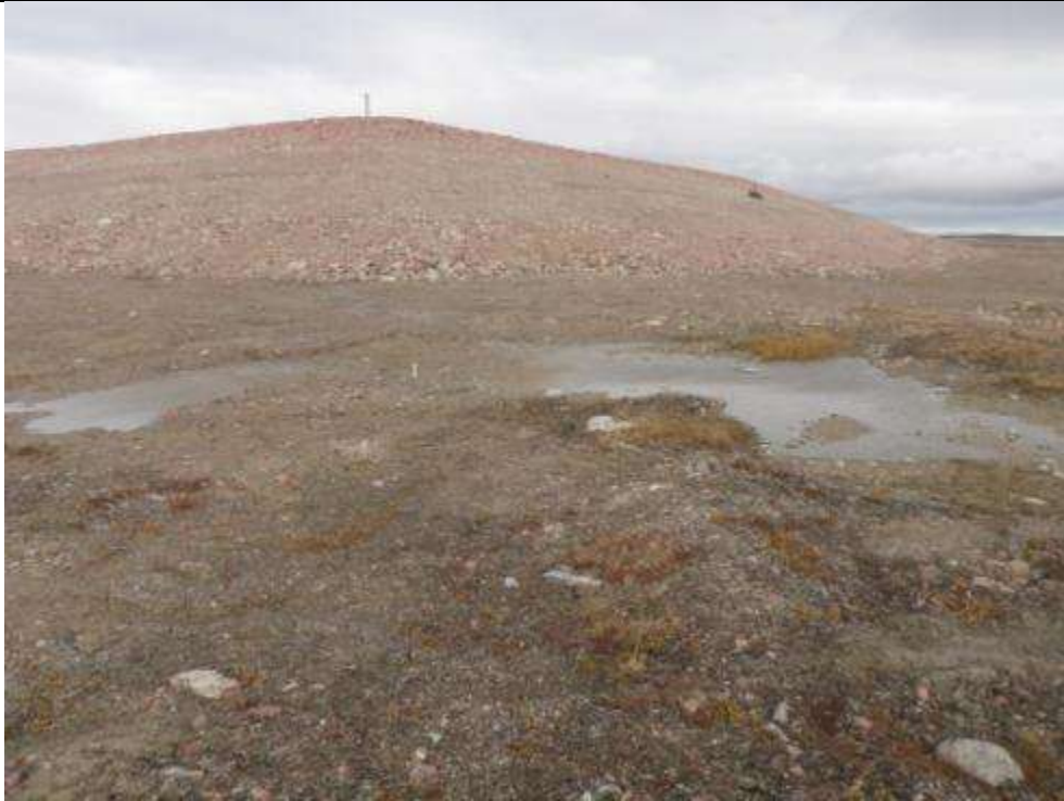
Ponding from active seepage at the southwest corner. Viewpoint 68 (Figure A-2; Appendix A). Photograph reference P8270165 (CD-ROM). Direction photo taken: NE
