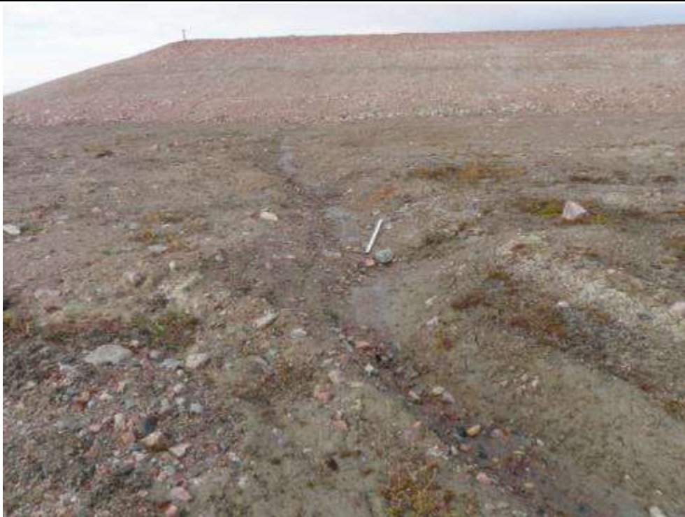
Active erosion from active seepage along the south toe of the SSDF. Viewpoint 74 (Figure A-2; Appendix A). Photograph reference P8270171 (CD-ROM). Direction photo taken: N
