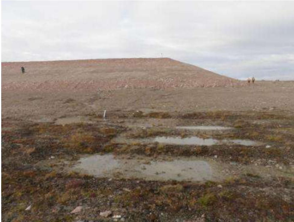
Ponded water from the active seep near the southeast corner of the SSDF. Viewpoint 78 (Figure A-2; Appendix A). Photograph reference P8270175 (CD-ROM). Direction photo taken: SE
