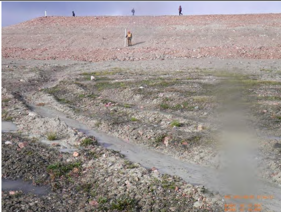
Active erosion from active seepage along the south toe of the SSDF. Viewpoint 80 (Figure A-2; Appendix A). Photograph reference RIMG0080 (CD-ROM). Direction photo taken: N
