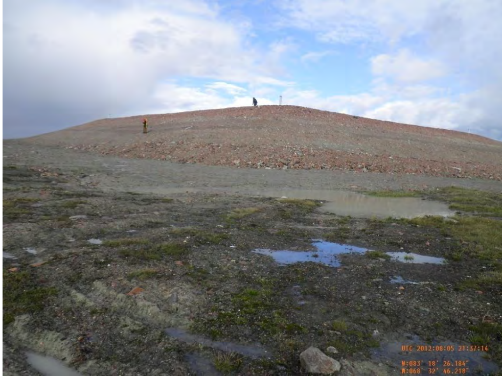
Ponding from active seepage at the southwest corner. Viewpoint 73 (Figure A-2; Appendix A). Photograph reference RIMG0073 (CD-ROM). Direction photo taken: NE
