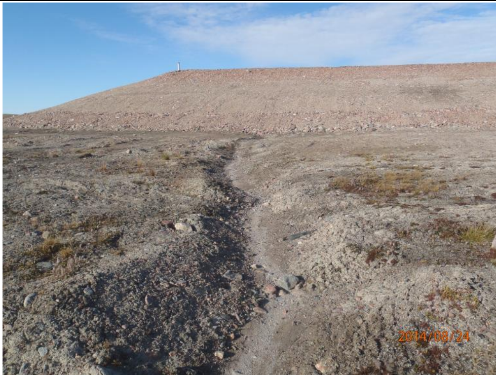
Active erosion from active seepage along the south toe of the SSDF. Dry in 2014. Viewpoint 80 (Figure A-2; Appendix A). Photograph reference P8240080 (CD-ROM). Direction photo taken: N
