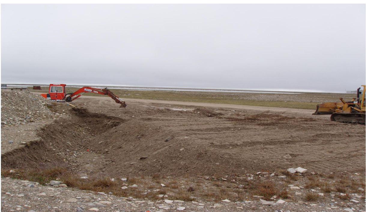
Photo 2: Backfilling contaminated soil area #9.
