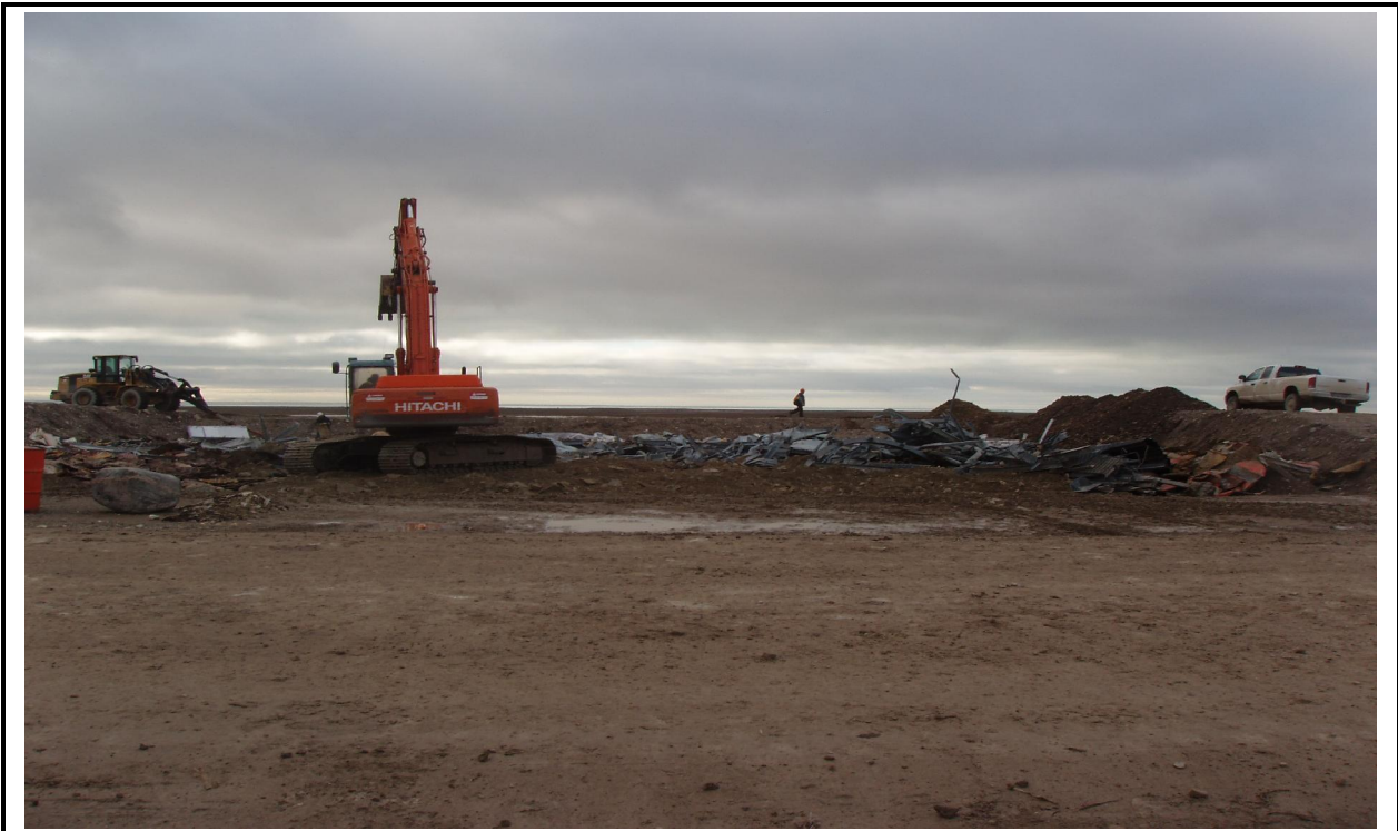
Photo 5: Placement of cover layer on Non-Hazardous Waste Landfill
