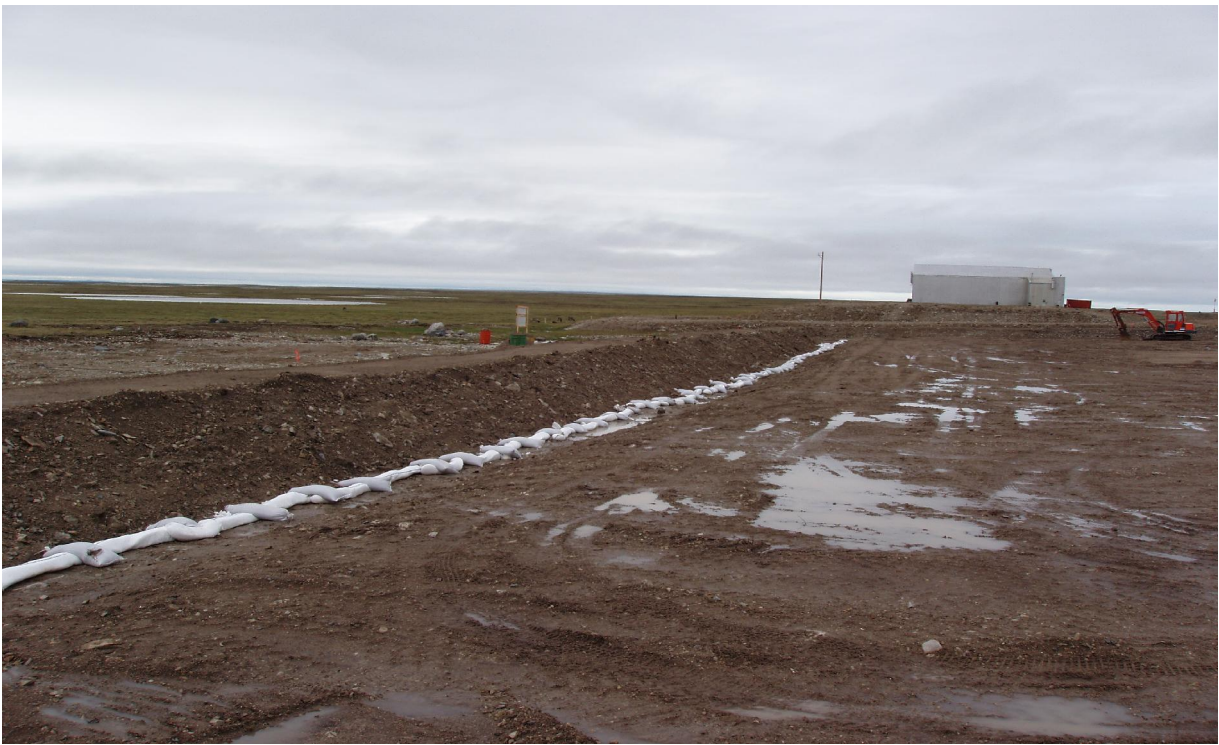
Photo 7: Oil sorbent booms at the landfarm
