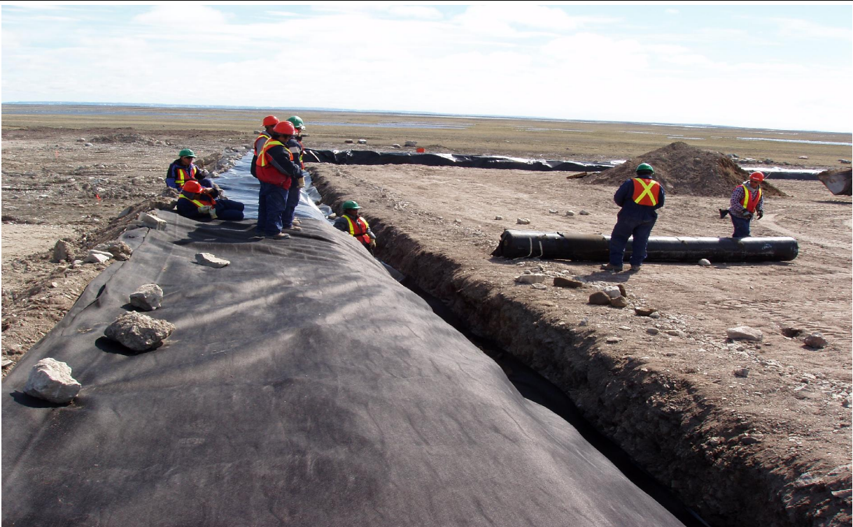
Photo 8: Placement of geotextiles at landfarm
