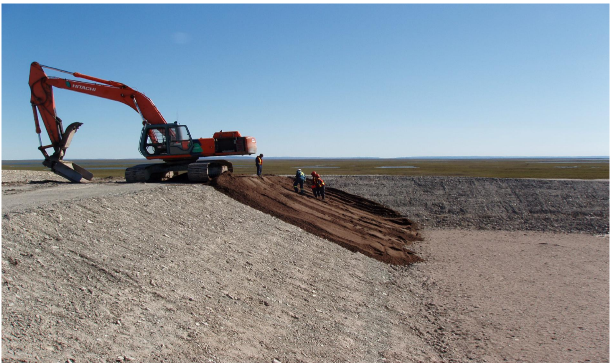
Photo 4: Placement of sand layer on Tier II Soil Disposal Facility berms
