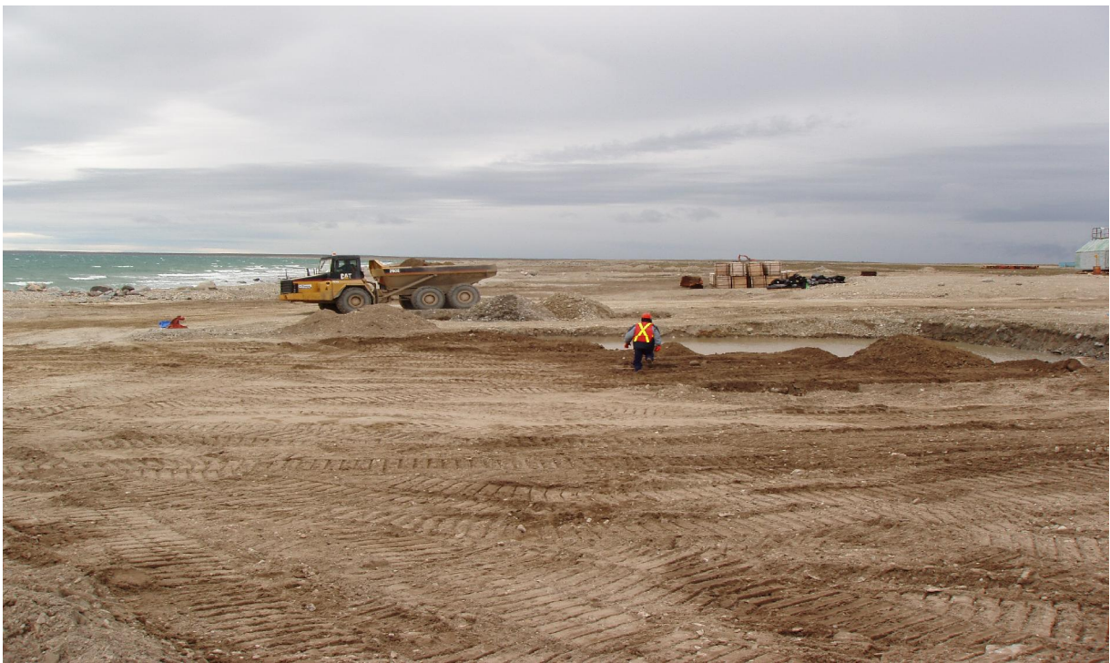
Photo 1: Backfilling Beach POL excavation.
