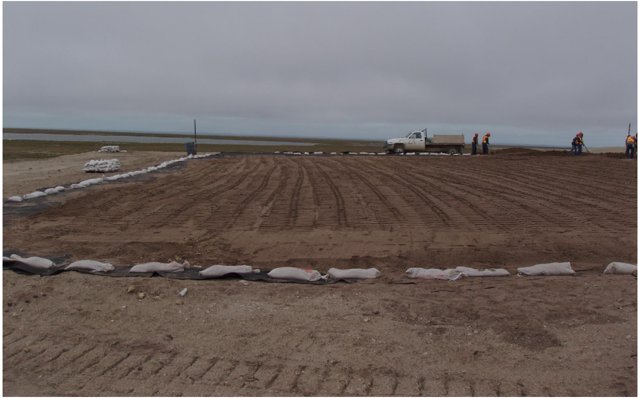
Photo 7: Tier II Landfill, compacted Tier II contaminated soil (prior to addition of liner and cap material)
