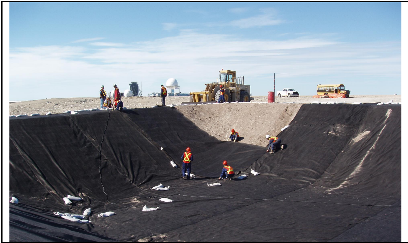
Photo 5: Tier II Landfill base liner installation
