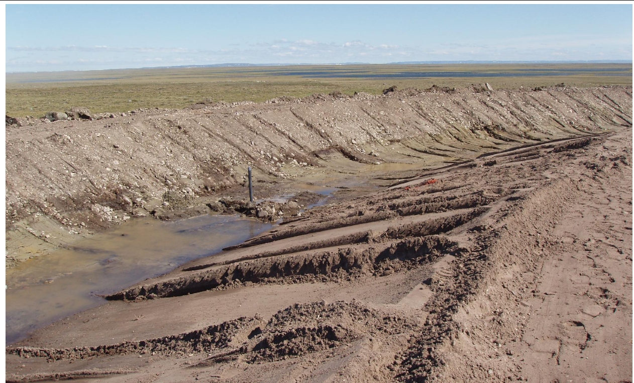
Photo 8: USAF Landfill liner key trench
