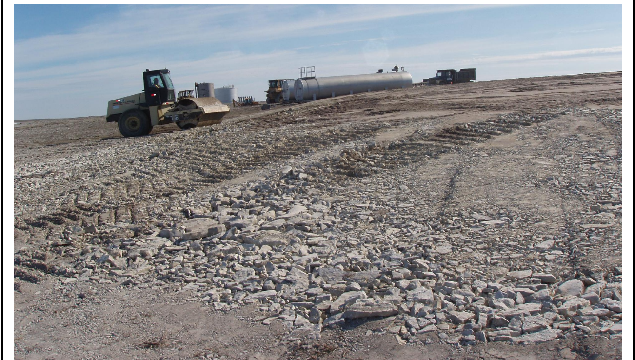
Photo 14: Beach Landfill (Regrade #1) compacting cover material
