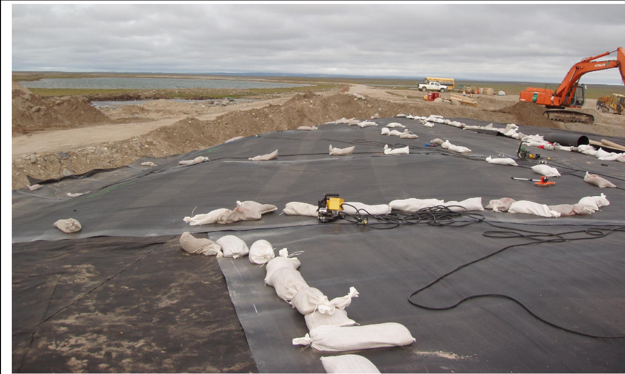
Photo 10: USAF Landfill, installing geomembrane, geotextile then type 5 granular fill over landfill
