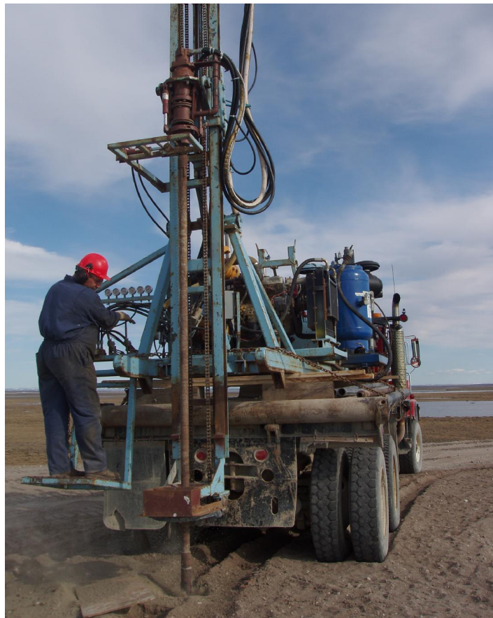
Photo 12: Drilling Thermistor borehole on Tier II Landfill
