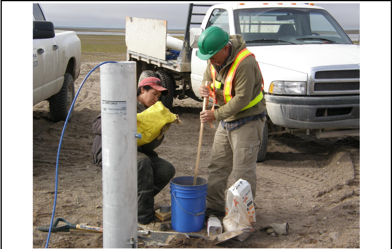
Photo 13: Installing Thermistor
