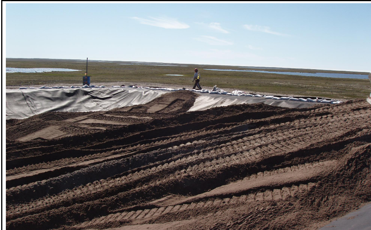
Photo 6: Tier II Landfill, adding base Type 5 granular fill
