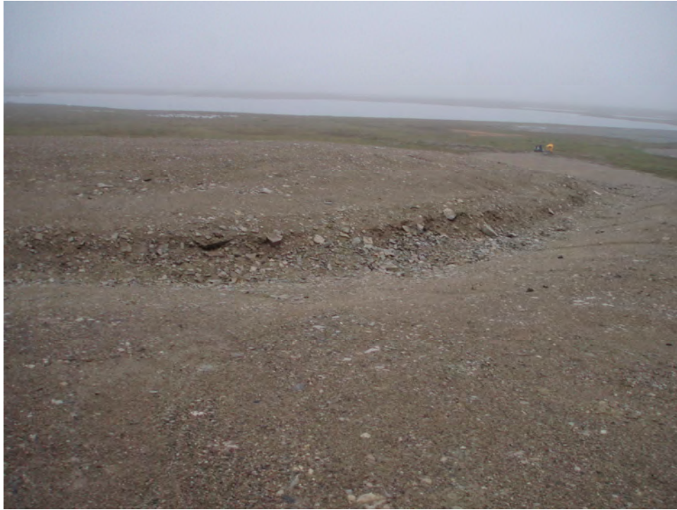
Photograph 3. Erosion in Side Ditch, Fines Washed Away, Course Material Exposed (20m) ↑
