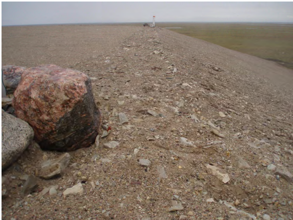
Photograph 6. Landfill Surface - Minor Erosion at Crest of Slope, Looking East (Fines Washed Away) ↑
