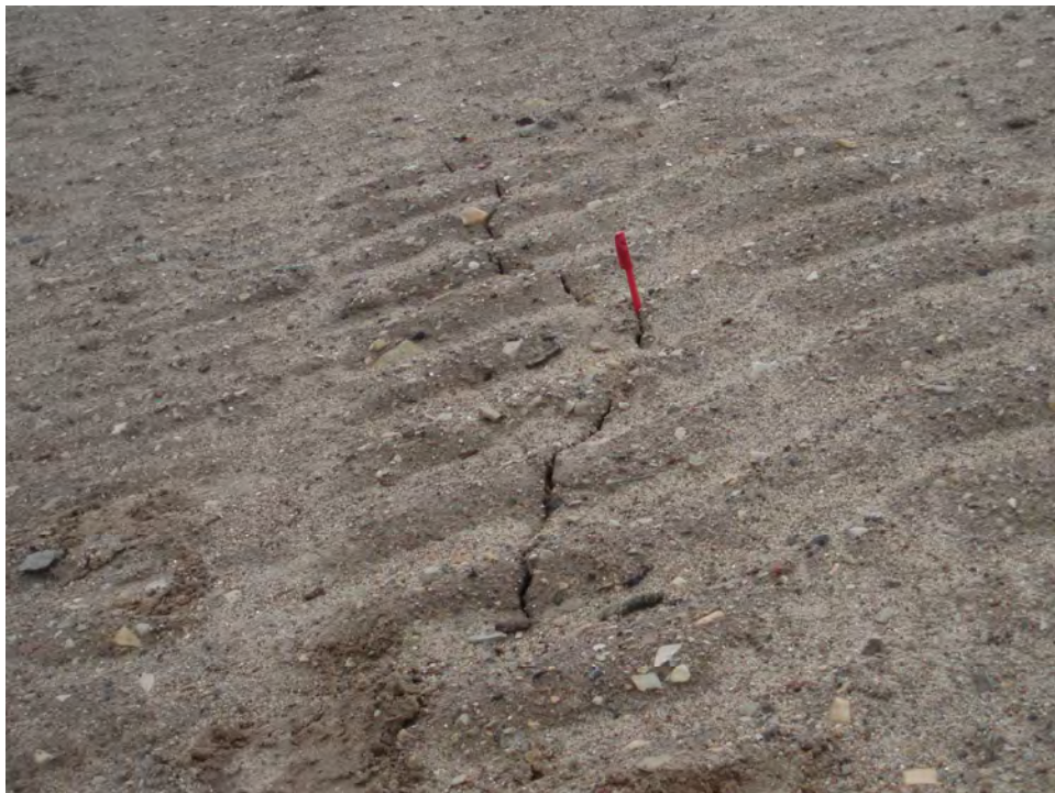
Photograph 4. South Facing Slope - Minor Crack (3-5 mm Wide) on Slope Running E-W ↑
